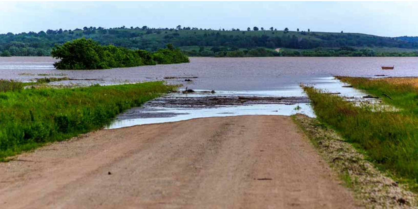
Flooded roadway and bridge in Marshall County, KS, 2015.
