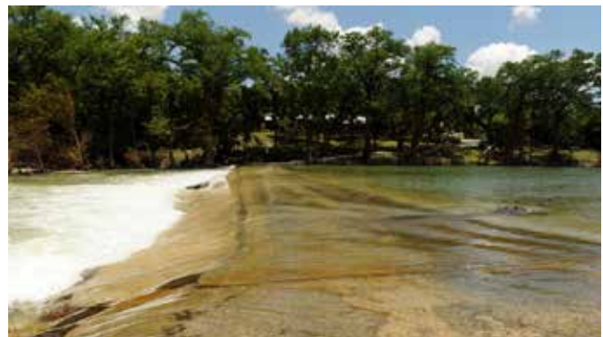
Fast-moving floodwaters in Texas, undated.
