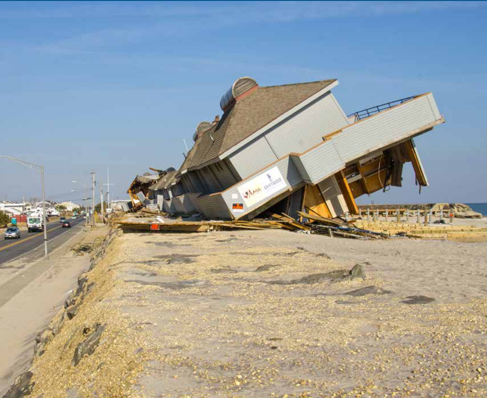
Flood damage in Sea Bright, NJ, 2012.
