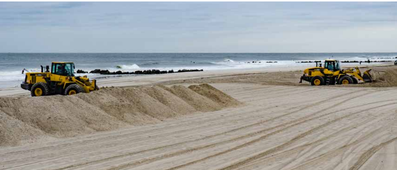
Sand berm construction in Long Beach, NY, 2015.
