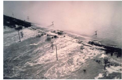
Figure 3-31: Failed Levee
