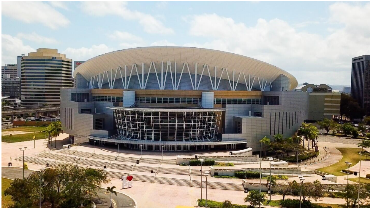
(Mar. 19, 2021) – In the case of the iconic José Miguel Agrelot Coliseum, known as the “Choliseo”, the allocation of approximately $4.9 million is earmarked for permanent works. Photo FEMA/Eliezer Hernández
