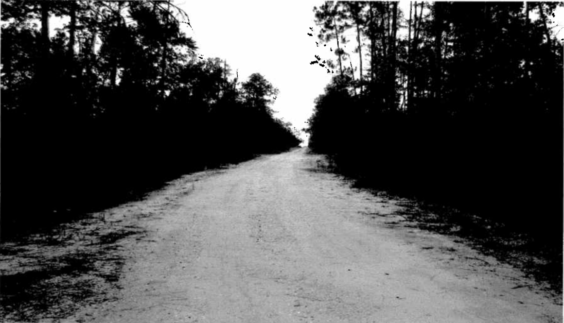
View of existing road facing north. The waterline will be buried under this road parallel to existing utility line. This photo is on the south side of Interstate 10.
