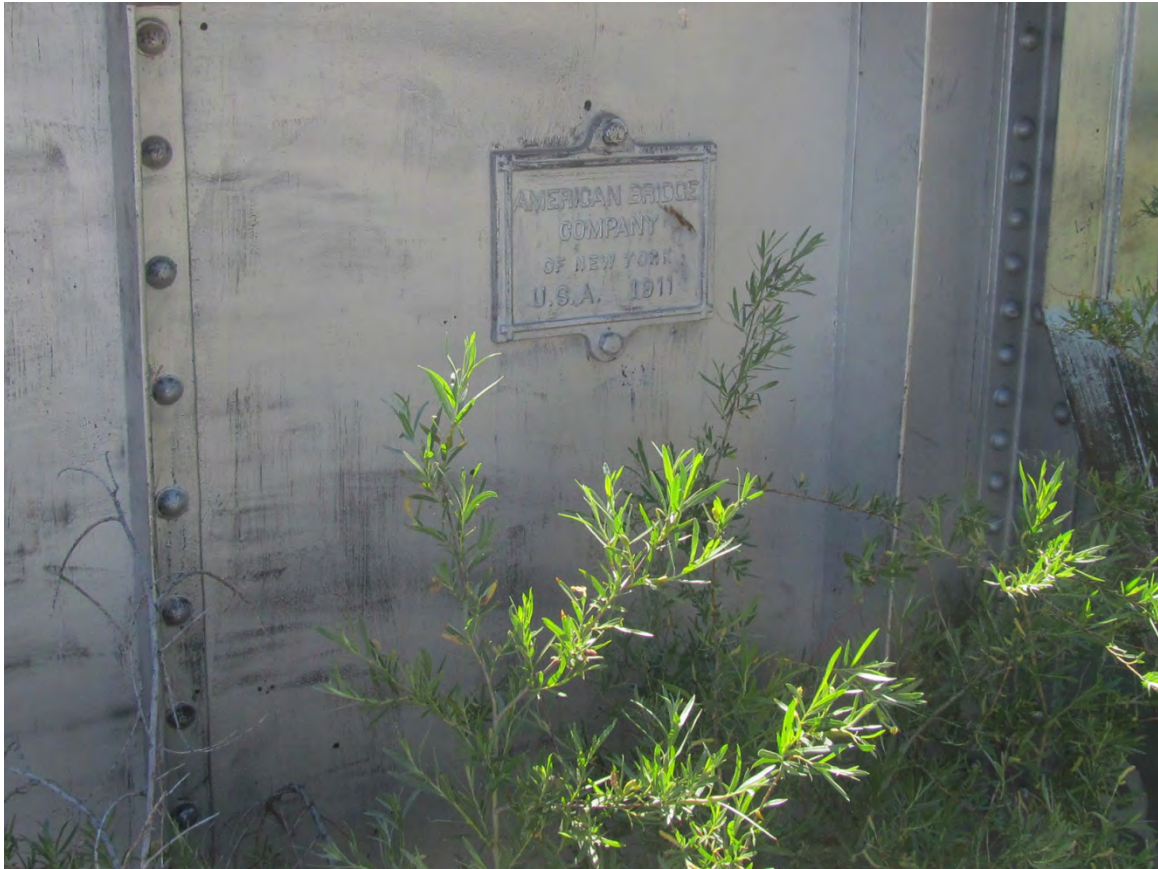
Figure 30. Plaque of American Bridge Company, 1911.
