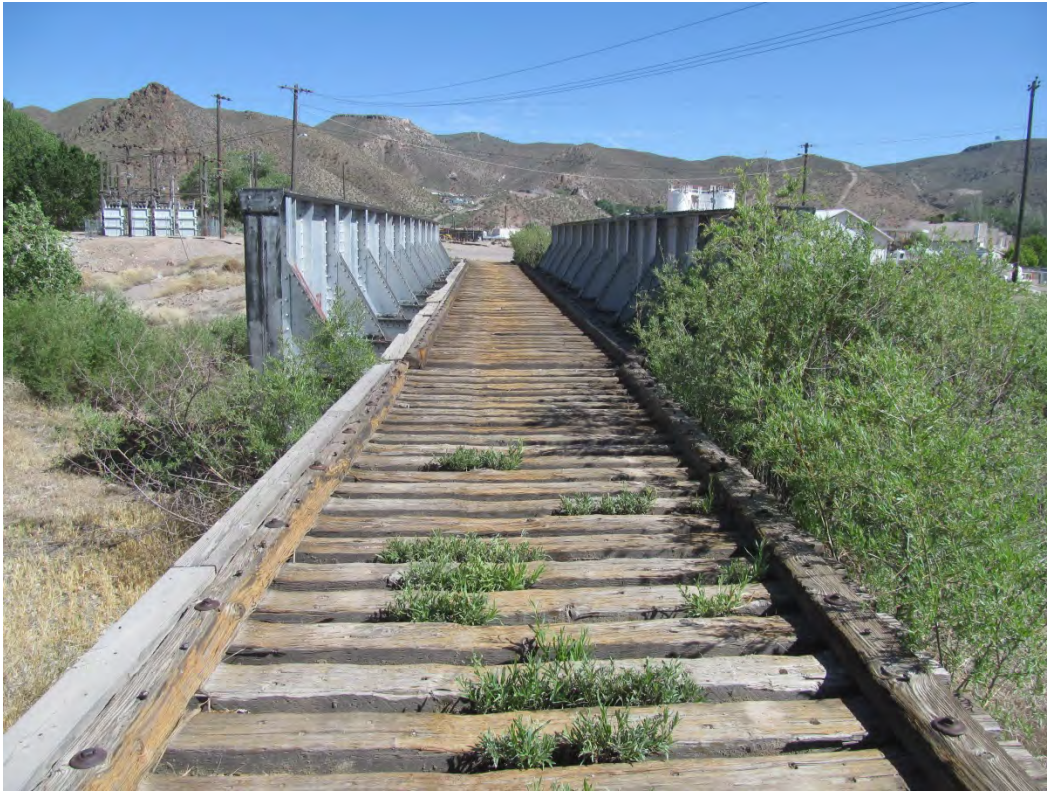
Figure 26. West end of C&P bridge, view southeast.
