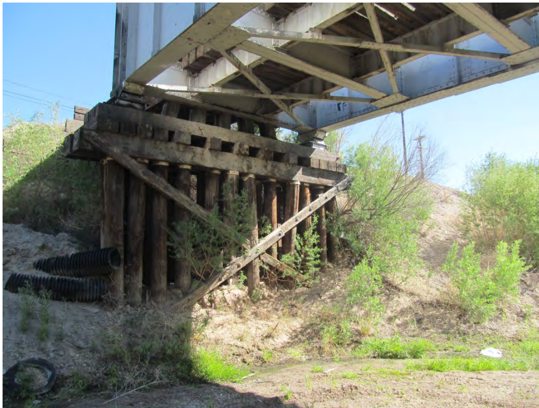
Figure 29. Substructure of west end C&P bridge, view southeast.
