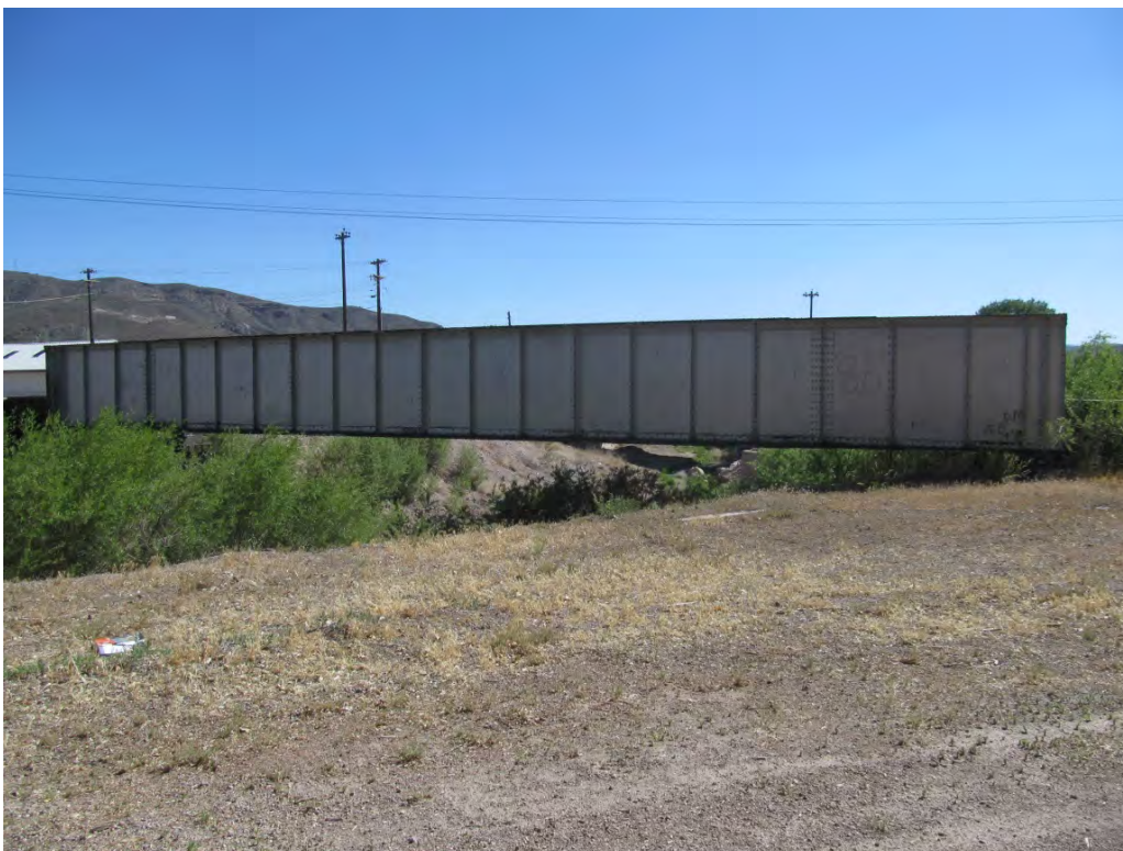
Figure 25. Full length of C&P bridge, view southwest.
