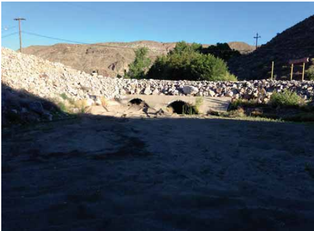
Clover Creek – looking west toward existing culverts/project site.
