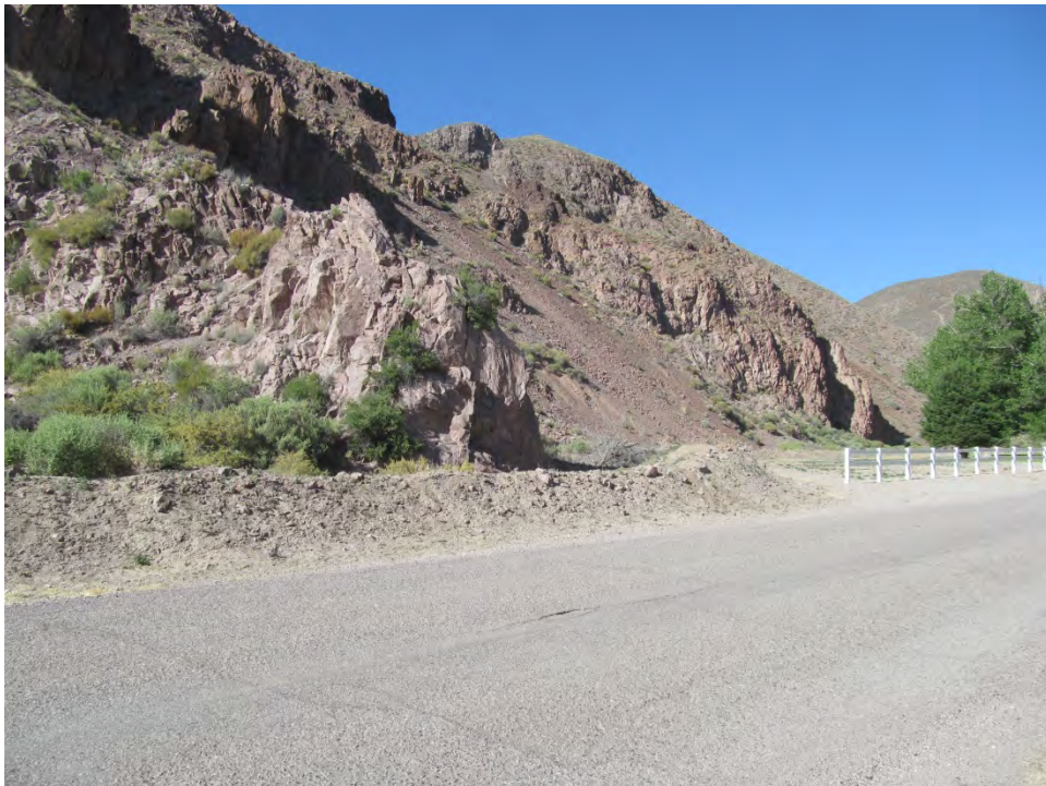
26LN6830. Site overview. Facing 27° Camera 1, Rotation 1, Image 32.tif. Taken at 719846mE/4166571mN (NAD 83).
