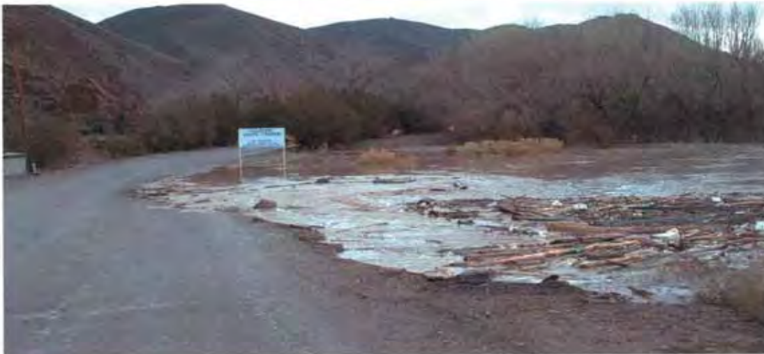
Caliente Youth Center Access Road - 1/10/05
