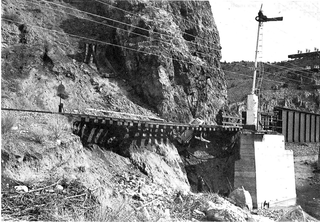
Figure 31. Historic photo of C&P bridge, washed out by 1938 flood (from Myrick 1963).
