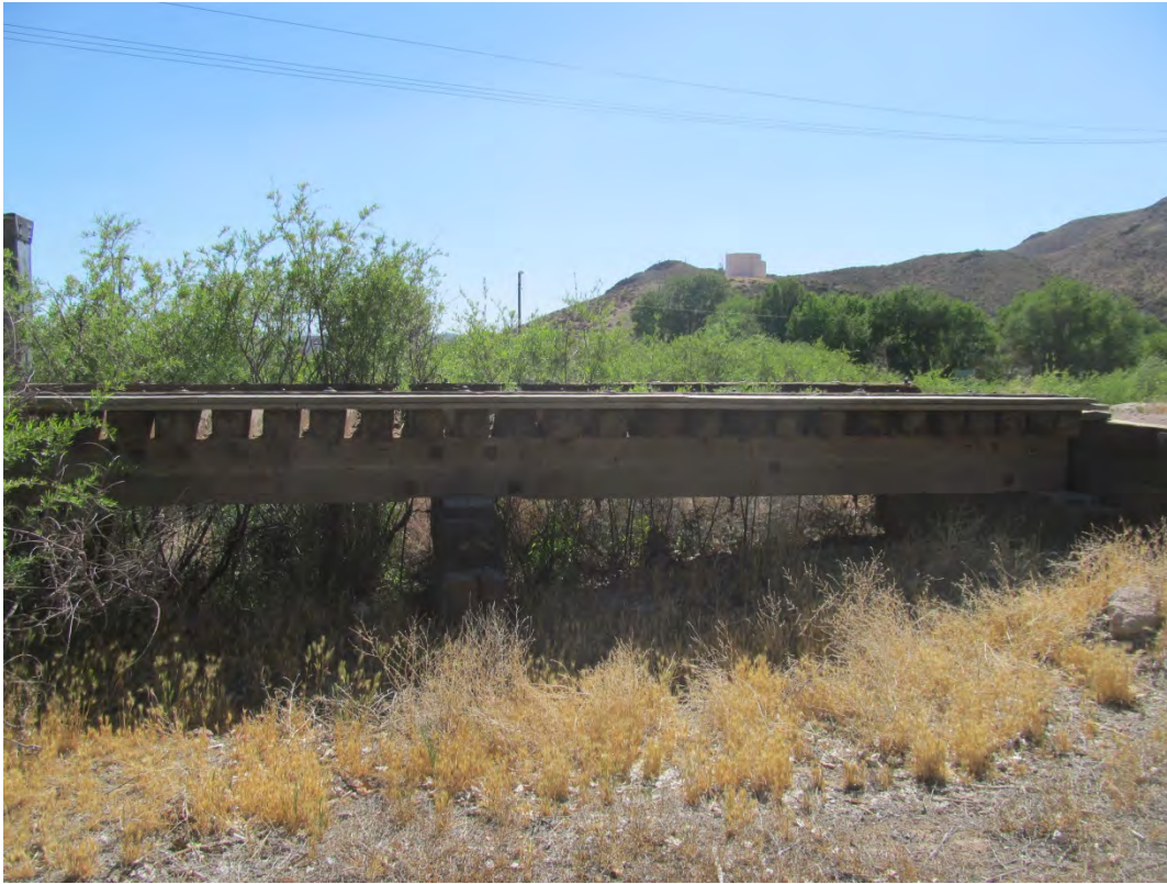
Figure 28. Profile of C&P bridge west approach deck, view southwest.
