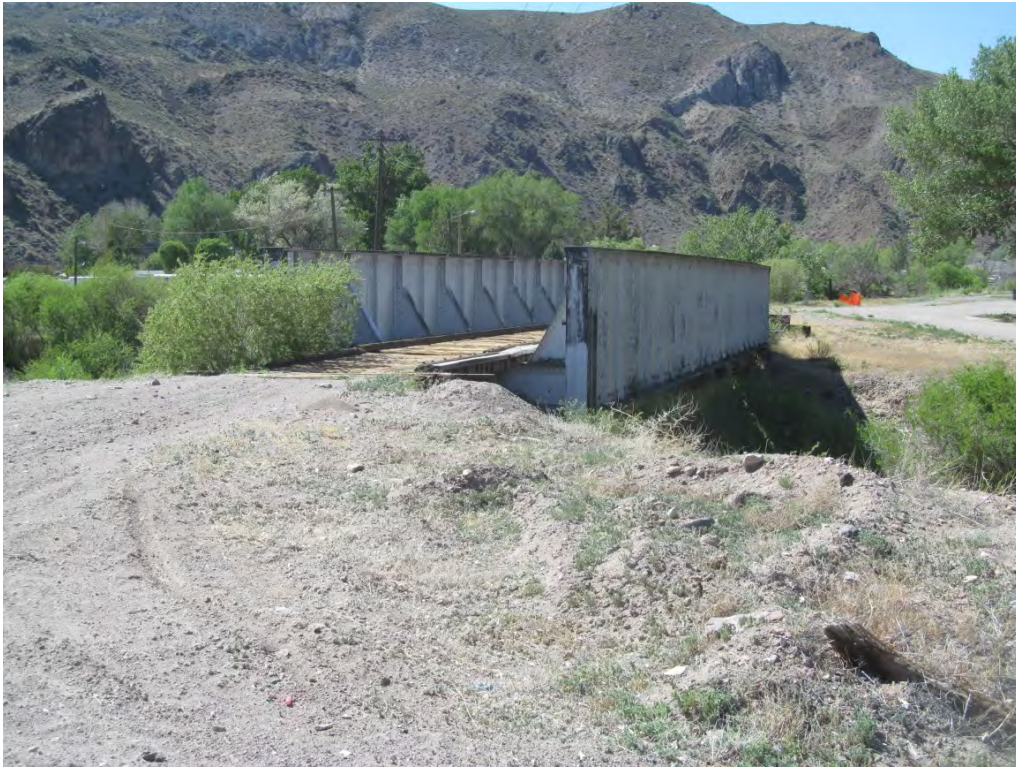
Figure 24. East end of C&P bridge, view northwest.
