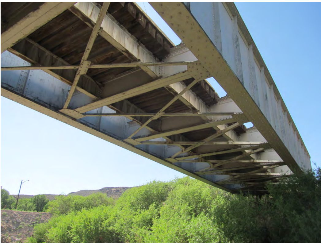
Figure 27. Underside of C&P bridge showing I-beam construction.
