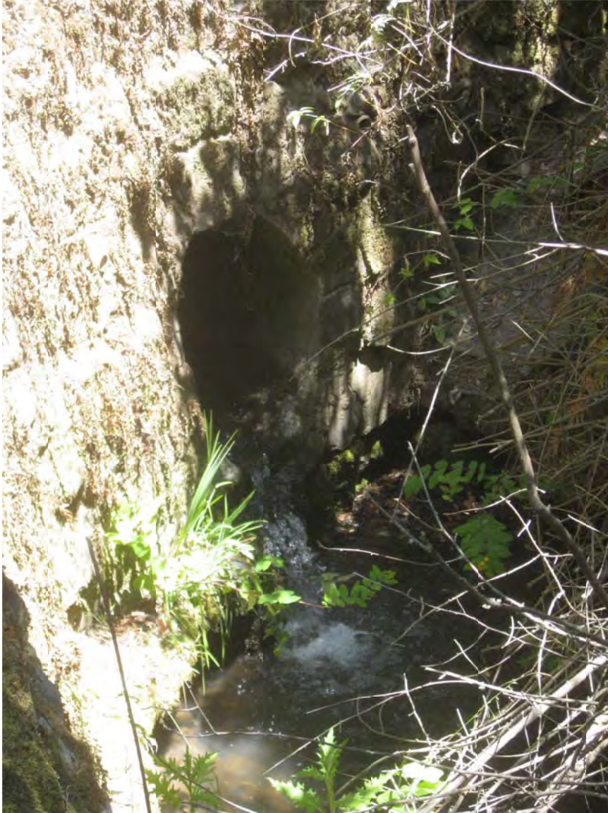
Figure 1, Culvert on lower fire trail, near Botanic Garden
