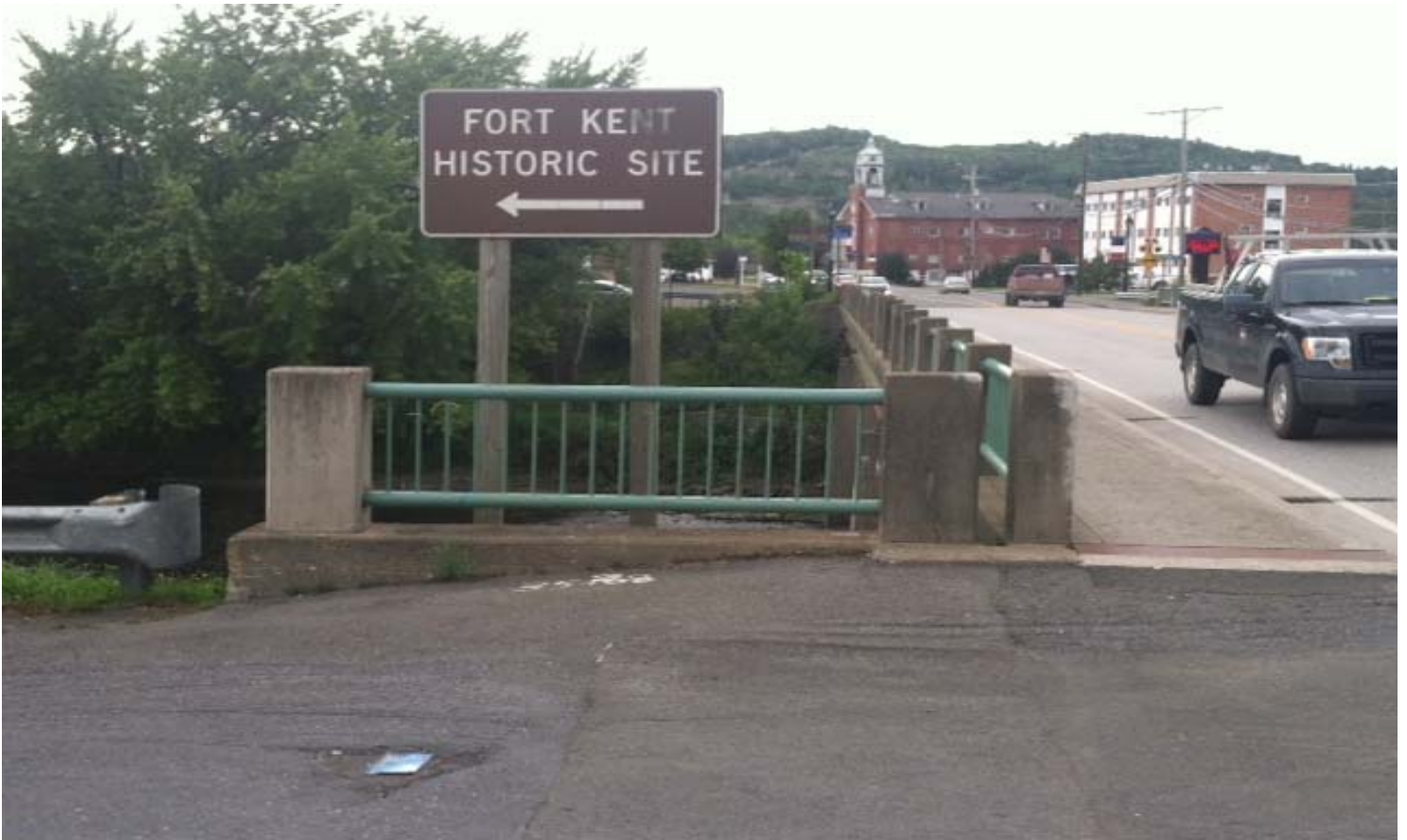
Photo 1: Fish River Bridge - Main Street at the mouth of Block House Road looking northeast
