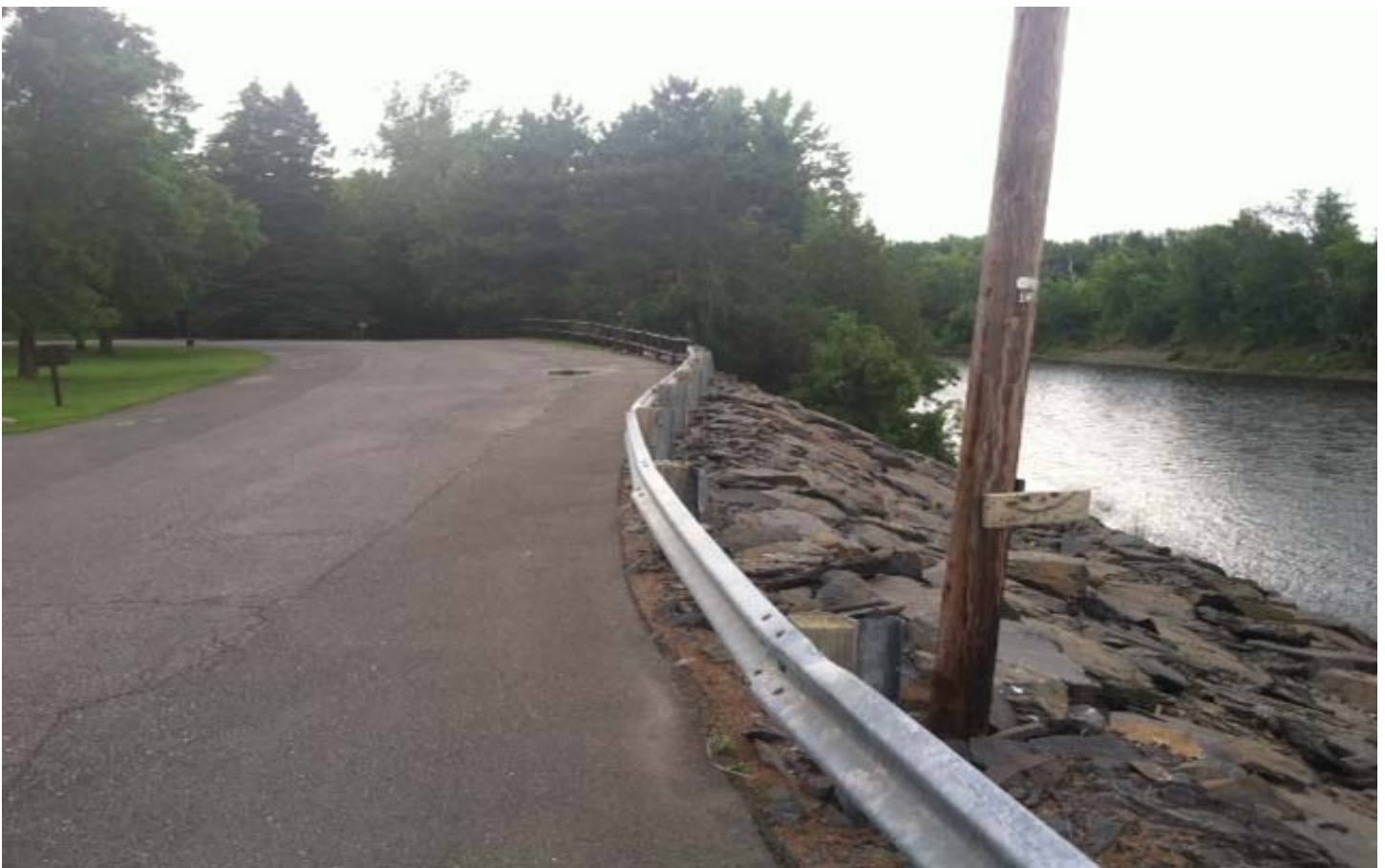
Photo 4: Block House Road adjacent to rip rap descending to river looking northwest
