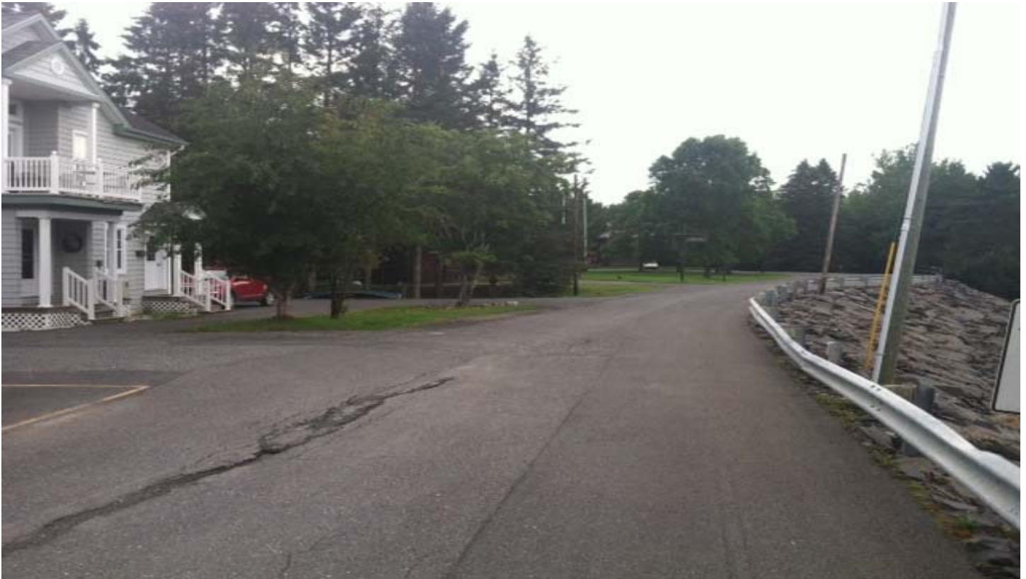
Photo 3: Block House Road adjacent to Old Fire House apartments looking northwest.
