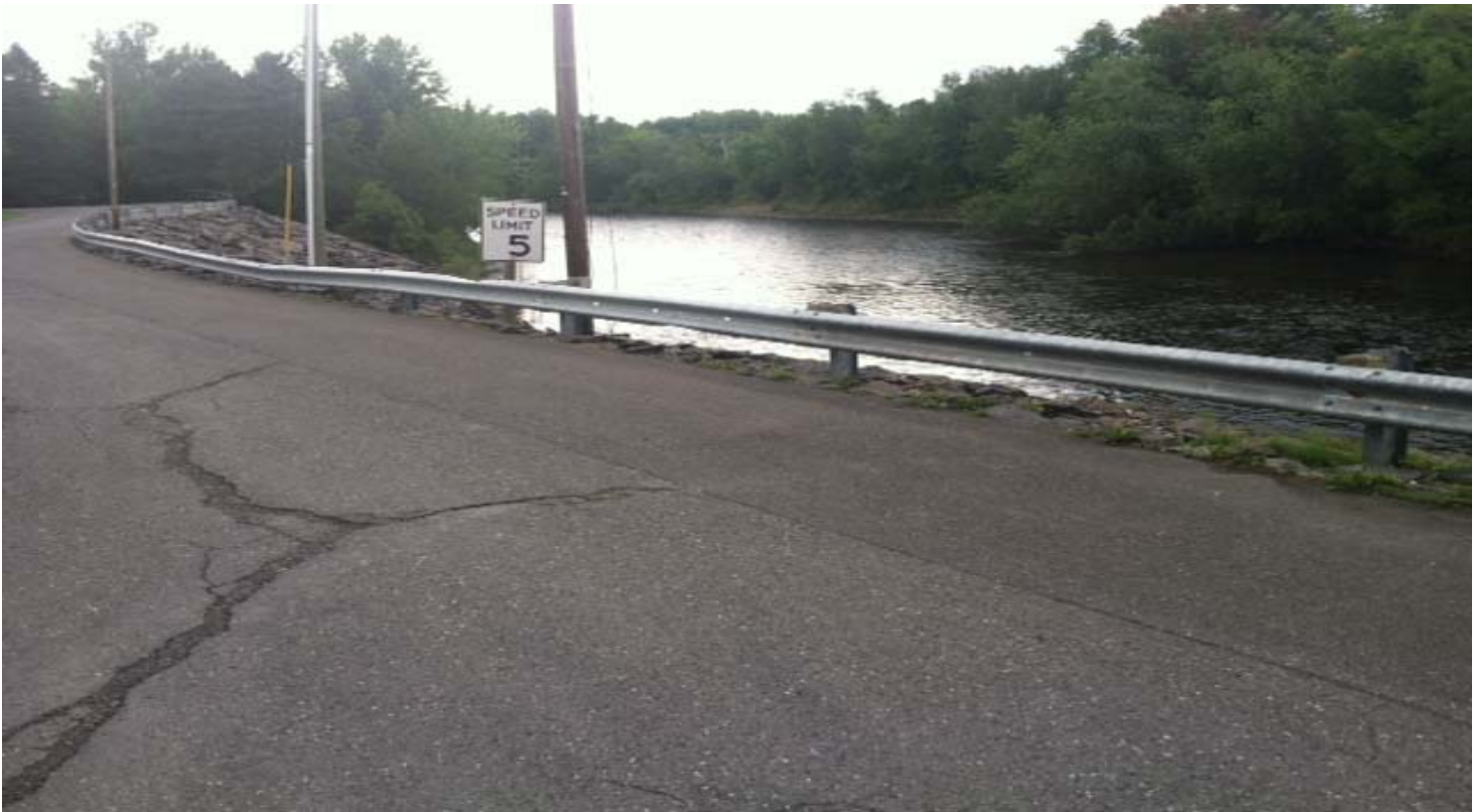
Photo 2: Block House Road looking north
