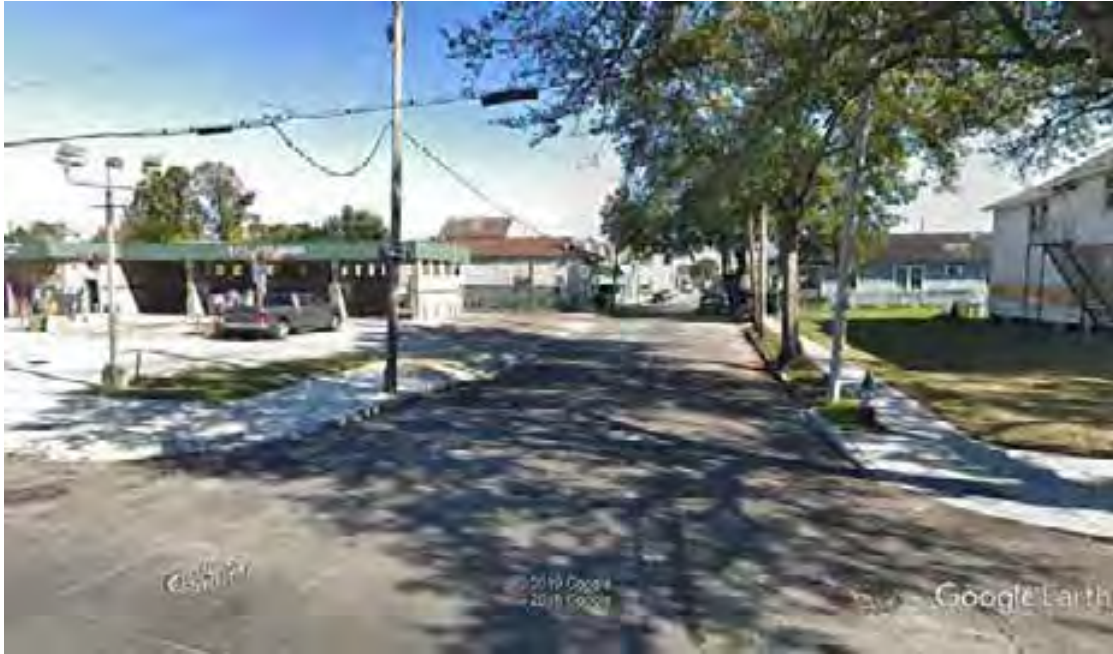
Figure 19. Representative view of Dryades St. (Google Street View, 11/2018), looking northeast from Louisiana Ave. Scope of work along ten blocks from Louisiana Ave. to Philip St. includes construction of ADA ramps at street corners, and replacement of roadway curbs, and existing water and drainage pipes and structures within the existing right-of-way. This area is located within the NRHP listed Central City Historic District.
