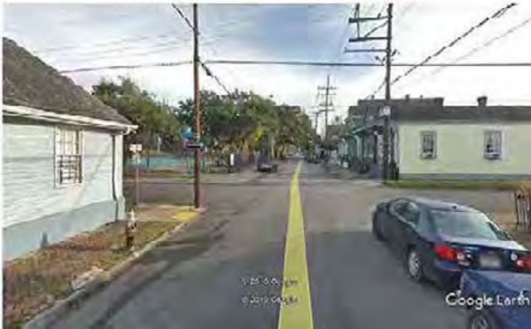
Figure 22. View of intersection at Chippewa and Third St. (Google Street View, 12/2018), looking northeast. Scope of work entails replacement of water lines; construction of a green intersection at this location, including replacement of roadway, construction of green drainage system under roadway, installation of permeable paver crosswalks and gutters, construction of vegetated street basins, narrowing of the roadway; and construction of ADA ramps and replacement of curbs and sidewalk. This area is located within the NRHP listed Irish Channel Historic District.
