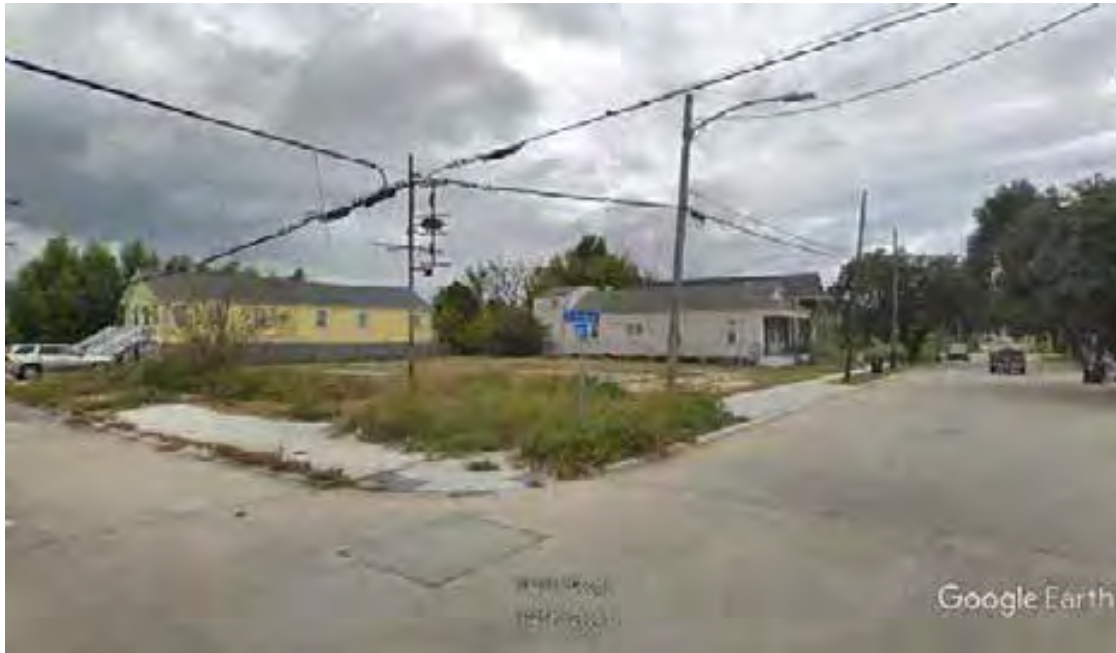
Figure 10. View of Stormwater Lot 2, 3200 Jackson Ave. (Google Street View 11/2018), looking northwest. Scope of work includes demolition/replacement of concrete sidewalk and curb; excavation of property; construction of surface retention ponds, new catch basins, two concrete runnels and footbridges; and installation of plant material. This area is not within an a NRHP listed/eligible historic district.
