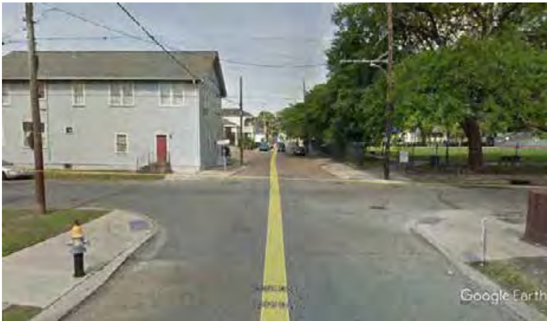
Figure 13. View of intersection at Annunciation St. and Third St. (Google Street View, 11/2018), looking northeast. Scope of work includes replacement of water lines; construction of a green intersection at this location, including replacement of roadway, construction of green drainage system under roadway, installation of permeable paver crosswalks and gutters, construction of vegetated street basins, narrowing of the roadway; and construction of ADA ramps and replacement of curbs and sidewalk. This area is located within the NRHP listed Irish Channel Historic District.
