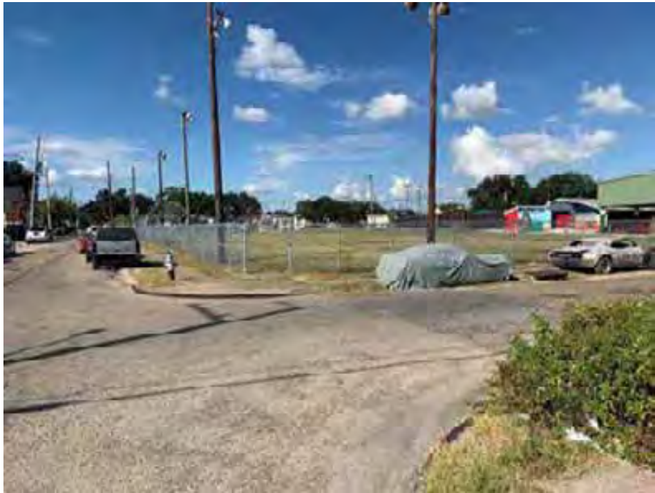
Figure 6: Proposed stormwater park at the current Taylor Playground as shown standing at the Derbigny Street and 3 rd Street intersection
