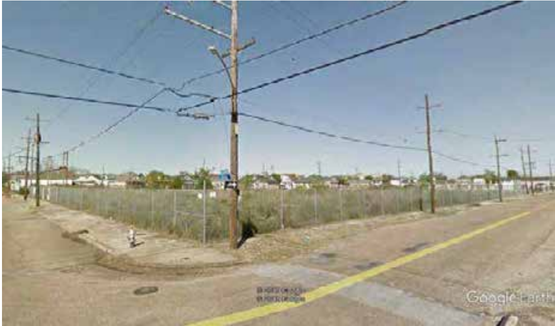
Figure 26. View of Saratoga Square, looking west (Google Earth Street View, 11/2018). Scope of work includes demolition/replacement of sidewalks, curbs, ADA ramps, and small segments of roadway around the perimeter of the city block; demolition/clearing of block; excavation and construction of multiple, interconnected detention ponds for the collection of stormwater; construction of supporting surface and underground drainage structures, interior park sidewalks; and planting of trees, shrubs, and groundcover. This area is located within the NRHP listed Central City Historic District.
