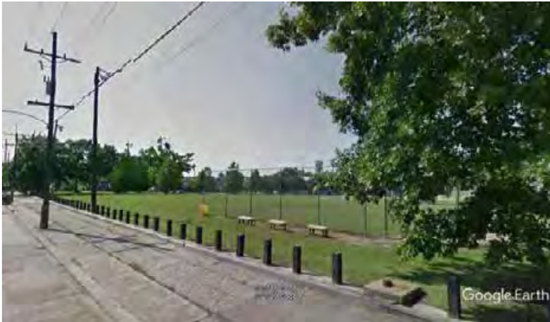
Figure 17. View of Annunciation Park, looking northeast (Google Street View, 11/2018). Scope of work includes demo/replacement of baseball backstop, excavation for and placement of underground stormwater storage tanks, repair and improvements to these areas following the placement of tanks, and planting of trees along Annunciation St. On the park perimeter, scope will include the demo/replacement of concrete sidewalks. This area is located within the NRHP listed Lower Garden Historic District.
