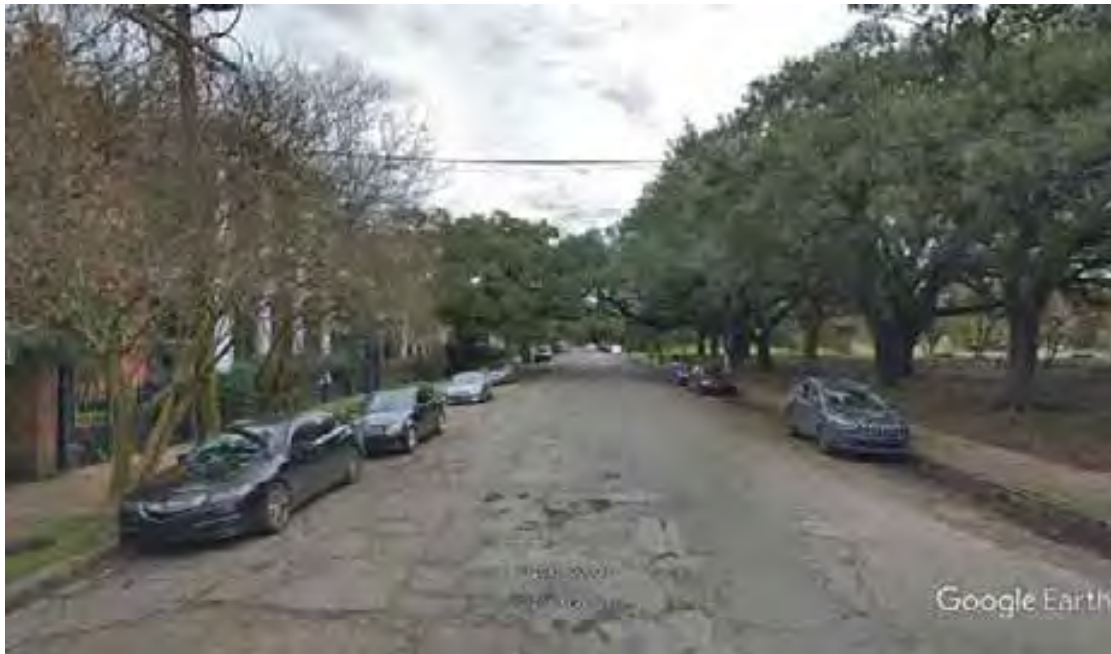
Figure 25. Representative view of Coliseum St. (Google Street View, 1/2019), looking northeast from Race St. Scope of work along four blocks from Race St. to Melpomene St. includes, installation of yellow thermoplastic pavement striping (crosswalks and no parking zones) and permeable paver gutters, construction of ADA ramps, and replacement of curbs, roadway, and existing water and drainage pipes and structures within the existing right-of-way. This area is located within the NRHP listed Lower Garden Historic District.
