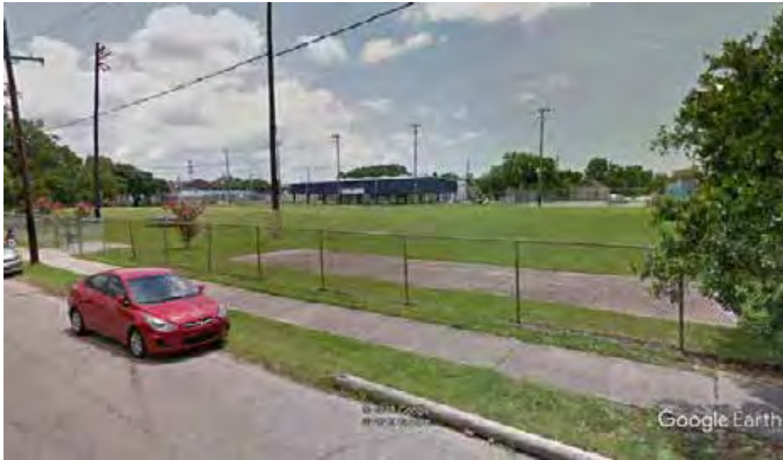
Figure 15. View of A.L. Davis Park, looking southeast (Google Street View, 11/2018). Scope of work includes demo/replacement of concrete pads and sidewalk, excavation for and placement of underground stormwater storage tanks, and the repair and improvements to these areas following the placement of tanks. On the park perimeter, scope will include the demo/replacement of concrete sidewalks, concrete curb, and concrete roadway, construction of ADA ramps. This area is surrounded by the NRHP listed Central City Historic District.
