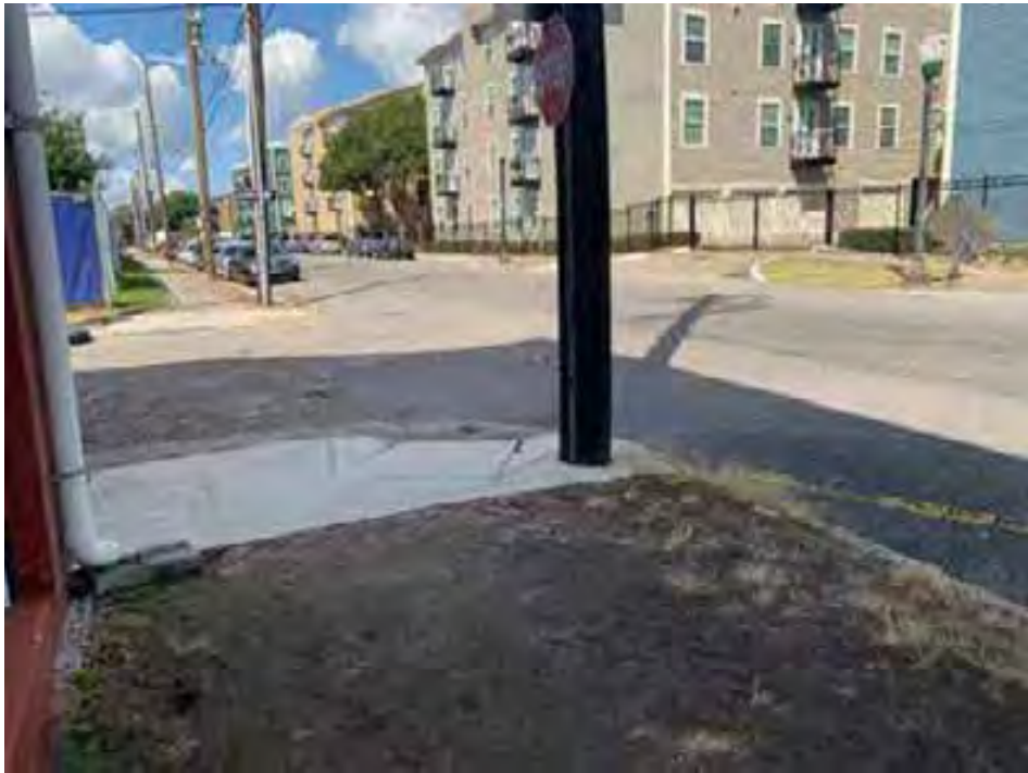
Figure 16: Typical conditions of Saint Thomas Street, as seen from its intersection with Race Street
