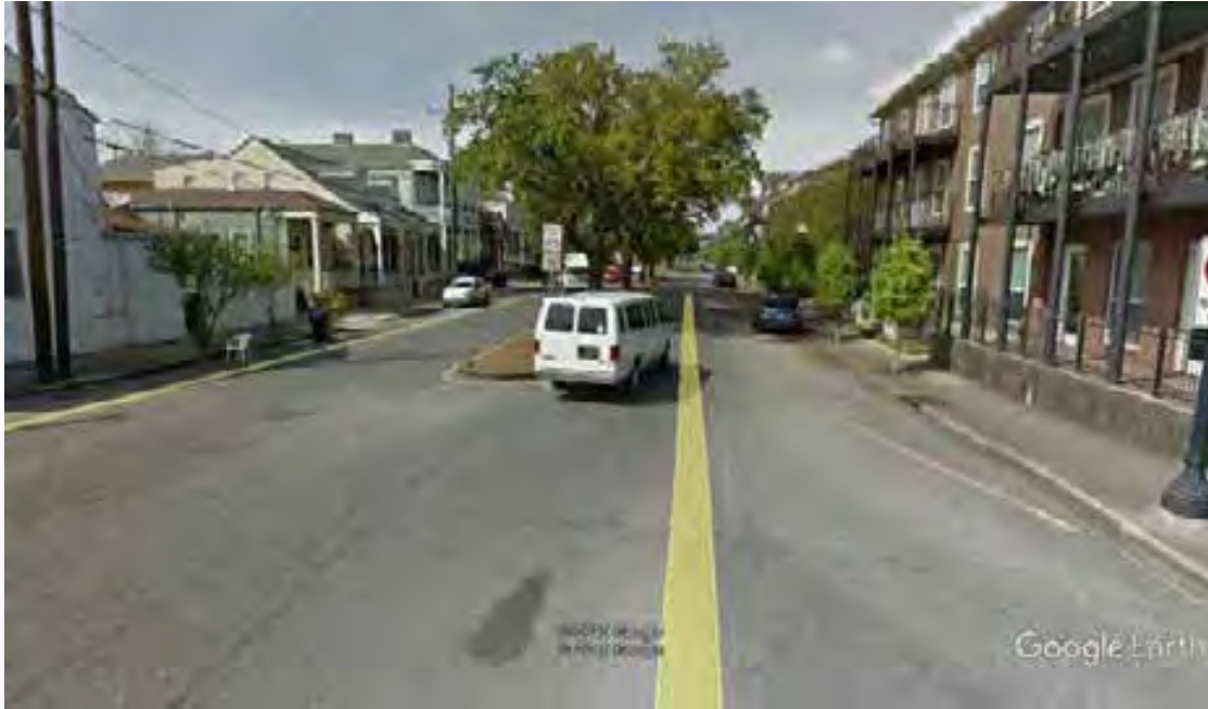
Figure 12. Representative view of Annunciation St. (Google Street View, 11/2018), looking northeast from Race St. Scope of work along three blocks from Race St. to Calliope St. includes replacement of roadway, construction of ADA ramps at street corners, installation of permeable paver crosswalks and gutters, re-striping parking lane, and replacement of existing water and drainage pipes and structures within the roadway. This area is located within the NRHP listed Lower Garden Historic District.
