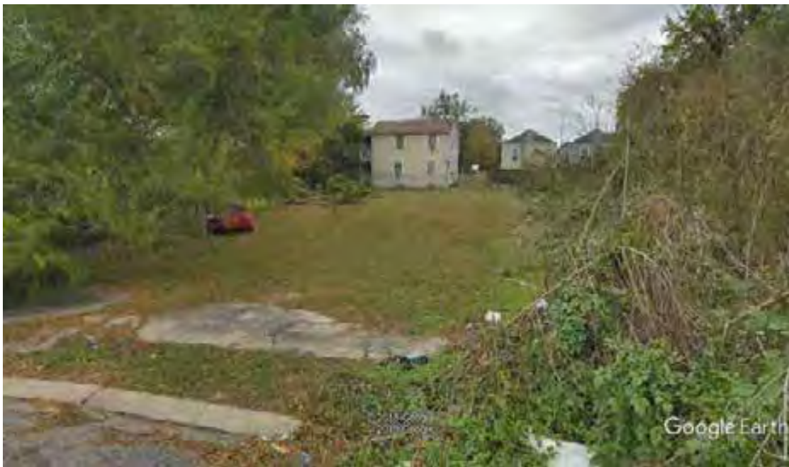
Figure 9. View of Stormwater Lot 1, 3621/3623 3 rd St. (Google Street View 11/2018), looking northeast. Scope of work includes removal of one 24" willow tree; demolition/replacement of concrete sidewalk, curb, and asphalt roadway; excavation of property; construction of surface dry detention ponds, new catch basins, a concrete runnel and footbridge; and installation of plant material. This area is not within an a NRHP listed/eligible historic district.
