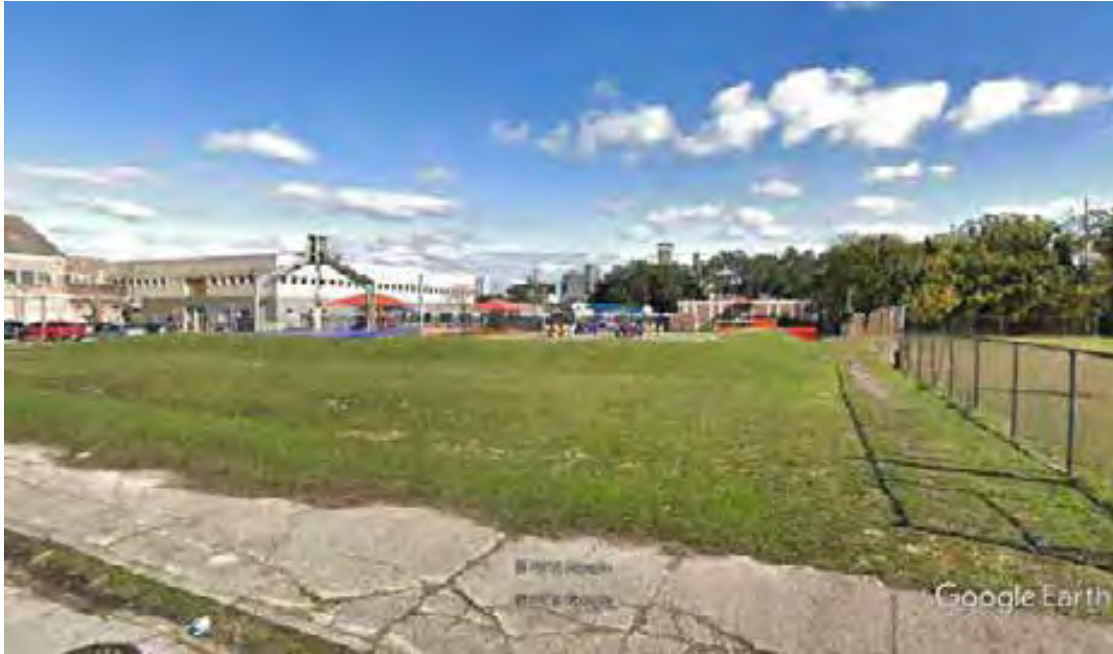
Figure 28. View of Van McMurray Playground, looking northeast (Google Earth Street View, 12/2018). Scope of work includes removal of paving material, four trees, four bollards, a basketball court, fences, gates, backstop, a driveway apron, and sidewalks; excavation for and placement of underground stormwater storage tanks; and the repair and improvements to these areas following the placement of tanks, including the planting of trees, installation of permeable pavers, and chain link fence. On the park perimeter, scope will include the demolition of bollards, and demo/replacement of concrete sidewalks. This is not within a listed or eligible NRHP District.
