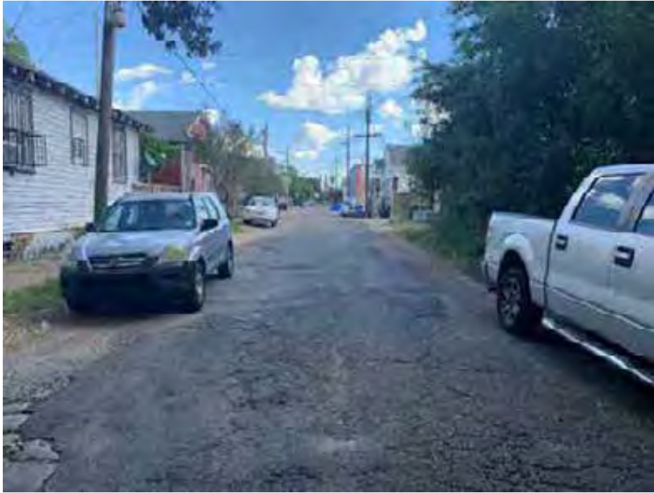
Figure 19: Typical conditions of Saint Thomas Street, as seen from its intersection with Washington Street, where the road reconstruction with bioswales is proposed
