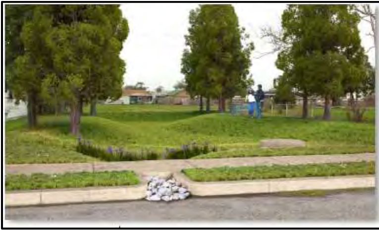
Photograph 1. An example of a completed stormwater lot
