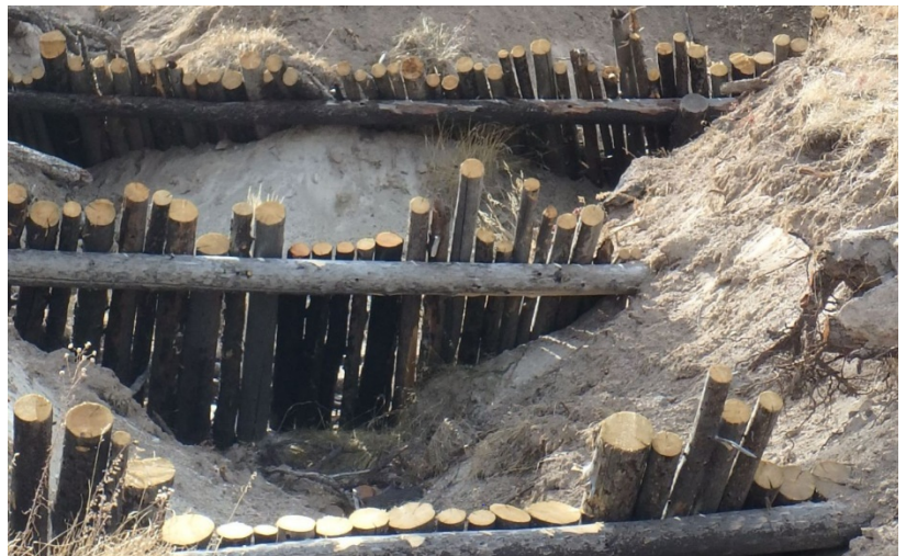
Figure 2. An example of a bank stabilization technique employed in Santa Clara Pueblo that uses natural materials. Source: Santa Clara Pueblo Forestry.
