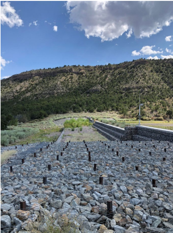
Figure 3. A mitigation project installed in the canyon to treat water runoff before it reaches the main stem of the creek improves the resiliency of the watershed while the natural vegetation recovers.
