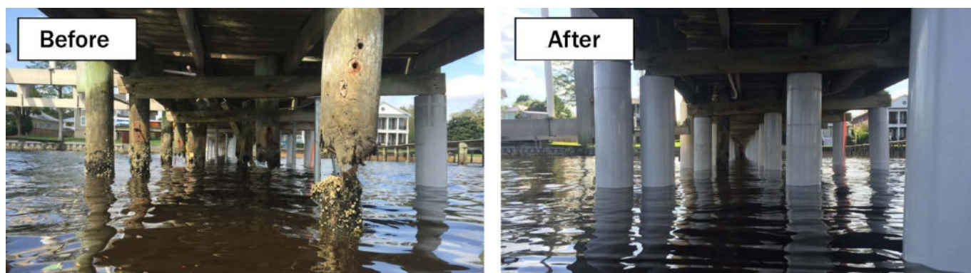
Figure 5.5.2. Fit aging piles with jacket encasements to strengthen and protect them (Source: Shoreline Plastics, No Date).
