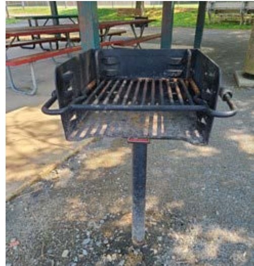
Figure 5.1.3. Some park equipment can be embedded deep enough into the ground to improve stability.
