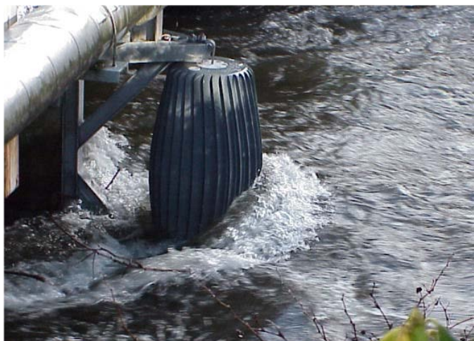
Figure 1.4.19. A debris sweeper can be attached directly to a pier to deflect debris (FHWA, 2005).
