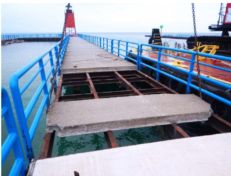
Figure 5.5.3. Improve pier performance during future storms by replacing storm-damaged pre-cast concrete pier deck panels with reinforced cast-in-place concrete (Source: U.S. Army Corps of Engineers, No Date).
