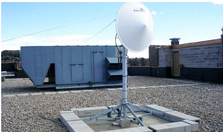
Figure 4.4.2. Rooftop antennas often are mounted using ballast sleds.
