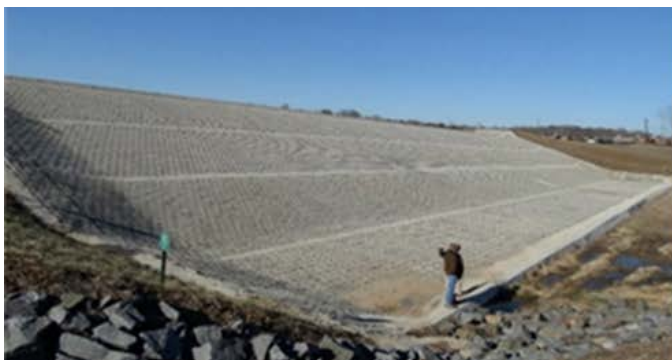
Figure 2.3.14. ACBs (left) and RCC (right) can protect spillways from overtopping erosion.
