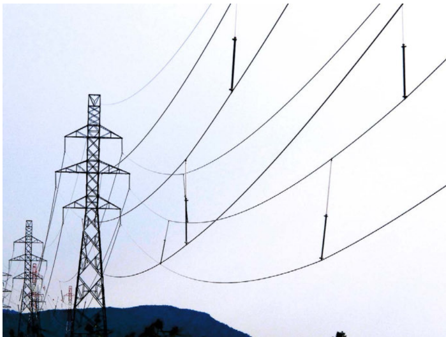
Figure 4.3.3. Interphase spacers can be used to help mitigate conductor gallop. (Source: INMR, 2021)
