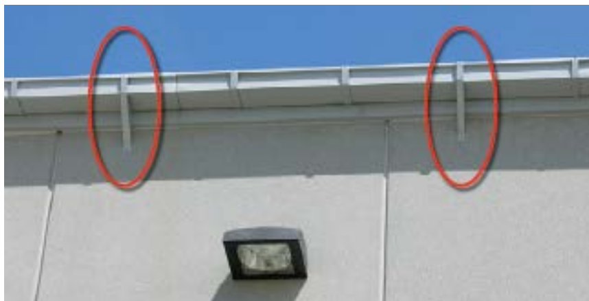
Figure 3.3.2.4. Sheet metal straps (circled) attached to an existing gutter to increase wind uplift resistance.
