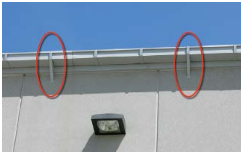
Figure 3.3.1.10. Sheet metal straps (circled) attached to an existing gutter to increase wind uplift resistance.
