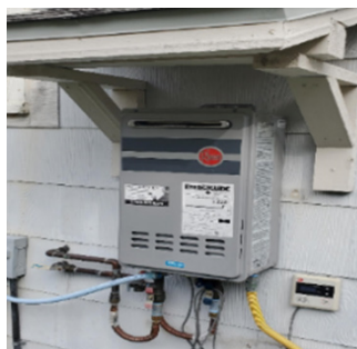
▲ A gas-fired flash water heater affixed to the building's exterior siding, making it part of the building and therefore covered.
