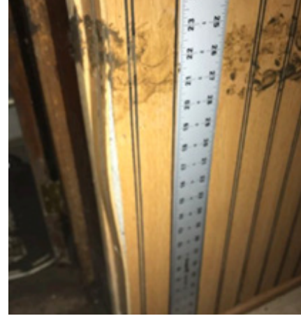
▲ Example of a questionable photograph: no flood debris, would not support a recommendation of damage by or from flood.
