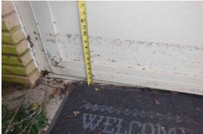
▲ Example of a good photograph: clear picture of the flood debris showing the waterline , from the floor slab to the water limit, with measurement .
