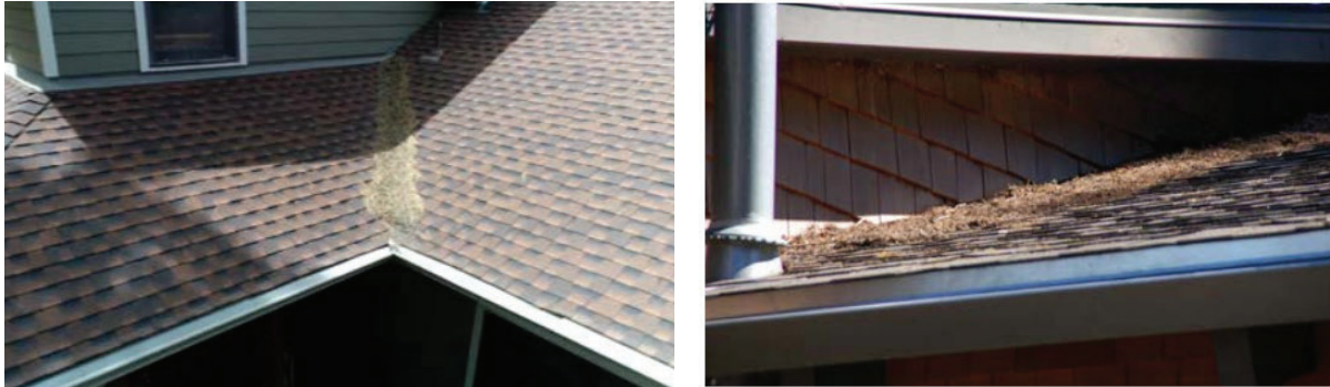
Figure 4. Vegetative debris (e.g., pine needles) and embers can accumulate at roof valleys (left, Source: NFPA®) and at the base of the wall on the roof of this split-level house (right, Source: Stephen Quarles).
