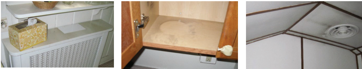
Figure 1. Photos of light soot levels associated with moderate smoke and ash damage. (Photos provided by John DiMenno of Romualdi Davidson & Associates and used with permission.)
