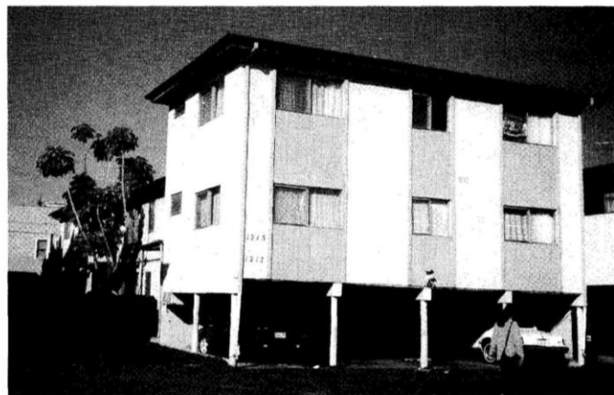
Figure 1-4 Short-side-open SWOF building type without damage (image credit: EERI, 1996).
