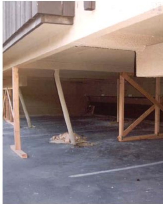
Figure 1-7 Northridge Gardens apartment building following the Northridge earthquake with direction of drift perpendicular to the open front (image credit: Schierle, 2003).
