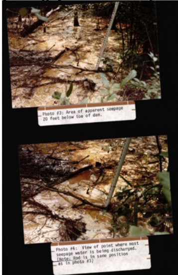
Figure 2 - Photographs from 1981 LRCC Inspection
