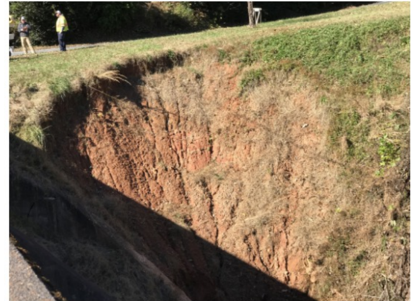
West Abutment Slough
