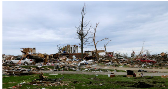
Figure 9. Debris on Private Property
