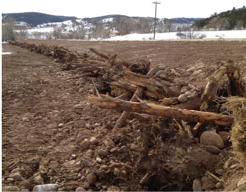
Figure 4-6: Bioengineering Using Engineered Woody Debris
