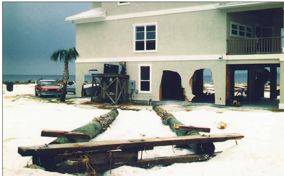
Figure 1-12. Pier piles were carried over 2 miles by the storm surge and waves of Hurricane Opal (1995) before coming to rest near this elevated house in Pensacola Beach, Florida.
