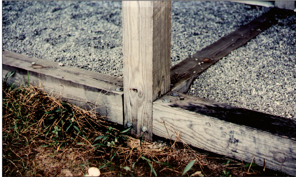
Figure 2-3. Compression strut at base of a wood pile. Struts provide some lateral support for the pile, but very little resistance to rotation.
