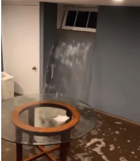
Figure 4. Surface water entering below-grade dwelling unit through window (left); NYPD officer searching flooded basement where three fatalities occurred (right)
