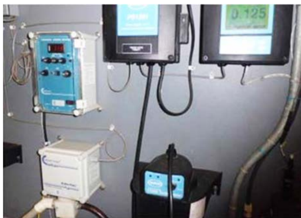
Figure 4.2.4. Elevating instrumentation can protect it from damage during flooding. (Source: U.S. EPA, 2014)
