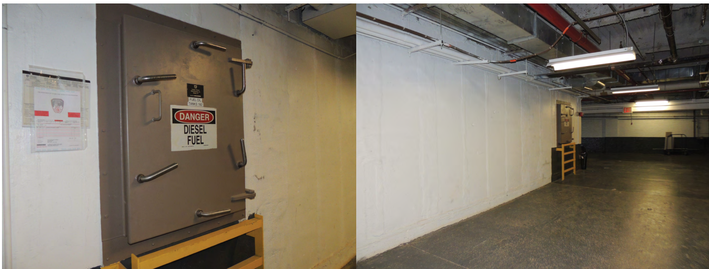
Figure 5-5. Dry floodproofed fuel tank enclosure in basement of a high-rise building
