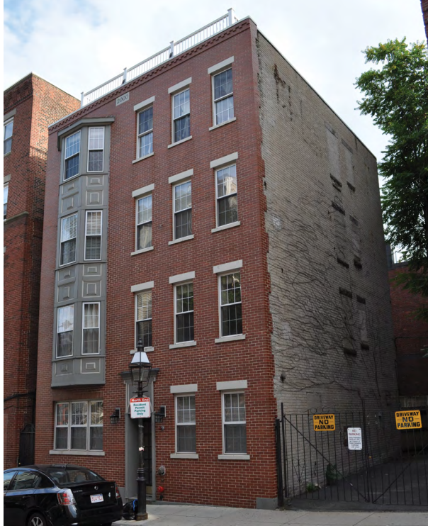
Figure 1-1. Representative multi-family building
