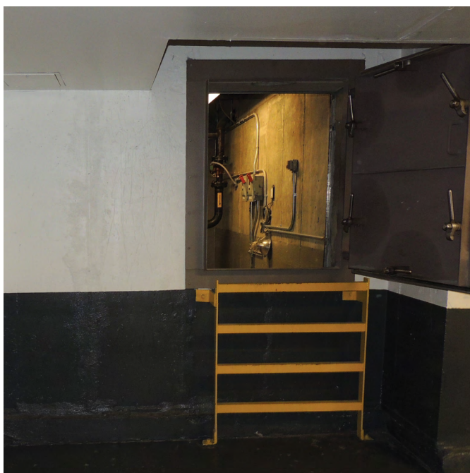
Figure 5-8. Example of basement that integrated wet and dry floodproofing techniques. The area in front had about 6 inches of floodwater, and the dry floodproofed fuel pump room (visible through doorway) continued to operate.
