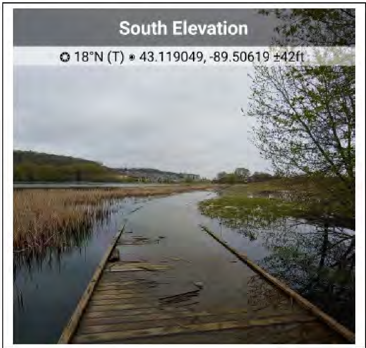
Photo 47: Site 35 (May 2019) taken at 43.11905, -89.50619. Graber Pond. View of damaged boardwalk.
