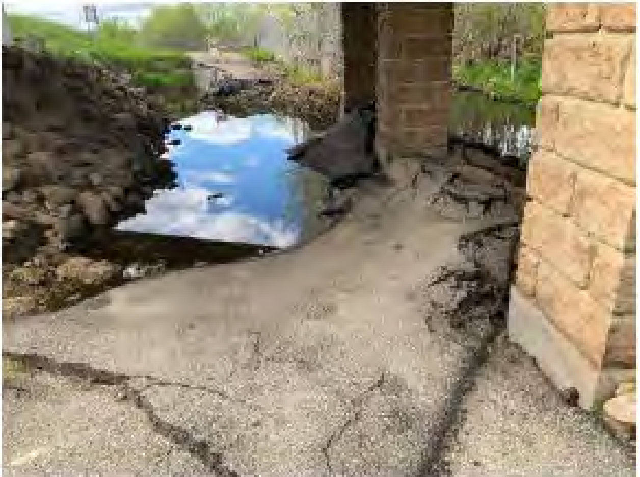
Photo 51: Site 37. Taken at 43.11126, -89.53614. Airport Road underpass. View of damaged asphalt trail and displaced rip-rap.
