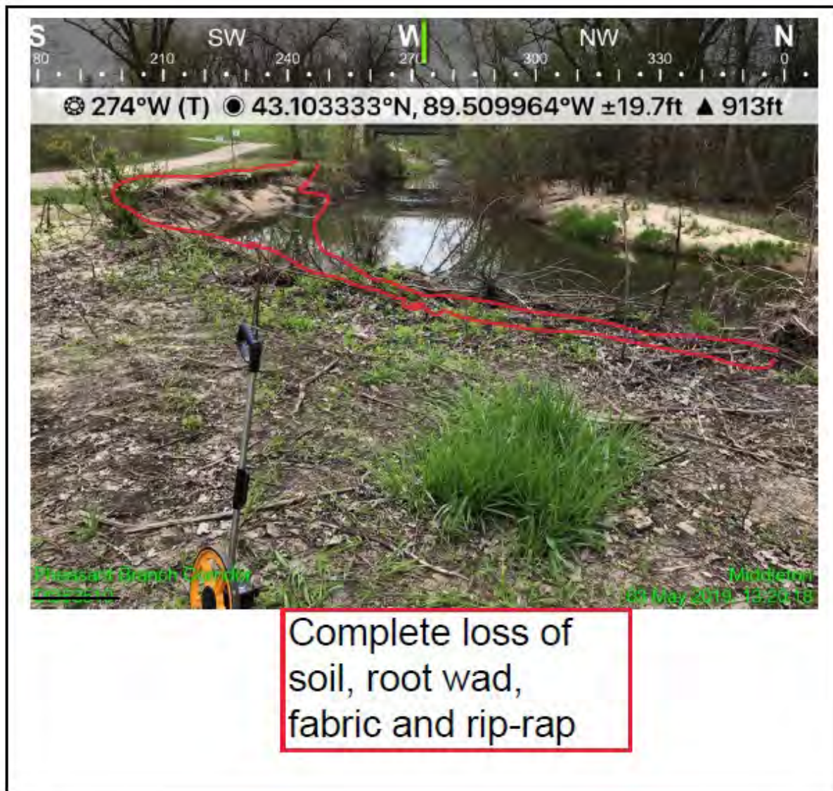
Photo 5: Site 4 (May 2019) taken at 43.10333, -89.50996. View of eroded south streambank facing Parmenter Street.
