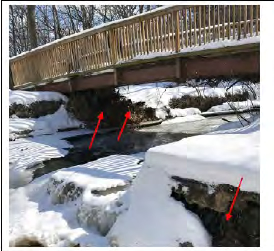
Photo 35: Sites 20 & 21 (March 2019) taken at 43.103065, -89.498190. View of displaced rip-rap surrounding pedestrian bridge abutment. Trail will be resurfaced to pre-disaster condition.
