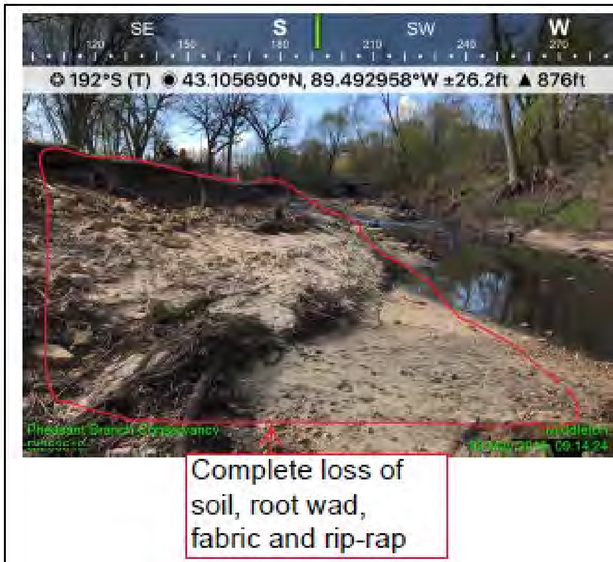
Photo 41: Site 27 (May 2019) taken at 43.10569, -89.49296. View of eroded streambank.
