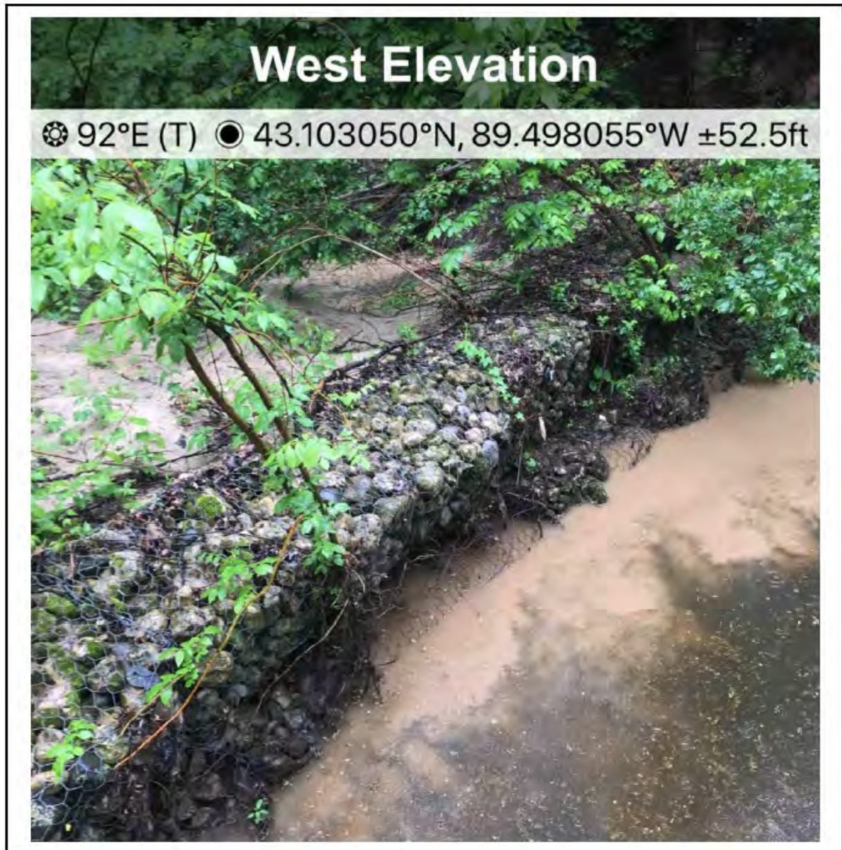
Photo 37: Site 23 (May 2019) taken at 43.103050, -89.498055. View of damaged gabion wall.
