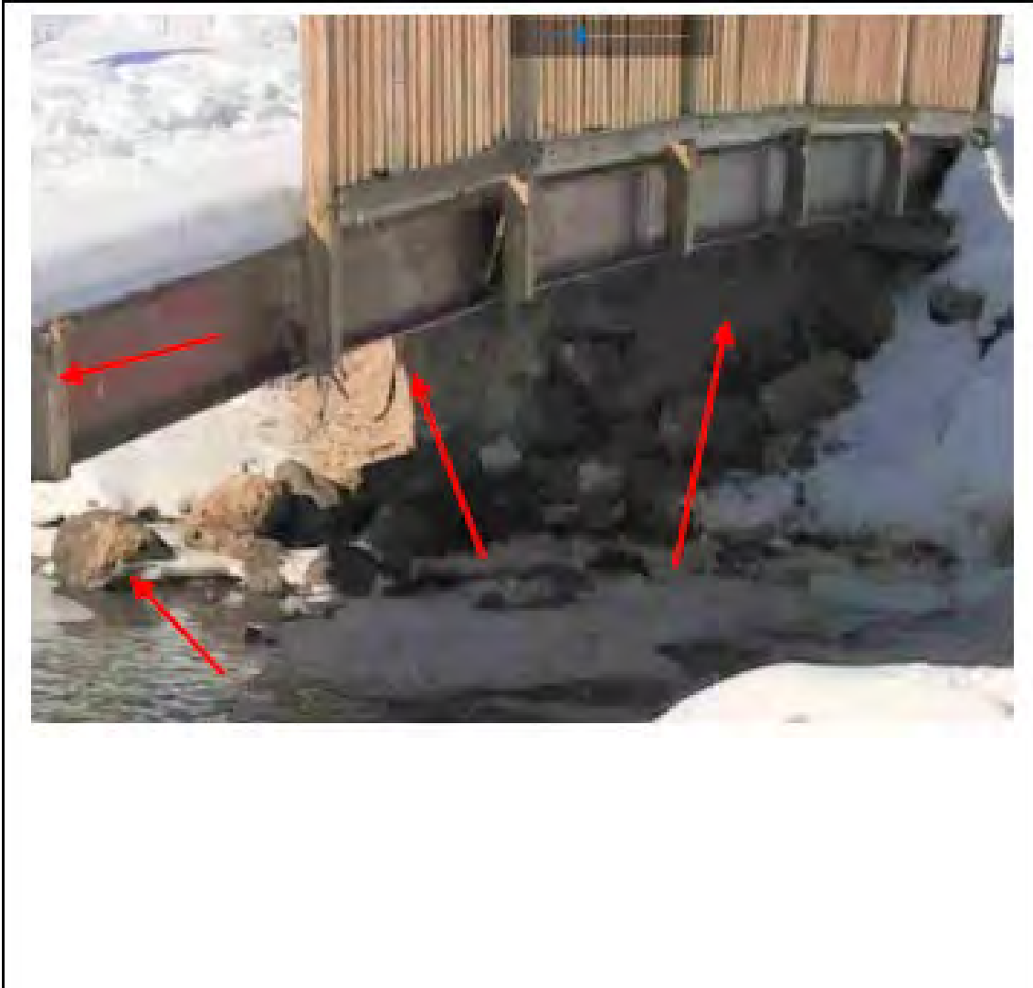
Photo 10: Site 6 (March 2019) taken at 43.103016, -89.509429. View of eroded rip-rap on abutment of damaged pedestrian bridge.
