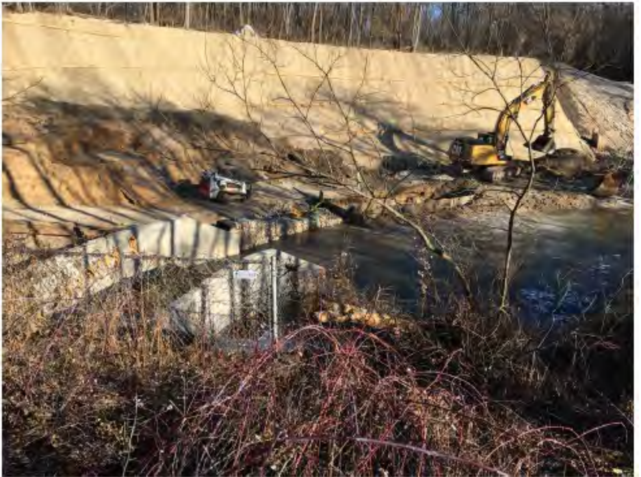
Photo 30: Site 16 (December 2019). Photo taken at Park Street facing east. View of repairs to eroded north streambank. Work completed in 2019.
