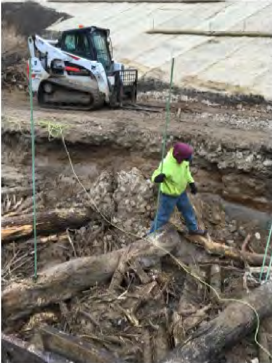
Photo 31: Site 16 (December 2019). Park Street. View of installation of footer logs and root wads to eroded north streambank. Work completed in 2019.
