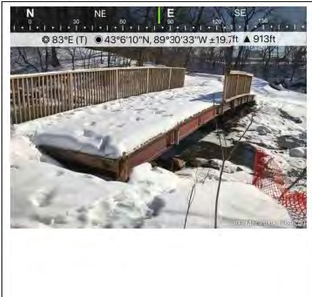
Photo 9: Sites 6 & 7 (March 2019) taken at 43.103016, -89.509429. View of damaged pedestrian bridge and eroded rip-rap on abutment. Asphalt path to be resurfaced.
