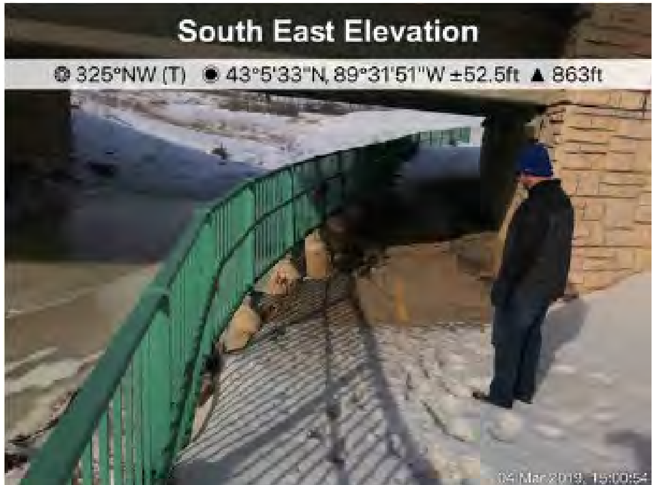
Photo 2: Site 2 (March 2019) taken at 43.092573, -89.531055. View of eroded under pass of Market Street bridge.
