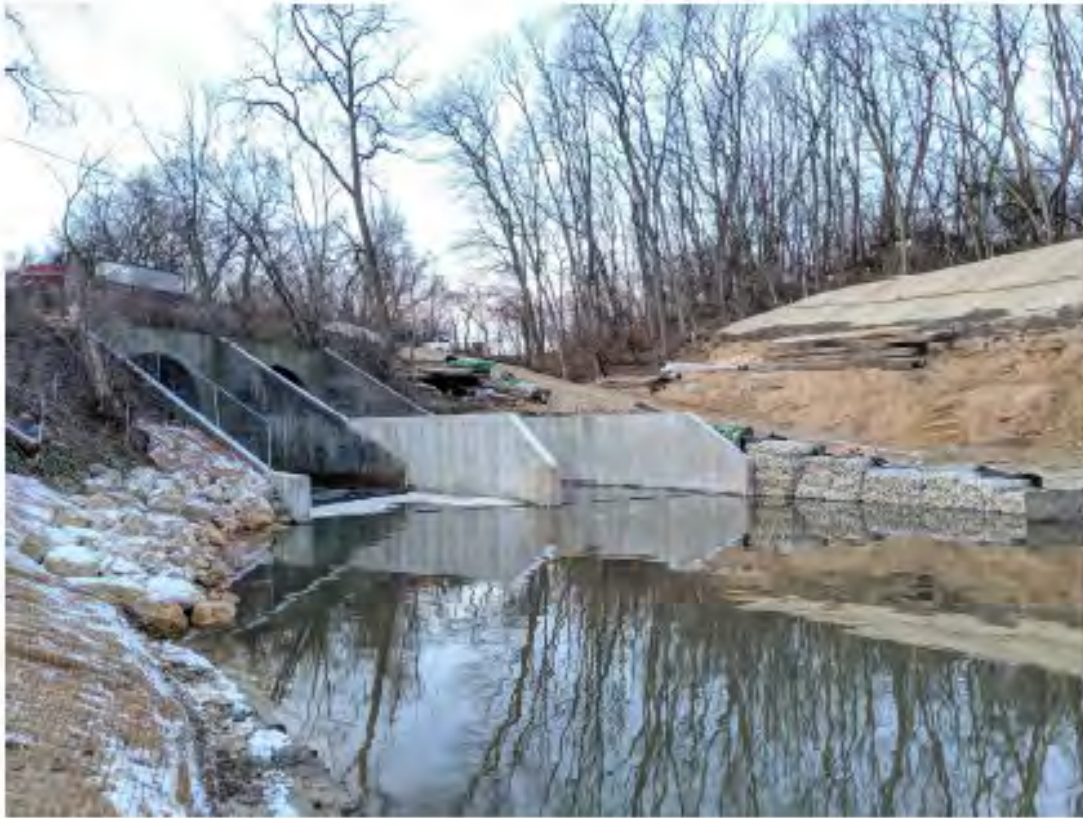
Photo 29: Site 16 (December 2019). View of work to extend culvert aprons. Facing west towards Park Street.
