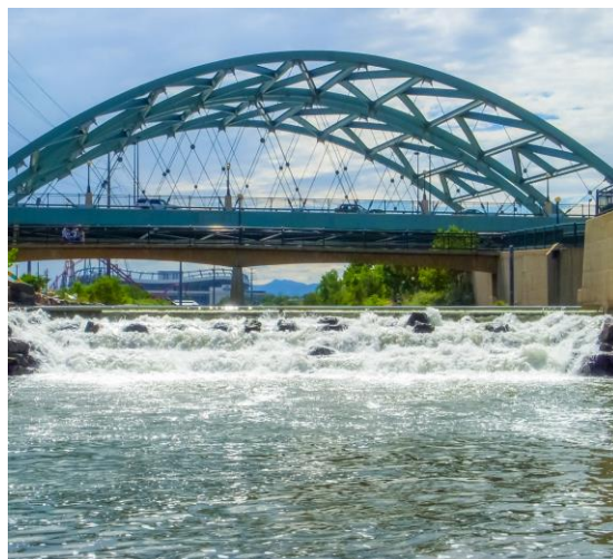
Figure 1. Mitigation in Confluence Park, Denver, Colorado
