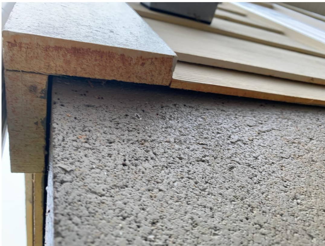
Figure 4. Homeowners should block gaps between siding and foundations (such as the one pictured here) using firestopping materials such as mineral wool or fire-resistant sealants to prevent embers, hot gases, and flames from entering and becoming trapped.
