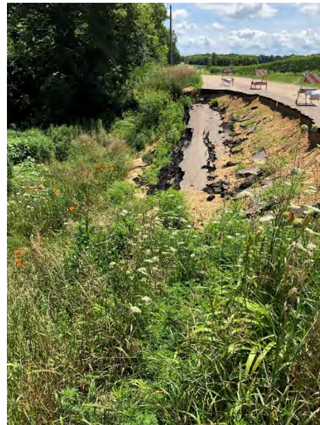
Upland area south of data point AU2: Loran Road erosion.
