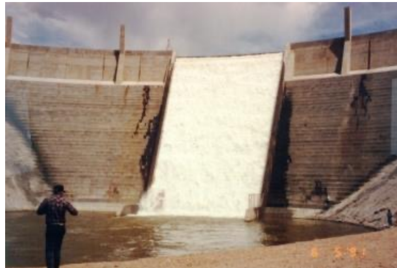
Santa Cruz Dam, NM
