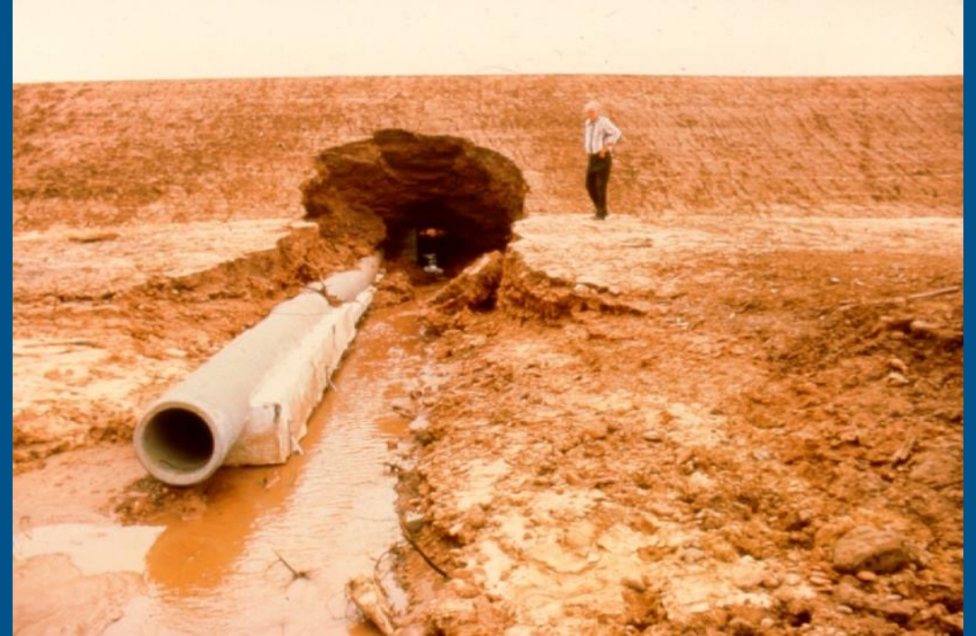
Pre-cast bell-and-spigot pipe outlet
