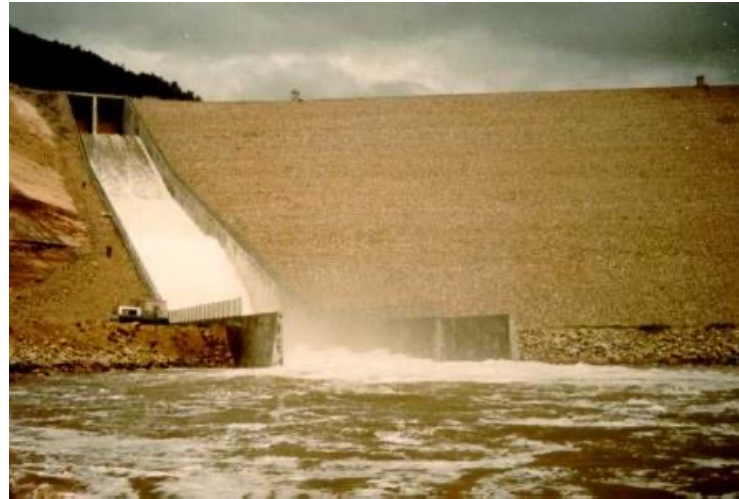
McPhee Dam, CO
