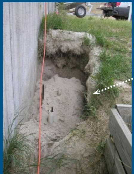
Sinkhole adjacent to outlet works control house.
