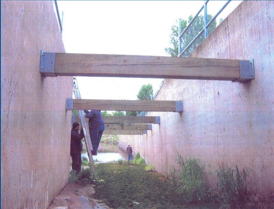
Jamestown Dam, ND Outlet works stilling basin
