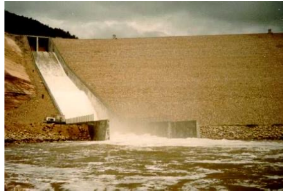
McPhee Dam, CO
