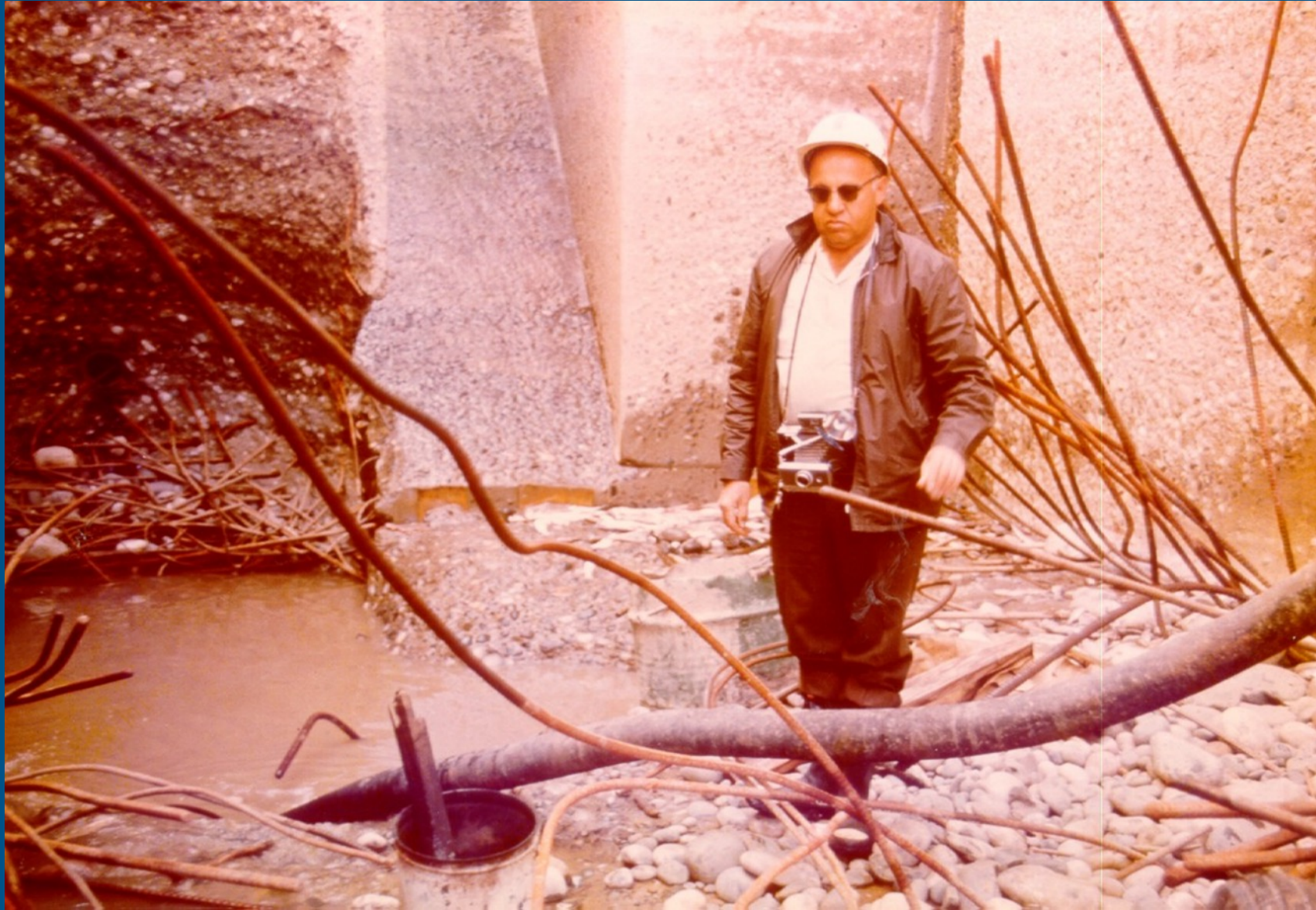
Navajo Dam, NM
