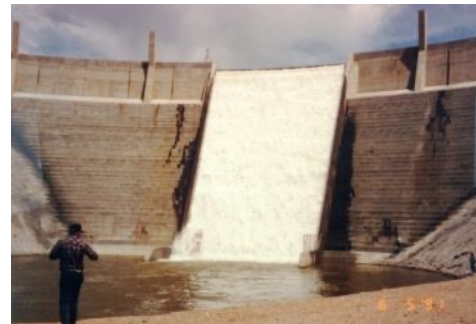
Santa Cruz Dam, NM
