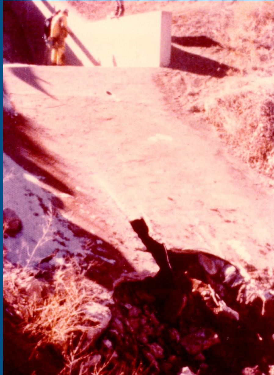
Unknown Dam, CO
