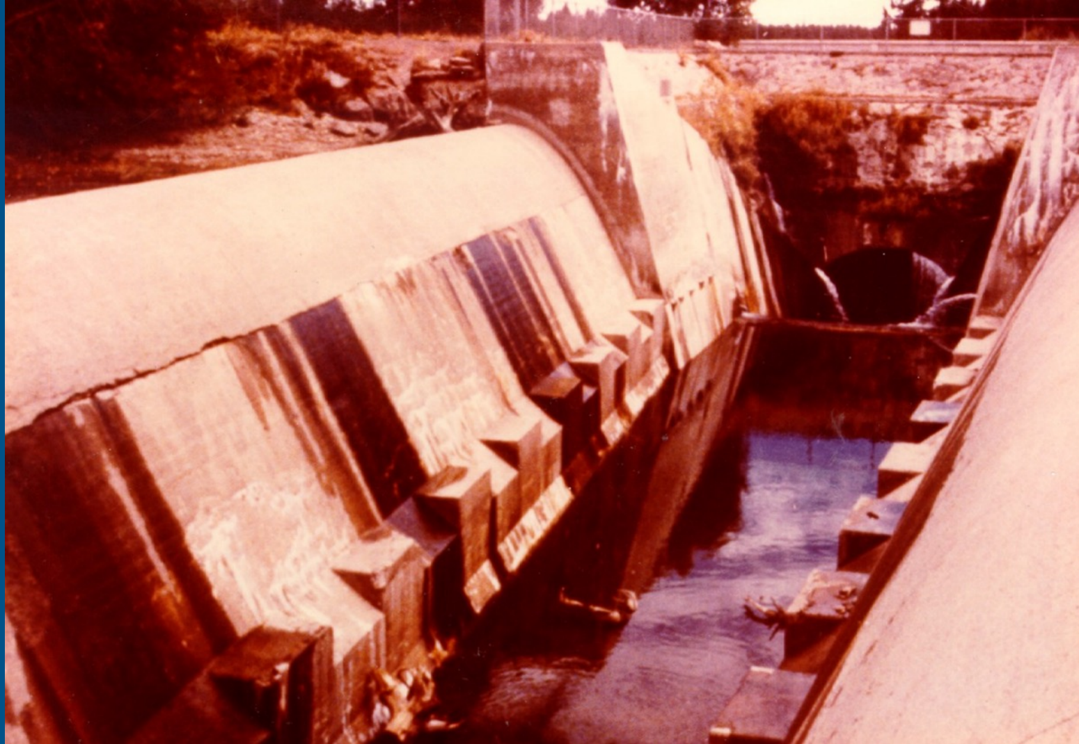
Island Park Dam, ID
