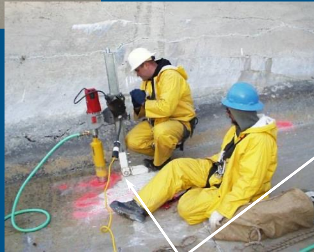
Exploration/investigation: Ground Penetrating Radar, coring, and video inspection of foundation
