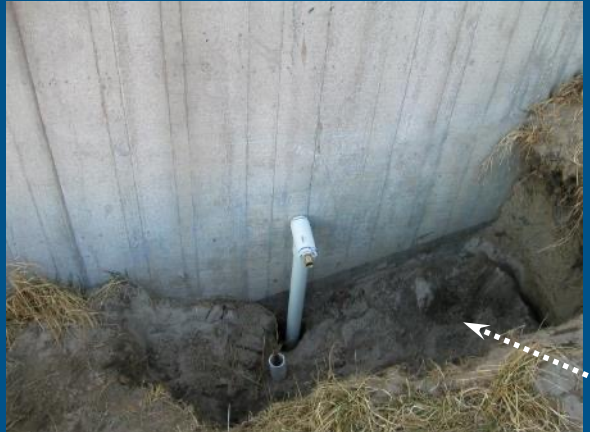
Sinkhole adjacent to outlet works control house.
