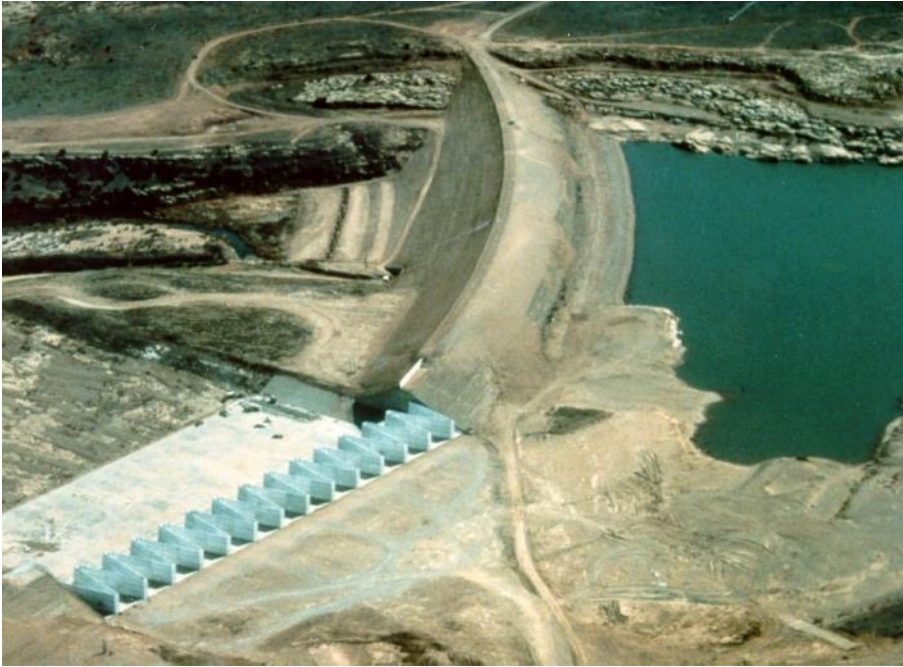
Labyrinth service spillway, Ute Dam, New Mexico
