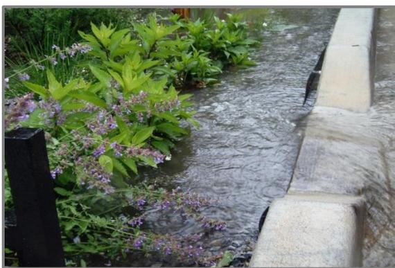
**Photo A4-3. Bioswale During a Storm Event**
