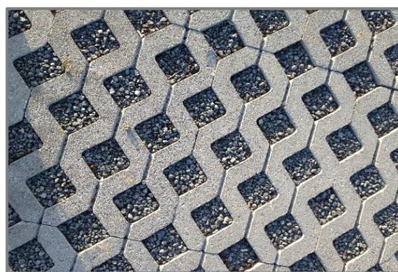
**Photo A4-2. Example of Permeable Pavement**
