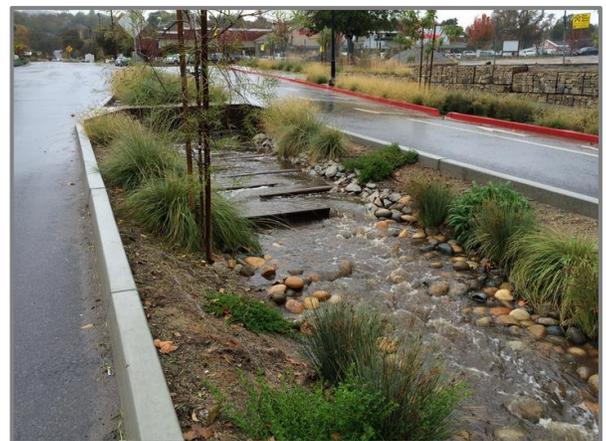
Photo 3-15. Example of Stormwater Storage during a Rainfall
