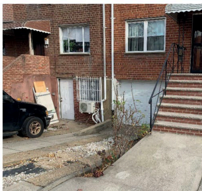
c. Driveway sloping down to converted basement
