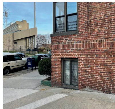
b. Basement window sill near sidewalk level
