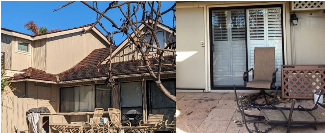
Figure 31. Examples of homes with outdoor furniture or other potentially combustibile material stored on patios and in yards.
