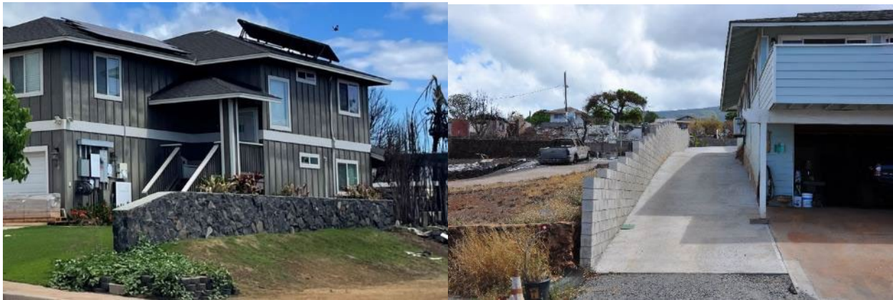
Figure 22. Homes with stone or masonry property fences that appeared to resist wildfire damage.
