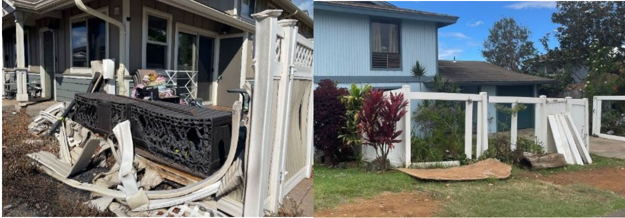
Figure 21. Residential buildings with vinyl property fences melted or warped by wind-driven wildfire.
