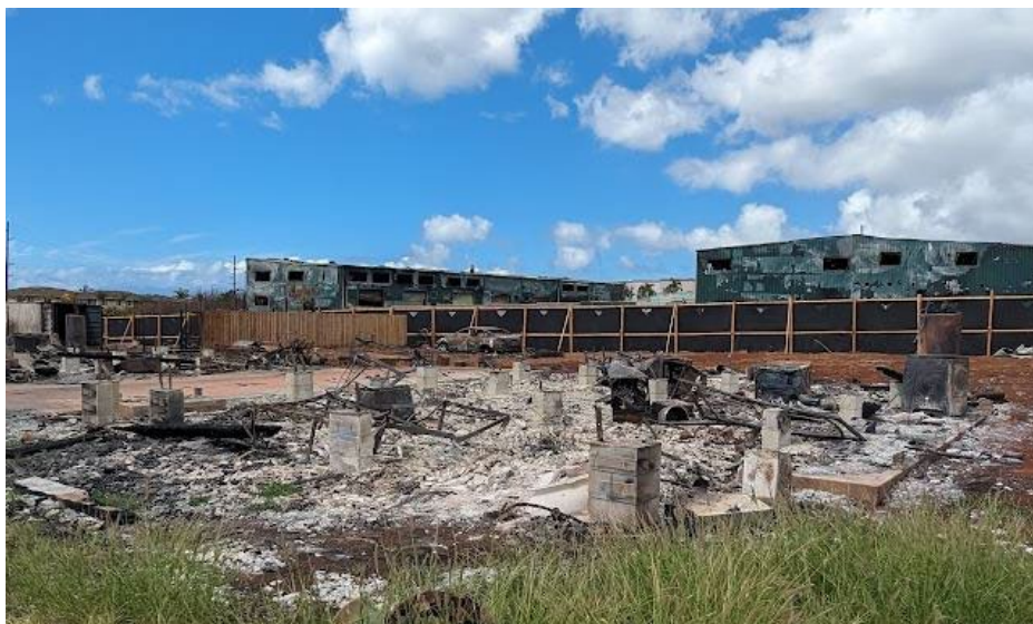
Figure 24. Home in Lahaina consumed by fire was elevated on masonry piers.
