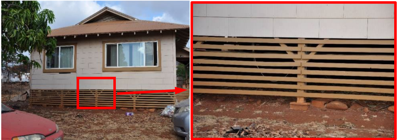
Figure 23. Maui residential building supported by post and pier foundation.
