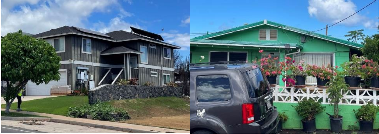
Figure 14. Wood-framed single-family residence with fiber cement siding in Lahaina (left) and painted masonry-framed single-family residence in Lahaina (right).
