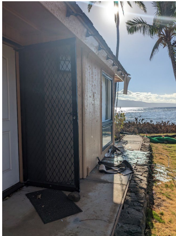
Figure 33. Concrete and stone hardscape creates a non-flammable ground cover around the perimeter of the home.
