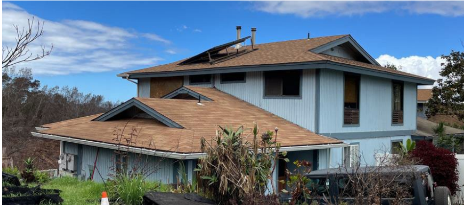
Figure 34. Example of Maui home with complex roof shape subject to debris or ember accumulation.
