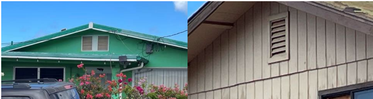
Figure 13. Examples of gable end louvred vents.
