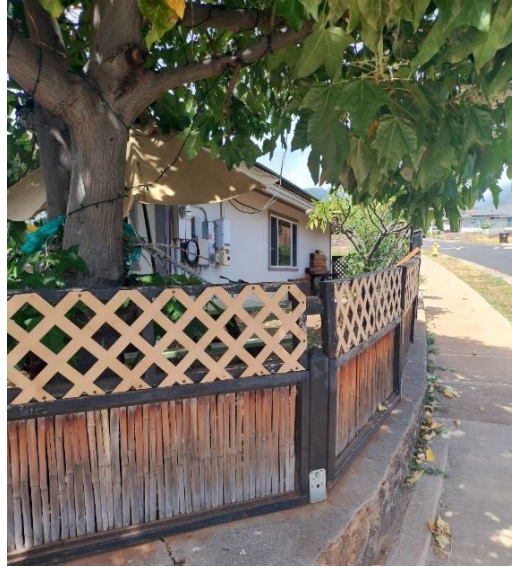
Figure 35. Maui home with lack of vegetation management from overhanging trees.
