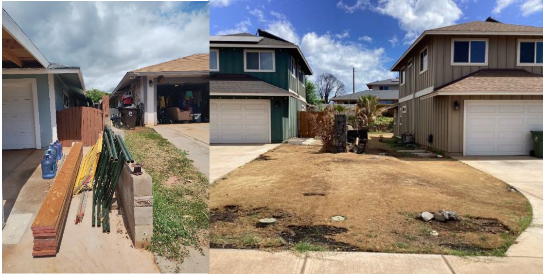
Figure 27. Examples of limited separation distances between residential buildings in Lahaina.
