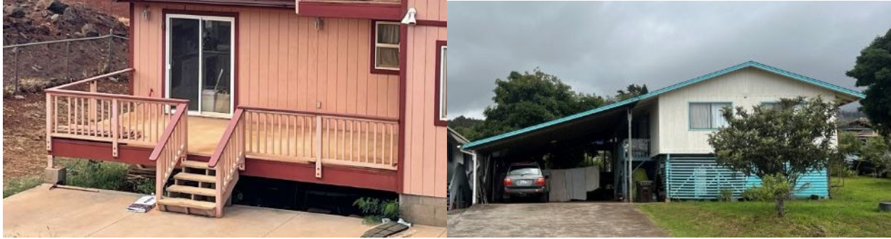
Figure 25. Elevated foundation homes with items stored underneath.
