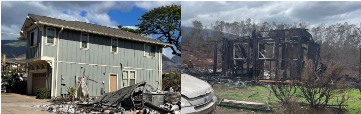
Figure 15. Comparison of residential buildings with noncombustible exterior siding (left) vs combustible exterior siding (right).
