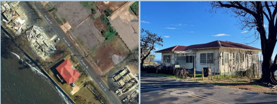
Figure 5. Aerial image of the “miracle house” (left) and a street view of the house with a metal roof that provided structural hardening and minimal landscaping that provided defensible space (right).
