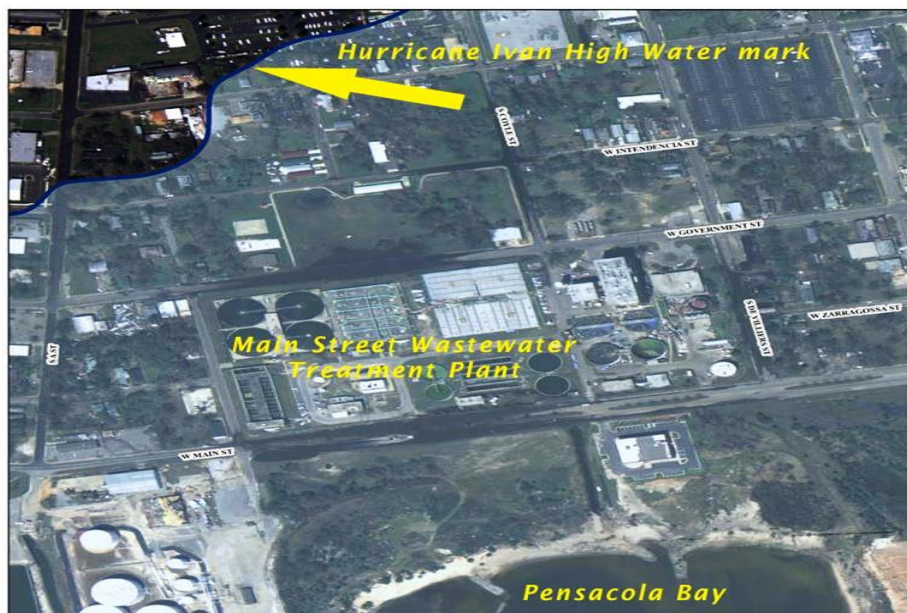
Figure 1. Storm surge from Hurricane Ivan wreaked havoc on the coastal communities of Florida's panhandle. In Pensacola, the highwater mark of the storm surge fully engulfed the Main Street Wastewater Treatment Plant in turbulent stormwaters, causing massive damage. Source: ECUA.
