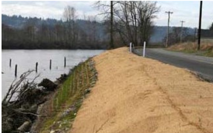
Figure 1. A photo of a soil stabilization project along a riverbank below a roadway.
