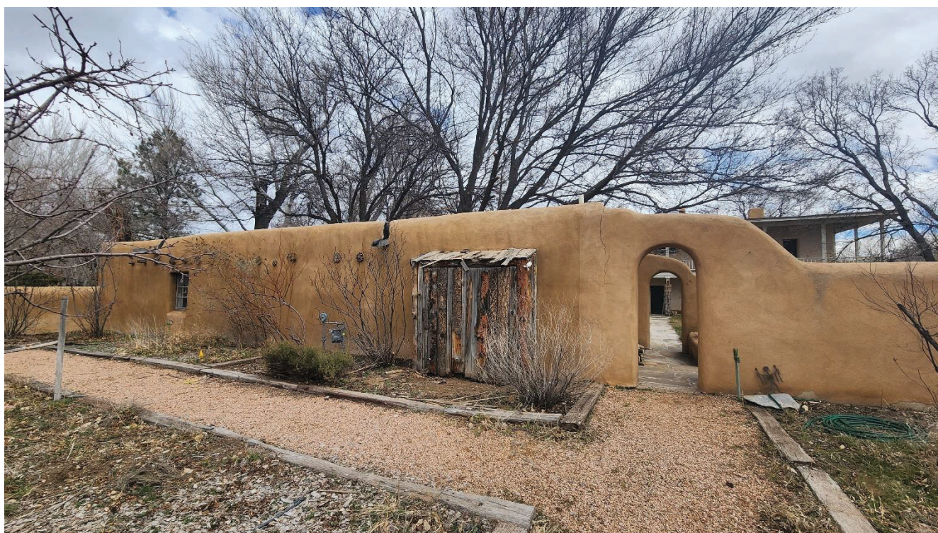
Figure 12: View east of Storehouse. Image via Applicant, 2023.
