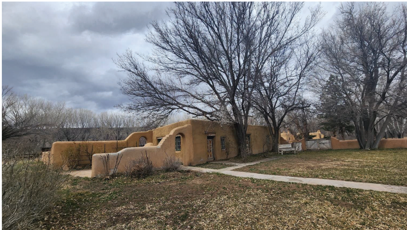
Figure 11: View northwest of Storehouse. Image via Applicant, 2023.
