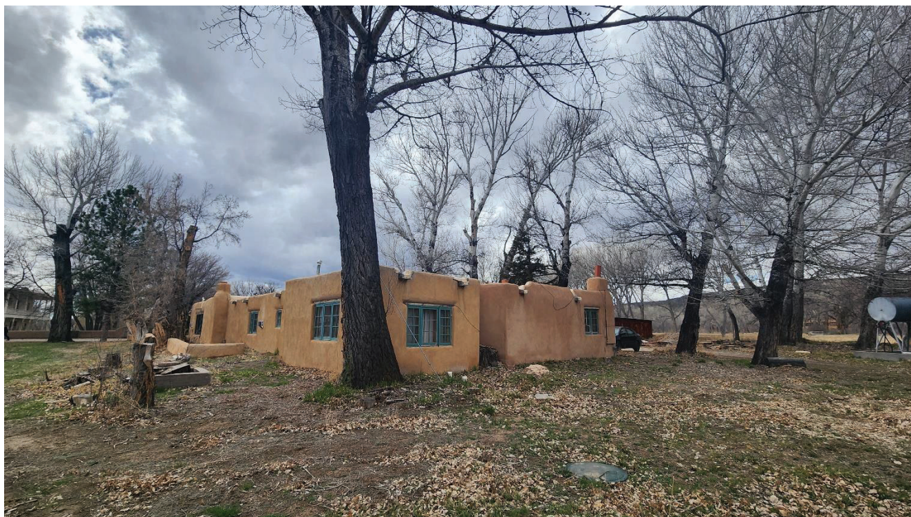
Figure 14: View southwest of Staff Housing. Image via Applicant, 2023.
