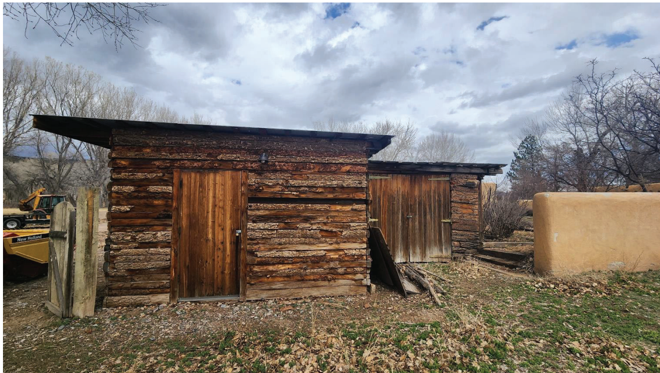
Figure 17: View north of non-contributing shed. Image via Applicant, 2023.
