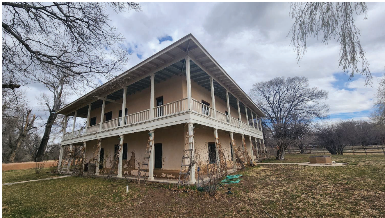
Figure 8: View northeast of Hacienda. Image via Applicant, 2023.
