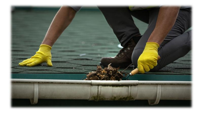
Your gutters work overtime in the winter to keep water away from your home. Failing to clean your gutters before winter can lead to clogged gutters, sagging or detached gutters, mold build-up, ice dams, and/or roof leaks.
