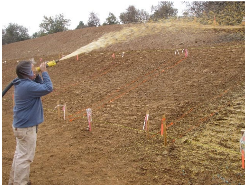
4. Hillslope Cover Application: Wet Mulch (Hydromulch)
