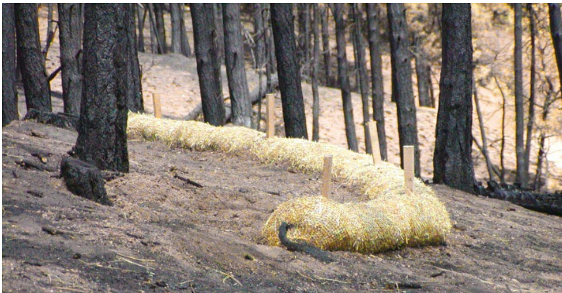
11. Barrier Application: Fiber Rolls (e.g., wattles)
