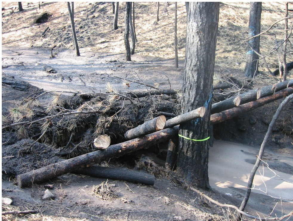
31. Road, Culvert, and Trail Flow Diversion Treatments: Debris Rack and Deflectors
