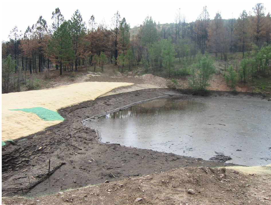
24. Channel Treatments: Debris Dams
