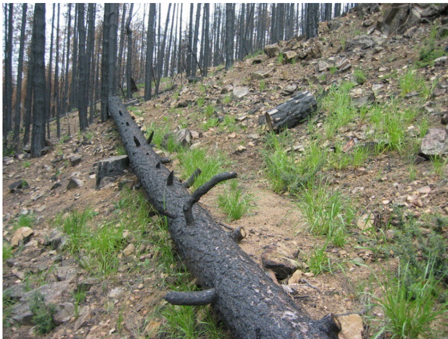
9. Hillslope Cover Application: Log Erosion Barrier
