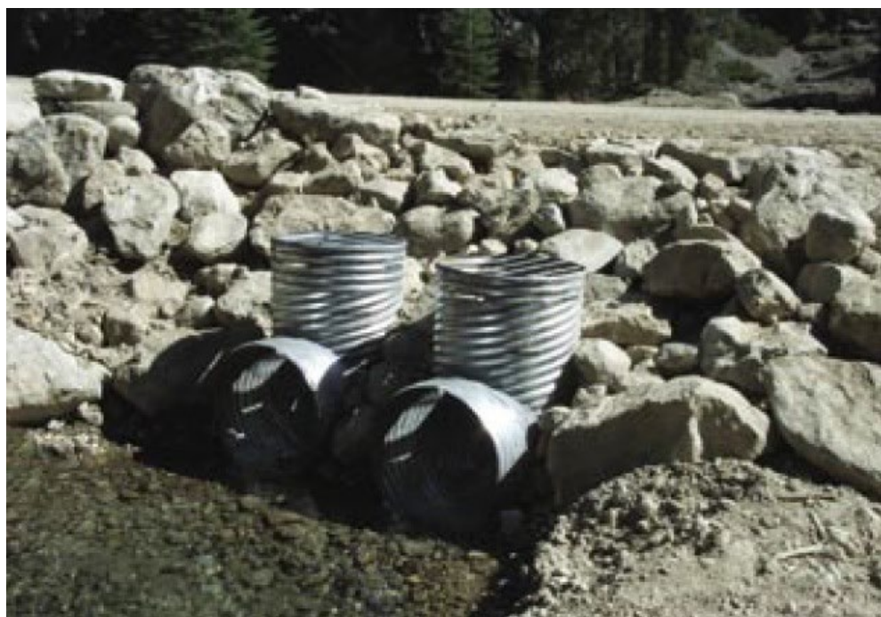
32. Road, Culvert, and Trail Flow Diversion Treatments: Riser Pipes
