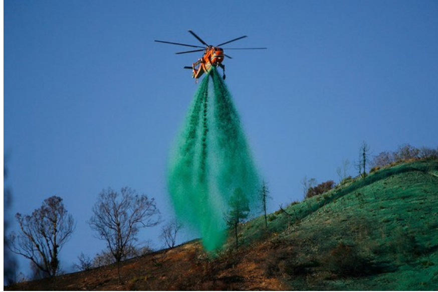
3. Hillslope Cover Application: Wet Mulch (Hydromulch)
