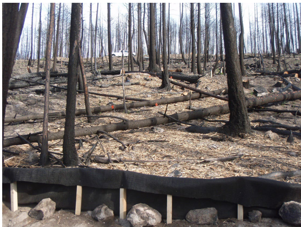
12. Barrier Application: Silt Fencing
