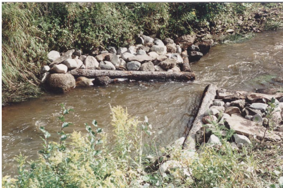
22. Channel Treatments: Flow Deflectors
