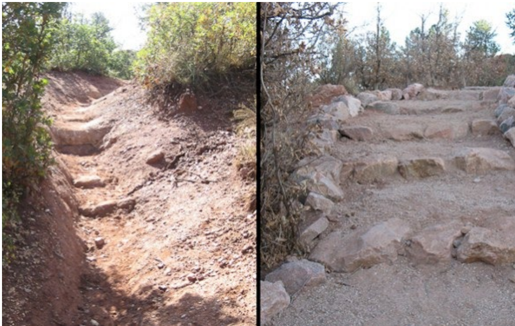
33. Road, Culvert, and Trail Flow Diversion Treatments: Trail stabilization (before/after)
