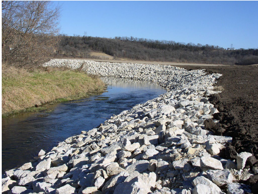
21. Channel Treatments: Bank Armoring (rip rap)
