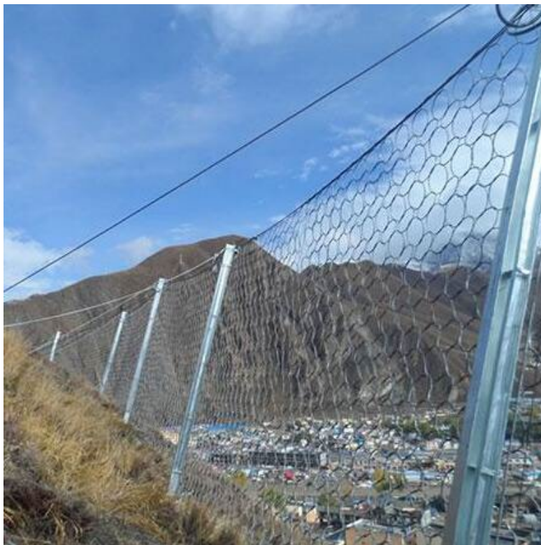
19. Channel or Hillside Treatments: Flexible Ring-Net Barriers
