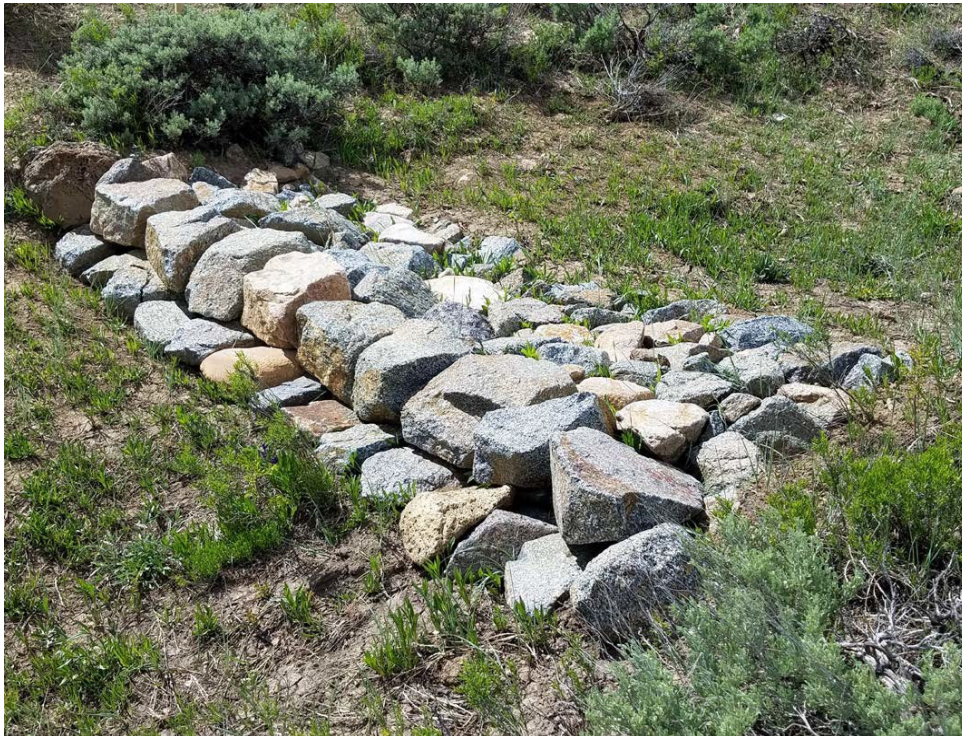
14. Channel Treatments: One Rock Dam Photo source: NRCS Conservation Practice 643 – Specification Sheet
