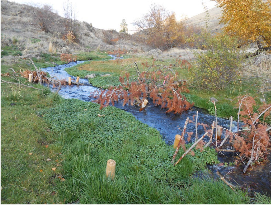
13. Channel Treatments: Post Assisted Log Structures (PALS). Photo source: Washington State Conservation Commission
