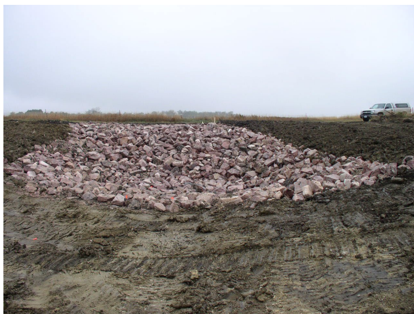
20. Channel Treatments: Grade Stabilizer
