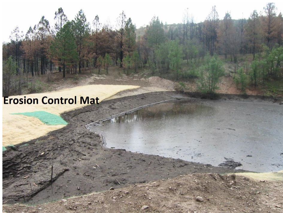
10. Barrier Application: Erosion Control Mat
