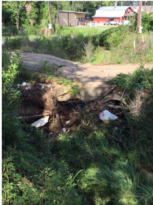
Photo 2. Proposed ROW along Hurricane Creek, facing southwest, showing two (2) existing, 36-inch-diameter culverts at Martin Luther Street to be replaced with an underground storage system consisting of two (2) 314-foot-long, 54-inch-diameter corrugated metal pipes (CMP).
