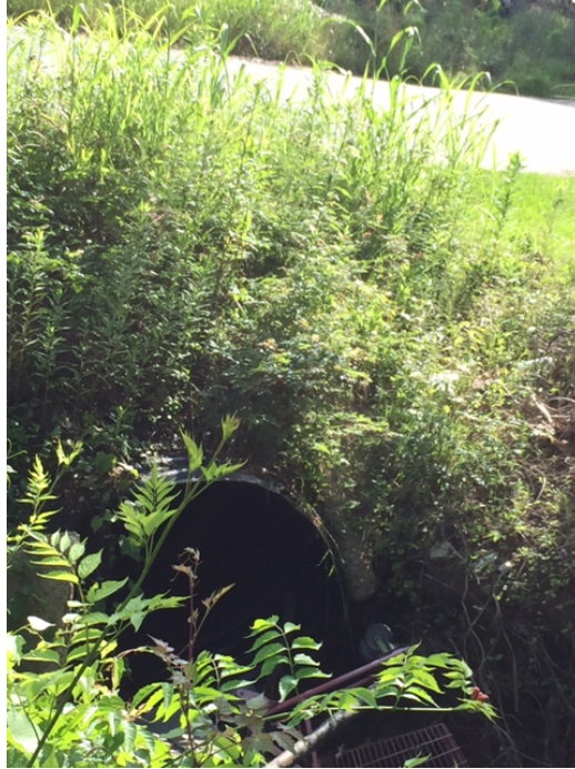
Photo 3. View of existing 54-inch diameter culvert at Martin Luther Street to be replaced with a single, underground storm drain system consisting of two (2) 314-foot-long, 54-inch-diameter CMP).
