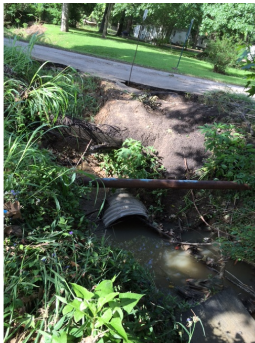
Photo 4. View of existing 48-inch culvert on Hurricane Creek at Garsee Road, facing southwest, to be replaced with a 46-foot-long, 60-inch-diameter CMP.
