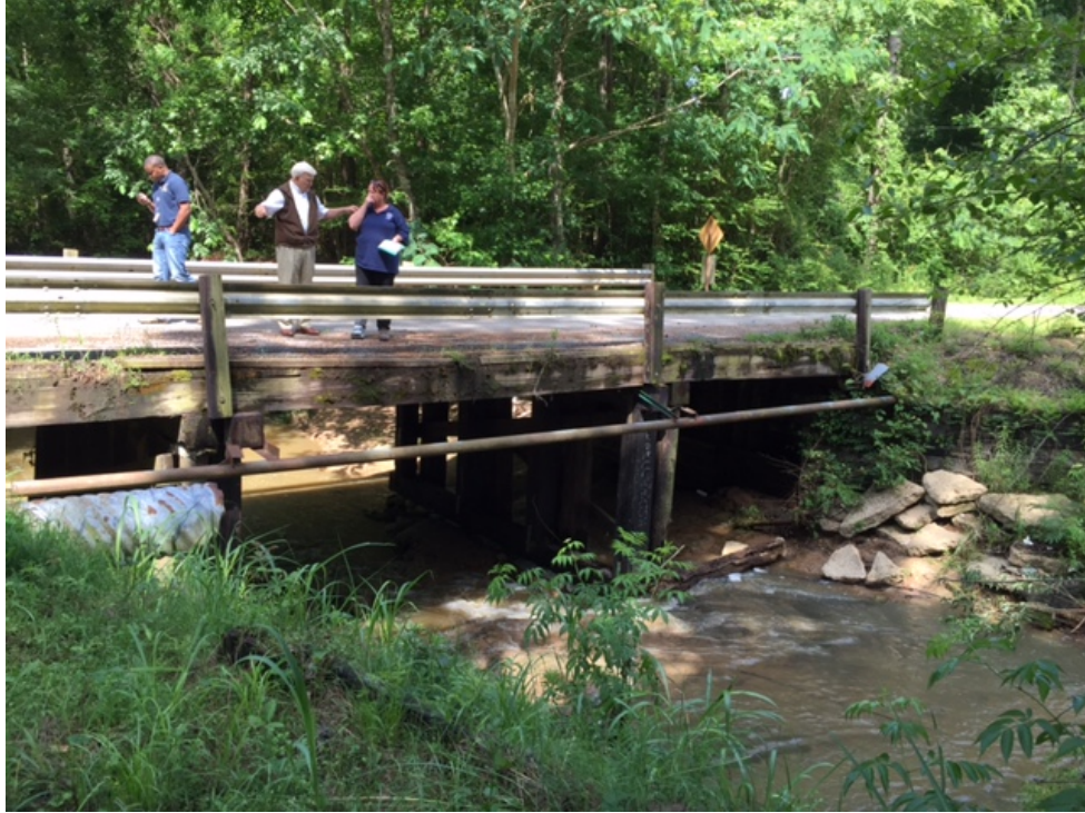
Photo 11. Existing bridge over Hurricane Creek on Central Street to be replaced with a new railroad flat car bridge.
