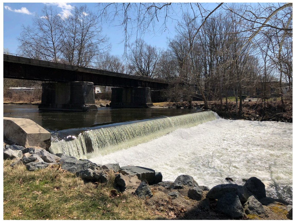
Lower E.R. Collins Dam
