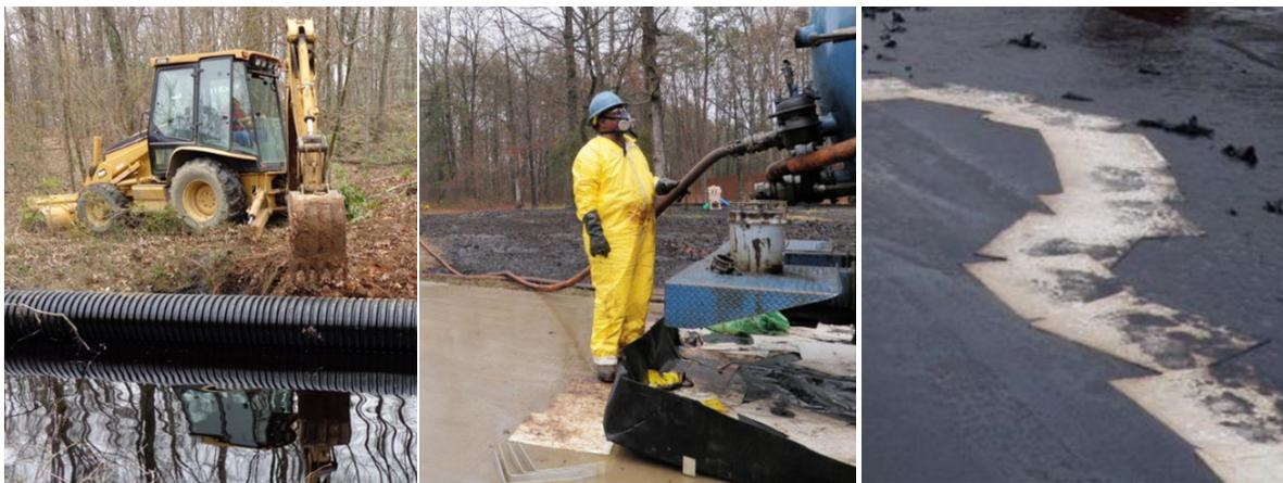
**Figure 50: Damming, vacuuming, and sorption for contamination control following a surface spill**
