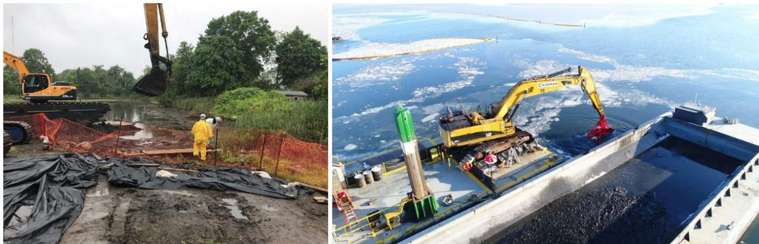
**Figure 70: Remediation of polychlorinated biphenyl (PCB)-contaminated soils and sediments in New Bedford Harbor**
