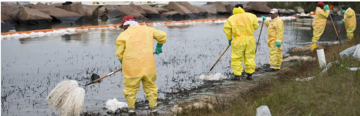
**Figure 1: PPE-clad responders cleaning an oil spill with pom-poms and rakes**
