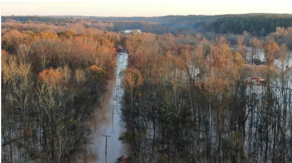
Figure 4: The access road to the pump station is completely submerged for several thousand feet during flood events.
