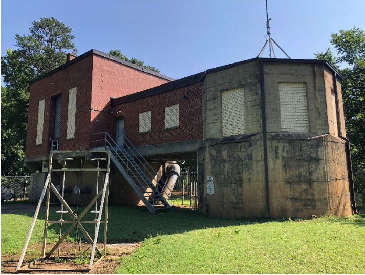
Figure 3: Existing pump station building during a flood event and during normal conditions.
