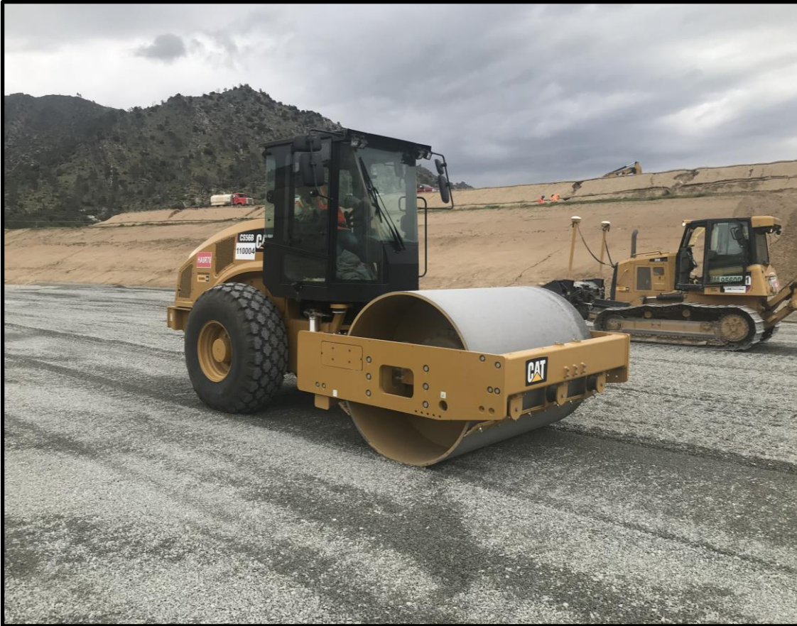
Vibratory Compactor for Coarse-Grained Granular Materials in Embankment Zones Such as Dam Shells, Filter, and Drainage Zones [Thinner Lifts]
