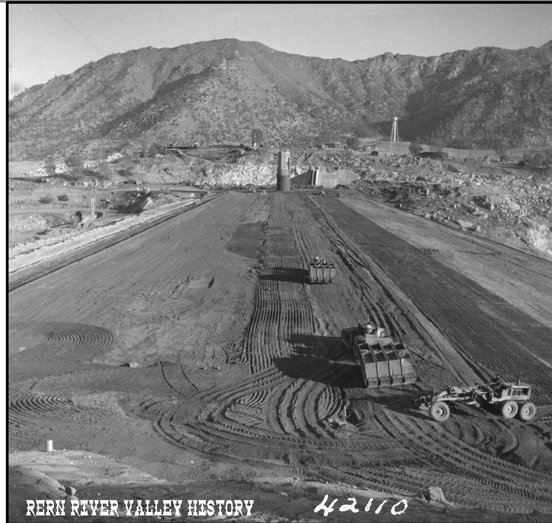
Example: Lake Isabella Dam Original Construction
