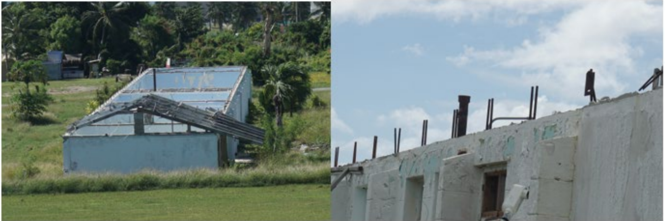
Figure 10: Home on Tinian that used informal roof-to-wall connections. The residential building lost the roof framing during high winds. The roof-to-wall connectors failed to secure the roof framing to the top of the wall.
