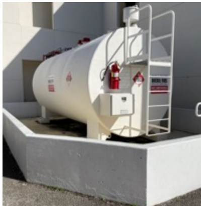
Figure 6. Examples of well-maintained generator fuel tank and pump systems.
