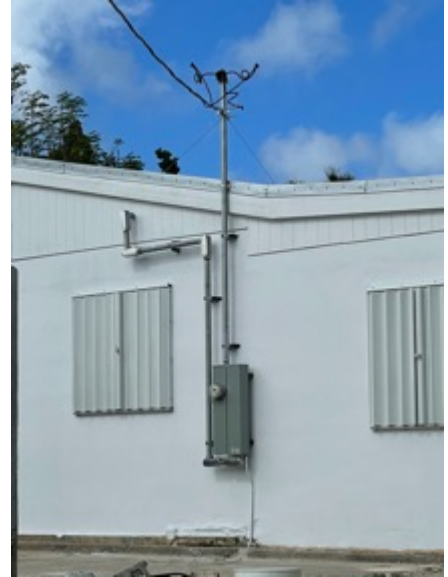
Figure 4. Properly secured service mast attached to renovated building.
