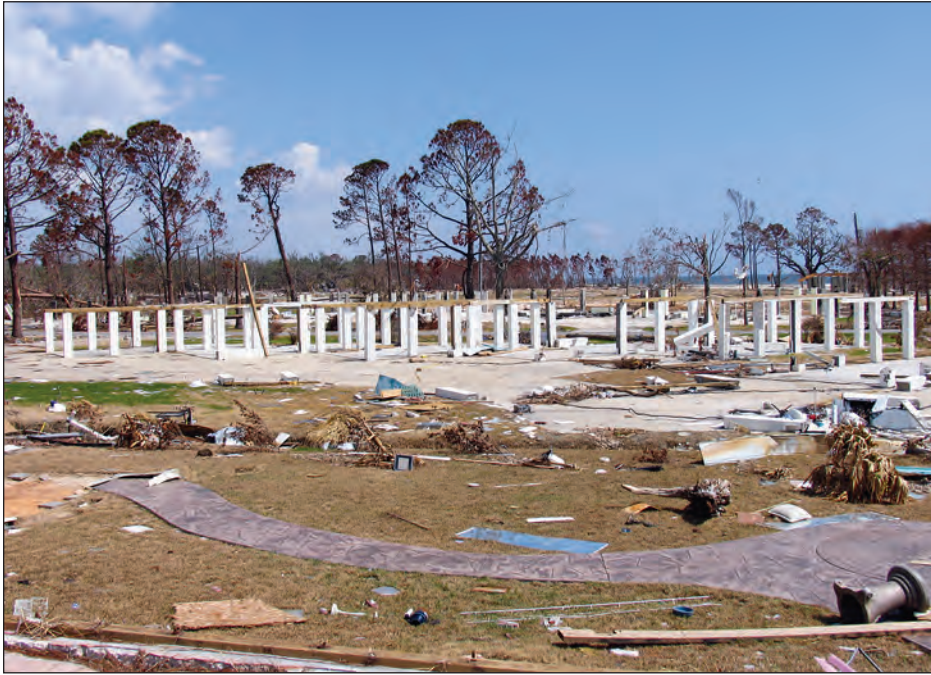
Figure 4-25. Another typical example of building failures when surge and waves exceeded pier foundation height (Long Beach, Mississippi)
