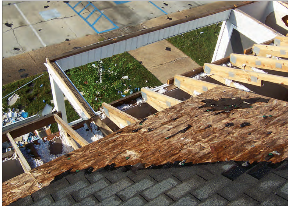
Figure 4-97. Another example of metal connectors lacking on the gabled roof that once existed over the entrance (estimated wind speed: 130 mph. inland Long Beach, Mississippi)
