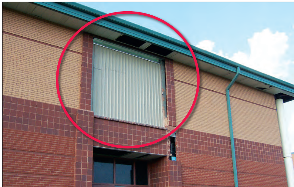
Figure 3-58. Window failed due to wind pressures, resulting in water entry into the building and damage to ceiling boards. After the failure, metal panels were installed for temporary protection (circled) (Gulfport, Mississippi).
