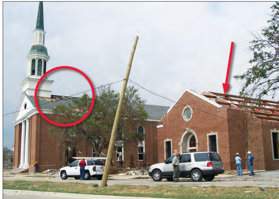
Figure 4-117. Gulfport First Presbyterian Church with wind damaged roofs. Note the wind damaged roof covering (circle) and the missing roof decking (arrow) (estimated wind speed: 130 mph. Gulfport, Mississippi).
