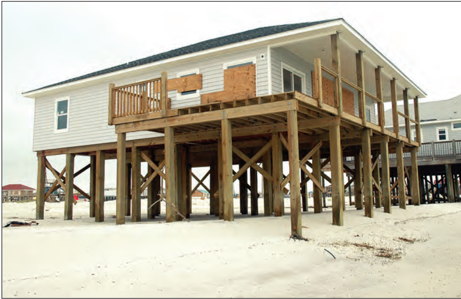
Figure 4-3. Successful example of well-elevated and embedded pile foundation following Katrina (Dauphin Island, Alabama)
