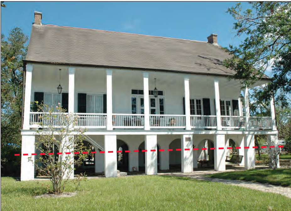
Figure 4-23. This 100-year-old building is on the National Register of Historic Places. It sustained minimal flood damage due to elevation on taller piers (an architectural choice, not a requirement when the building was constructed in 1905). Note the estimated flood depth in relation to the first floor (red line) (Mandeville, Louisiana).
