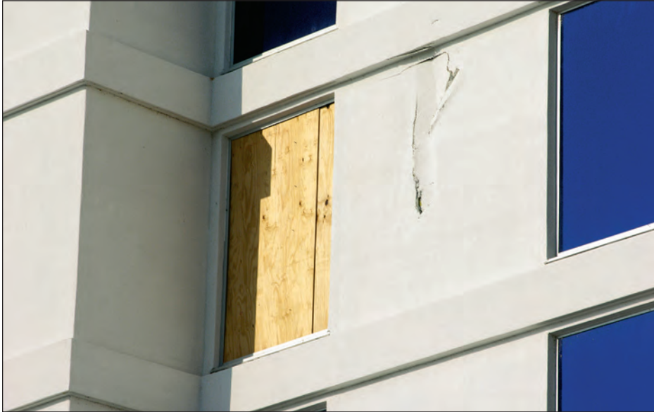
Figure 3-46. Closeup of high-rise building whose structure performed well, but experienced widespread damage to its EIFS envelope and some glazing damage (Biloxi, Mississippi)
