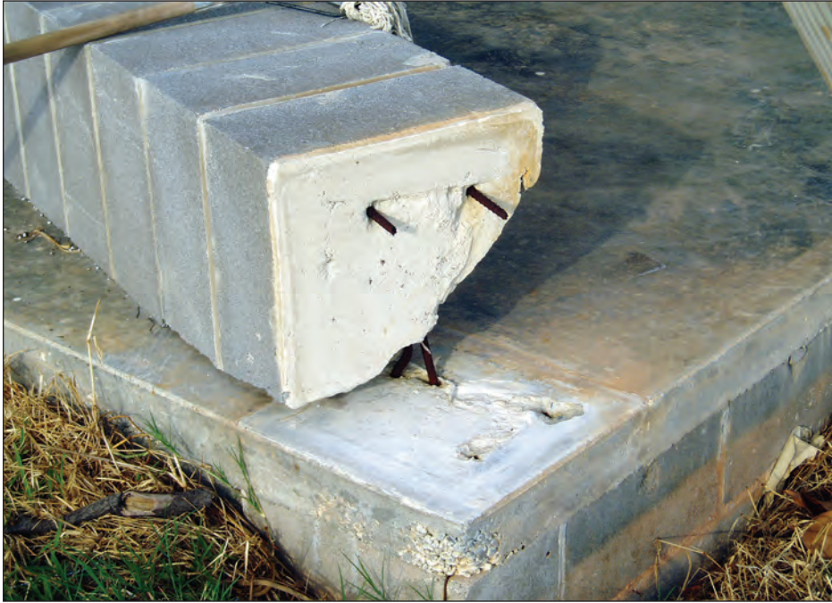
Figure 4-28. Pier connection failure (Belle Fontaine Point, Jackson County, Mississippi)
