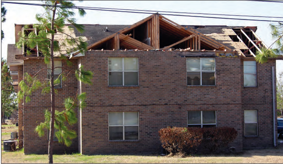
Figure 3-42. Gable end wall and roof sheathing loss to apartments near the City of Toca (St. Bernard Parish, Louisiana)
