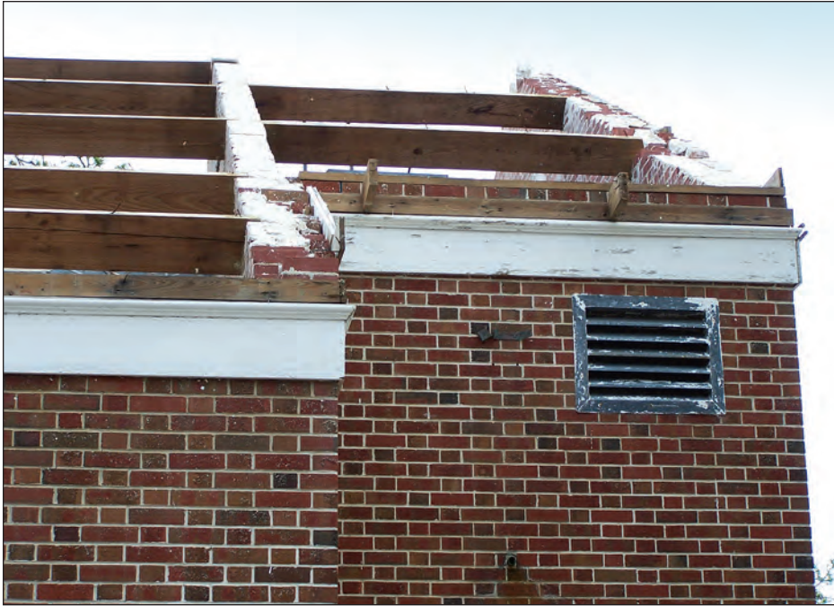
Figure 4-118. Grouted multi-wythe masonry walls. Note loss of roof decking (estimated wind speed: 130 mph. Gulfport, Mississippi).
