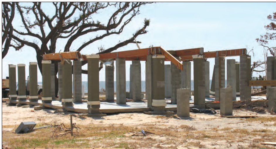
Figure 3-6. Elevated house atop masonry pier foundation was lost, probably due to waves and storm surge reaching above the top of the foundation (Long Beach, Mississippi)
