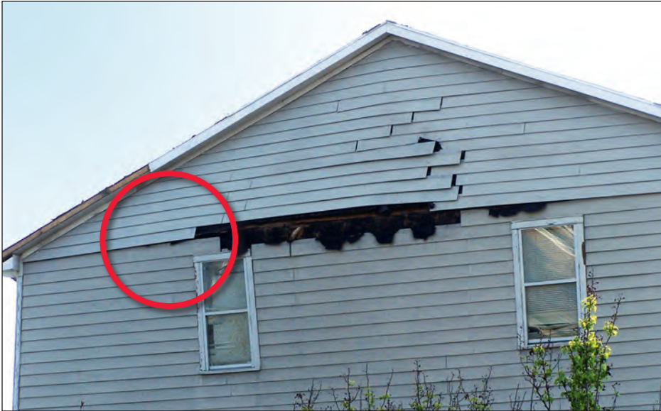
Figure 4-73. Hinge formed between gable end and top of wall (hinge circled) (estimated wind speed: 120 mph. Ocean Springs, Mississippi)
