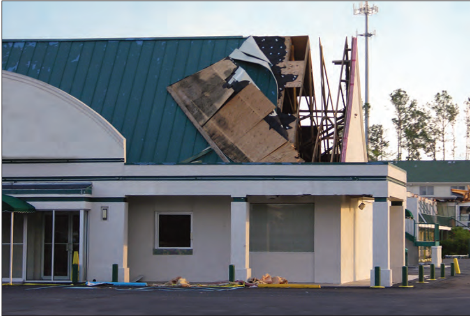
Figure 4-108. Roof uplift failure in wood-framed commercial building (estimated wind speed: 115 mph. Slidell, Louisiana)
