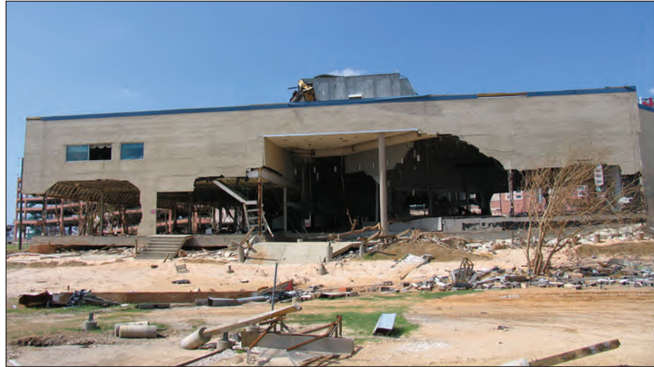
Figure 3-20. Marine Education Center, which lost most of its walls due to wave action, storm surge, and floating debris (Biloxi, Mississippi)
