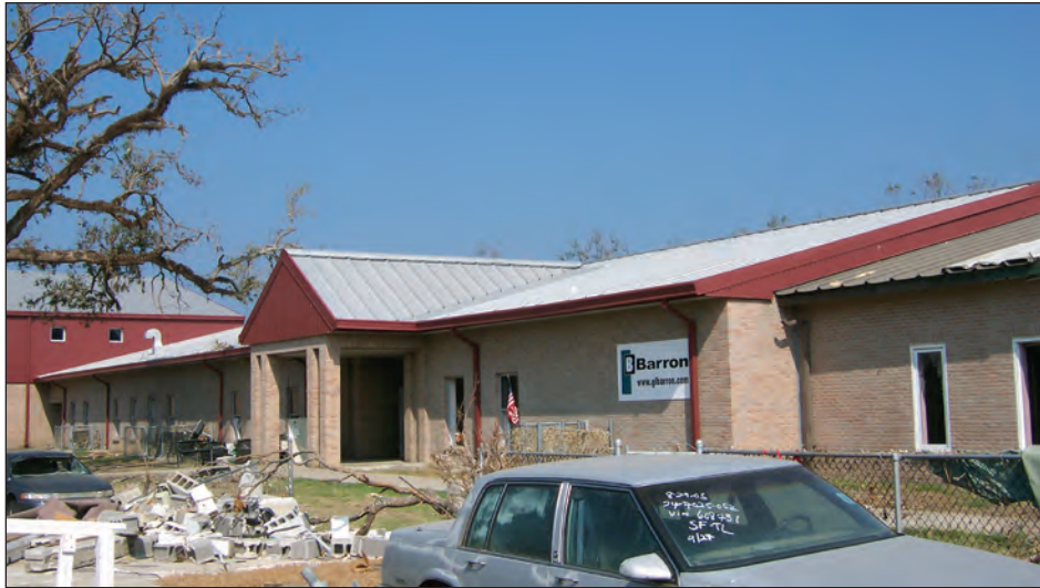
Figure 4-120. Undamaged newer PEMB constructed in 2001 (estimated wind speed: 130 mph. Pass Christian, Mississippi)
