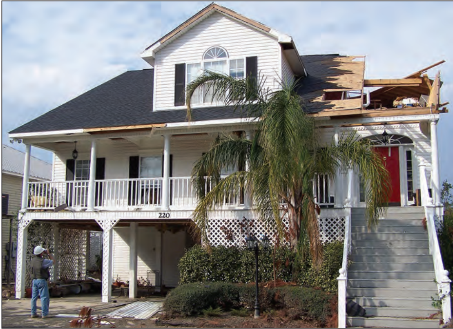
Figure 3-32. Relatively new home damaged from internal pressurization and lack of adequate connections (Pass Christian, Mississippi)
