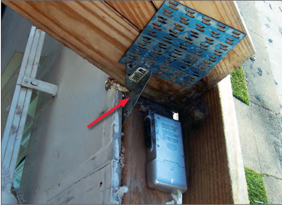
Figure 4-95. Metal connectors (arrow) were used on main trusses (estimated wind speed: 130 mph. inland Long Beach, Mississippi).
