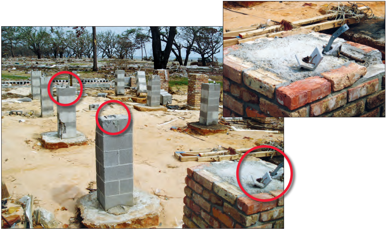
Figure 4-31. Failure of pier-to-beam connections due to wave and flood forces acting on the elevated building (Long Beach, Mississippi)
