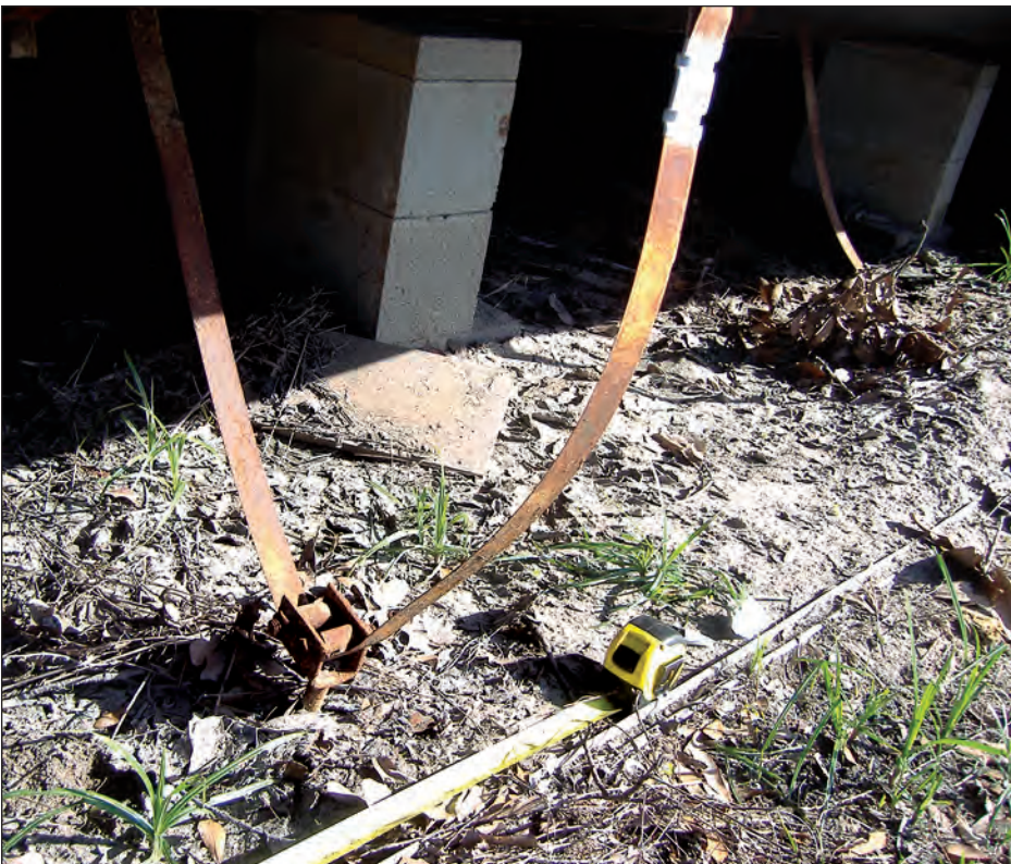
Figure 4-48. Foundation of home shown in Figure 4-47. The flood level rose above the floor, the ground anchors were apparently pulled up from the saturated soil, and the piers were displaced (St. Bernard Parish, Louisiana).
