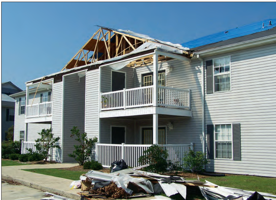
Figure 4-78. Pressurization of the second floor porch ceiling of this apartment led to soffit failure and loss of roof decking and other structural components (estimated wind speed: 120 mph. Ocean Springs, Mississippi).
