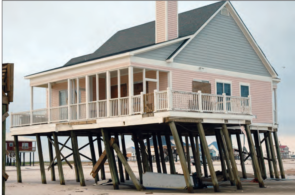
Figure 3-5. House on verge of collapse due to shallow embedment of timber pile foundation (Dauphin Island, Alabama)
