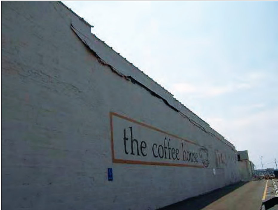
Figure 4-114. Unreinforced masonry parapet failure on a building located in Exposure C (estimated wind speed: 130 mph. Gulfport, Mississippi)
