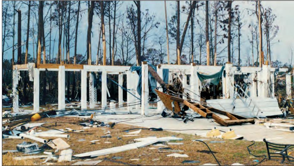
Figure 4-10. Failure at connections between pile foundations and buildings (Pass Christian, Mississippi)
