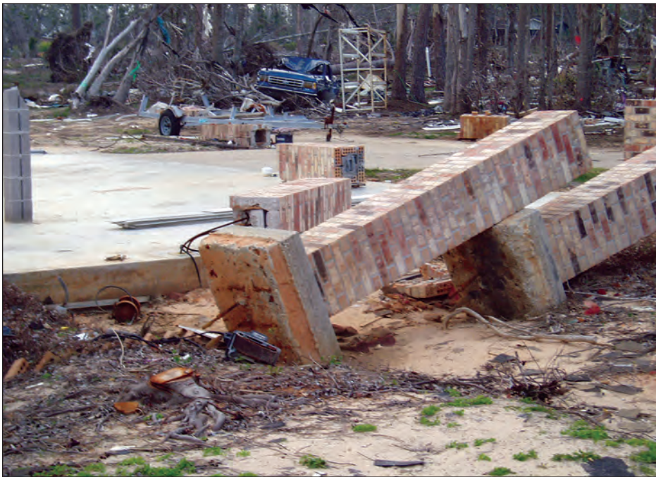
Figure 4-26. Failure of masonry piers on shallow footings (Pass Christian, Mississippi)
