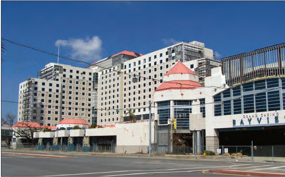
Figure 4-111. East tower located in Exposure C under construction with reinforced concrete and post-tensioned floor slabs. The east tower was water-inundated on the first floor and suffered only minor wind damage to the roof covering of the finished tower (estimated wind speed: 120 mph. Biloxi, Mississippi).
