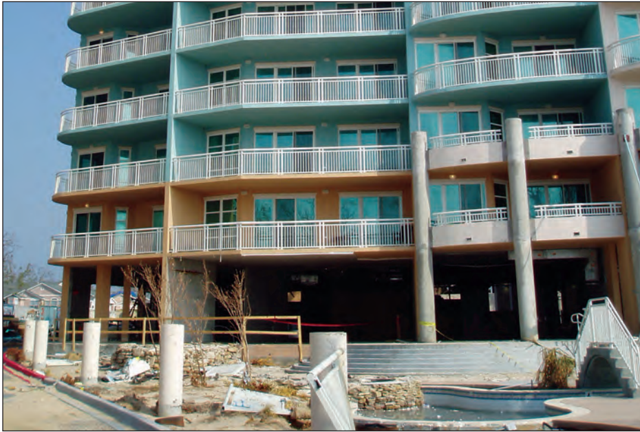
Figure 3-18. Waves and storm surge washed through the lowest floor of this condominium building, but the building reportedly sustained no structural damage (Gulfport, Mississippi).
