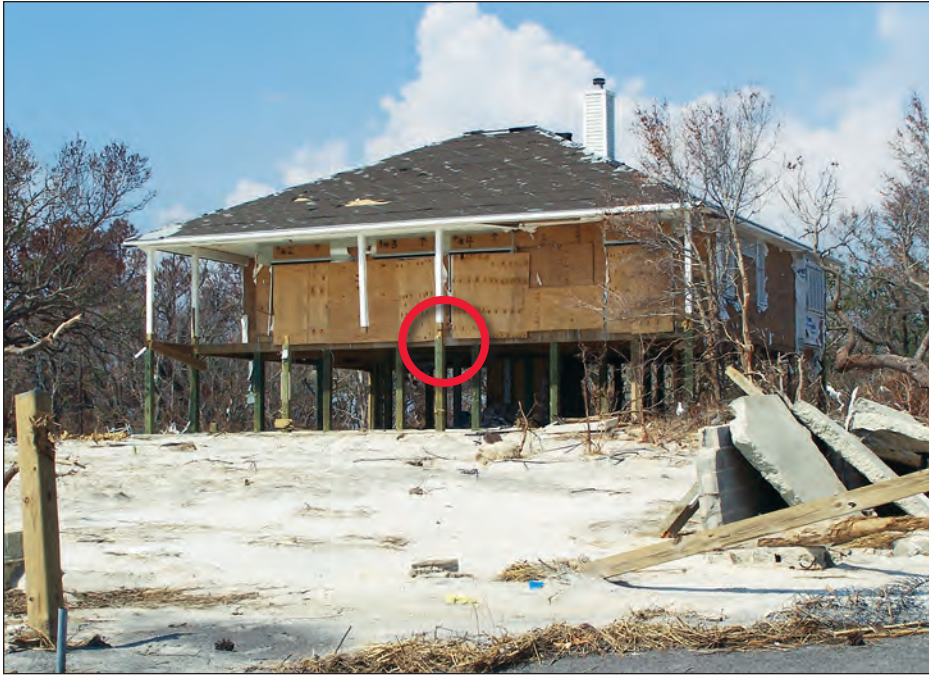
Figure 4-80. Coastal home located in Exposure C received significant surge damage into the habitable level and, although it lost its porch and three porch columns, the basic load path remained connected. Red circle indicates location of Figure 4-81 (estimated wind speed: 120 mph. Ocean Springs, Mississippi).
