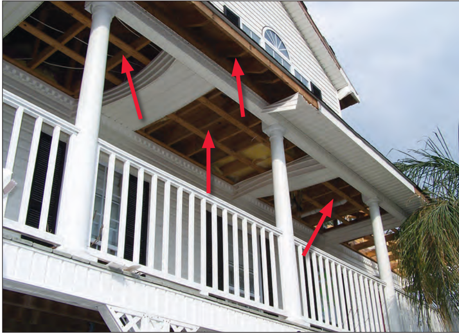
Figure 4-77. High pressures under overhangs often lead to progressive structural failures. Note the vinyl soffit material removed by high-wind pressures (arrows) (estimated wind speed: 130 mph. Pass Christian, Mississippi).
