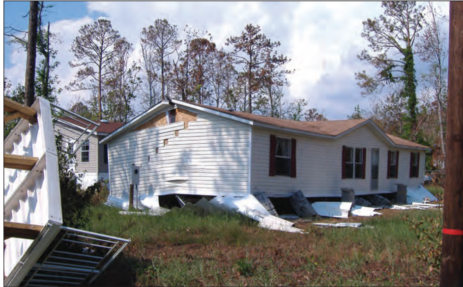
Figure 3-12. Manufactured home washed off its supports by moving floodwaters (Ocean Springs, Mississippi)
