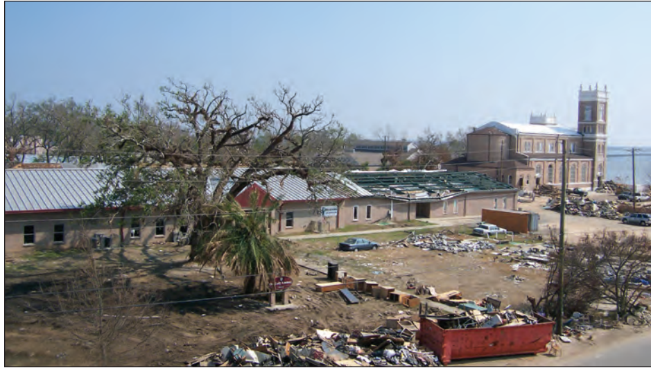
Figure 4-119. Relative performance of older and newer PEMBs located in Exposure C. The 5-year old building on the left was not damaged by winds; the 30-year old building (estimated) on the right lost its roof (estimated wind speed: 130 mph. Pass Christian, Mississippi).
