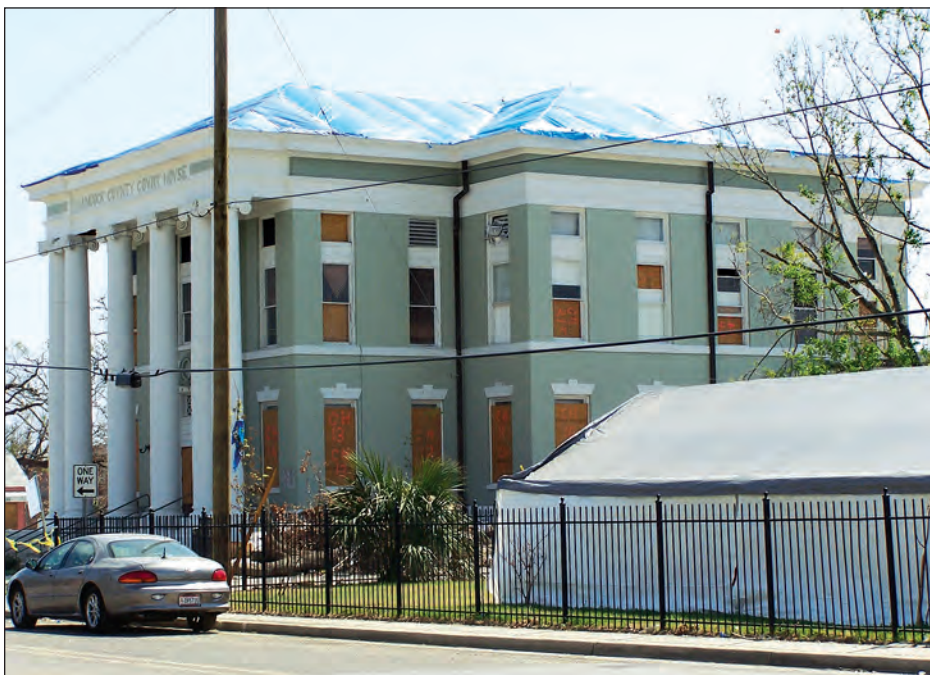
Figure 4-115. Hancock County Courthouse located in Exposure C with roof and windows damaged by wind and windborne debris (estimated wind speed: 125 mph. Bay St. Louis, Mississippi)
