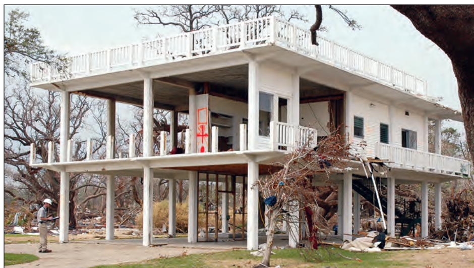
Figure 4-19. Another surviving house constructed with a reinforced concrete frame. The wave elevation was approximately 2 to 3 feet above the elevated floor (Long Beach, Mississippi).
