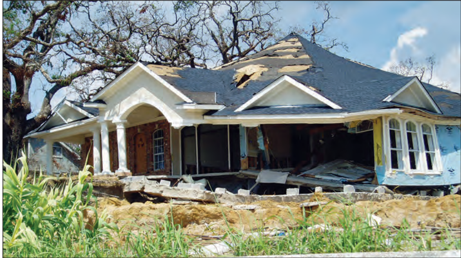
Figure 4-39. Shallow foundation failure due to localized scour and damage to walls by surge and wave impacts (Ocean Springs, Mississippi)
