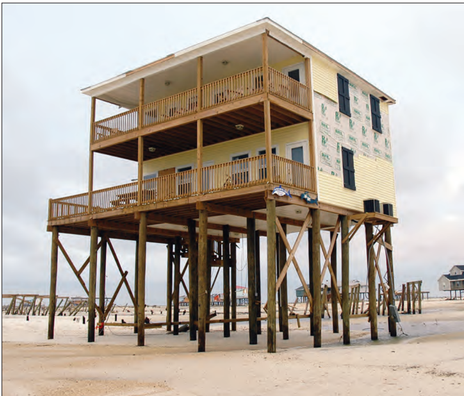
Figure 4-4. Another successful example of well-elevated and embedded pile foundation following Katrina. Note adjacent building failures where foundations were not high enough or where pile embedment was inadequate (Dauphin Island, Alabama).
