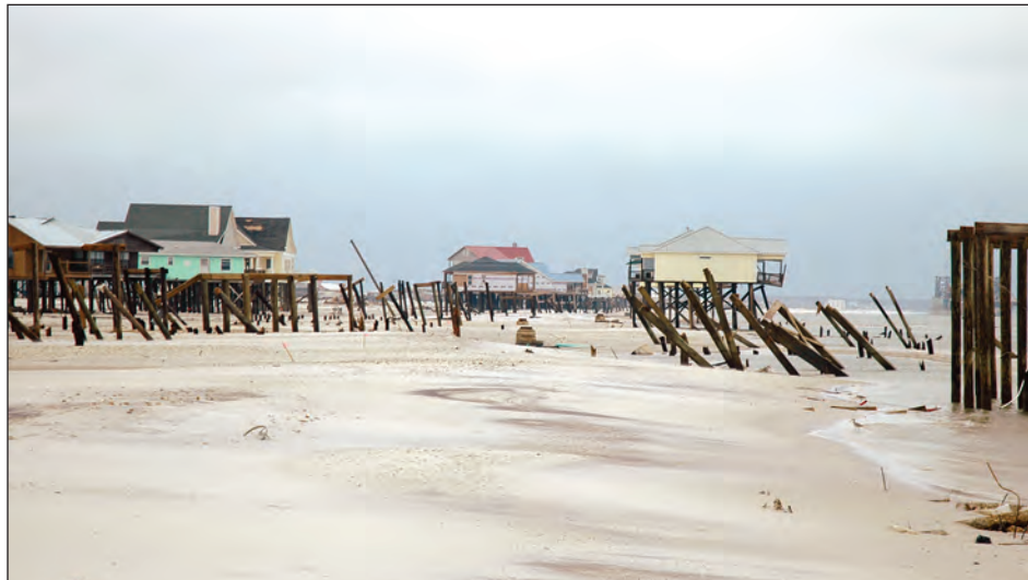
Figure 4-6. Leaning piles indicate building failures due to shallow embedment (Dauphin Island, Alabama).
