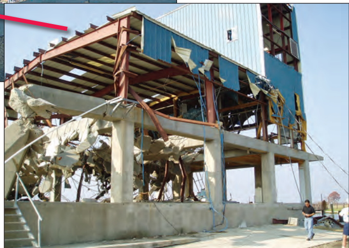
Figure 3-21. A reinforced concrete and pre-engineered metal building (PEMB) housing a seafood processing building sustained severe damage due to storm surge, waves, and floating debris. Nearby marina buildings were also destroyed (Lakeshore area, Hancock County, Mississippi).
