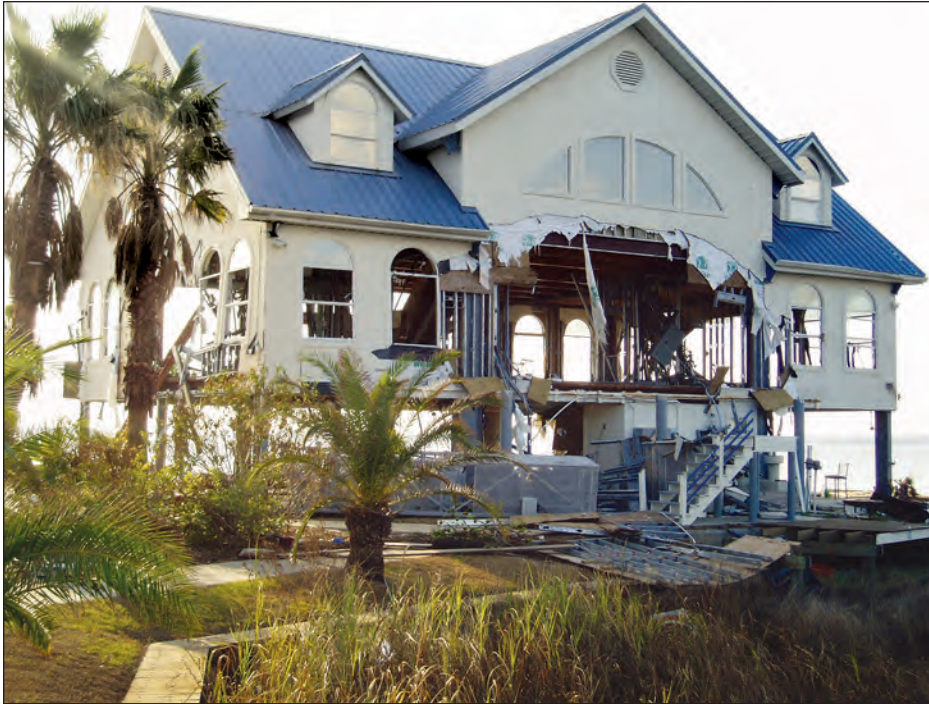
Figure 4-15. Steel-framed building on St. Louis Bay survived storm surge and wave action above the elevated floor level (Pass Christian, Mississippi)
