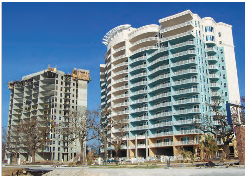
Figure 4-67. High-rise building along Beach Boulevard received non-structural flood damage to lower floors, but no apparent flood or wind damage to higher residential floors (Gulfport, Mississippi)
