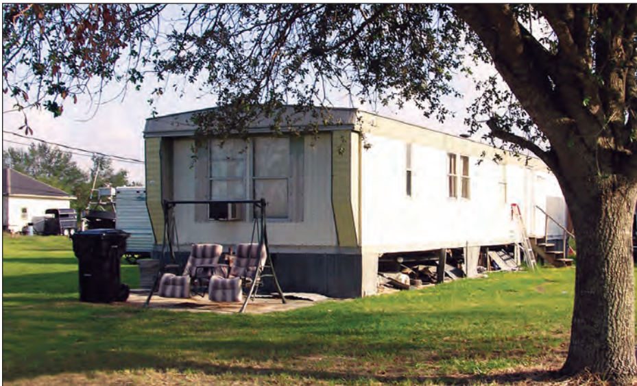
Figure 4-104. Manufactured home located in Exposure C installed with ground anchors (estimated wind speed: 110 mph. Plaquemines Parish, Louisiana)
