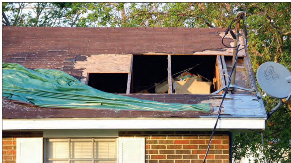
Figure 3-36. Roof sheathing damage to an older home (Gulfport, Mississippi)
