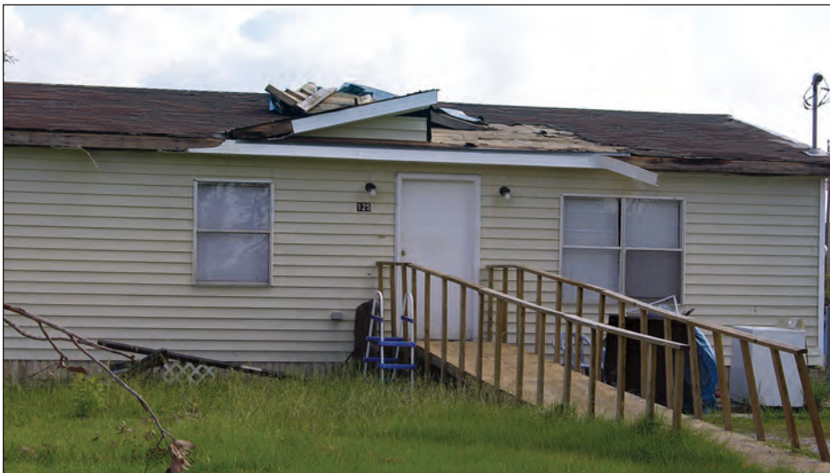
Figure 3-38. Manufactured home lost a gable roof over its entrance, asphalt shingles, and metal fascia along its eaves (Plaquemines Parish, Louisiana)
