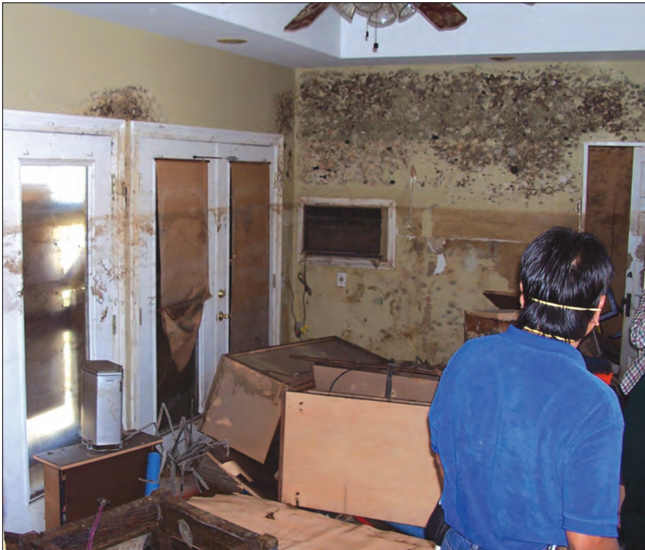
Figure 3-9. Interior damage and mold from prolonged flooding (New Orleans, Louisiana)
