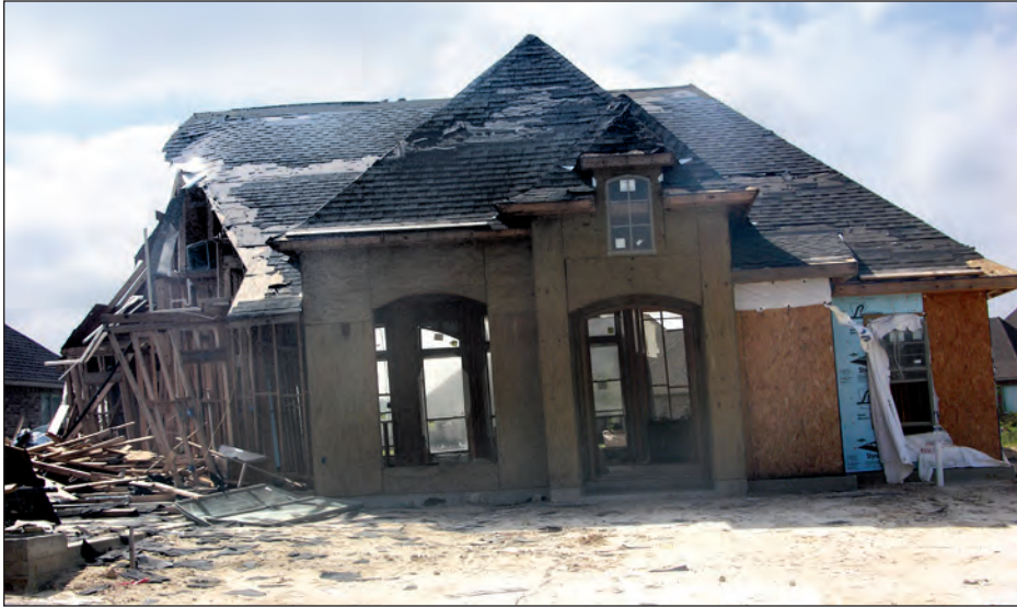
Figure 3-37. A home under construction racked severely when exposed to Katrina's winds. Its attached garage also collapsed (Slidell, Louisiana).
