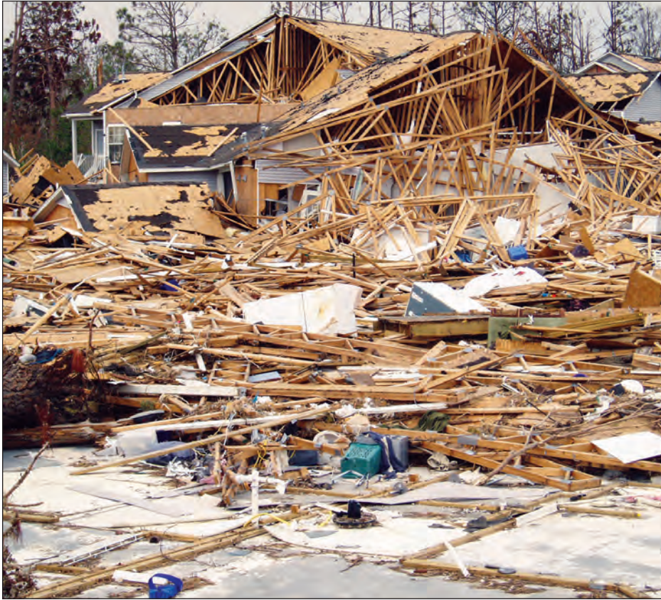
Figure 3-14. Apartments on slab foundations destroyed by waves, storm surge, and wind (Long Beach, Mississippi)
