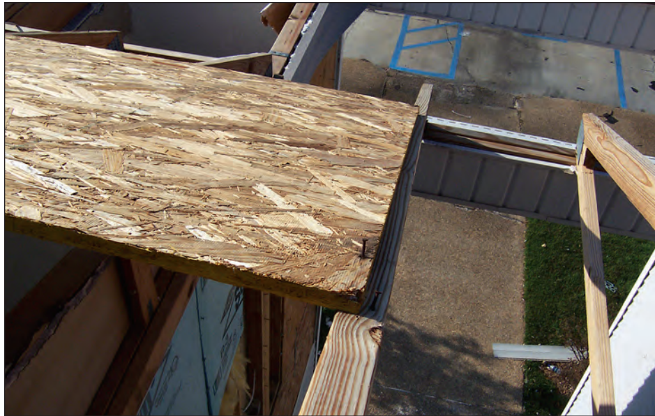
Figure 4-94. Roof sheathing attachment was inadequate. Several staples were missing, some staples missed framing, and inland the sheathing pulled over the staples (estimated wind speed: 130 mph. Long Beach, Mississippi).
