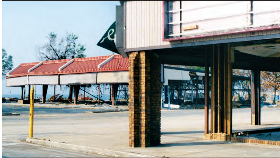
Figure 4-55. Steel-framed strip mall construction with exterior and interior wave damage (Gulfport, Mississippi)
