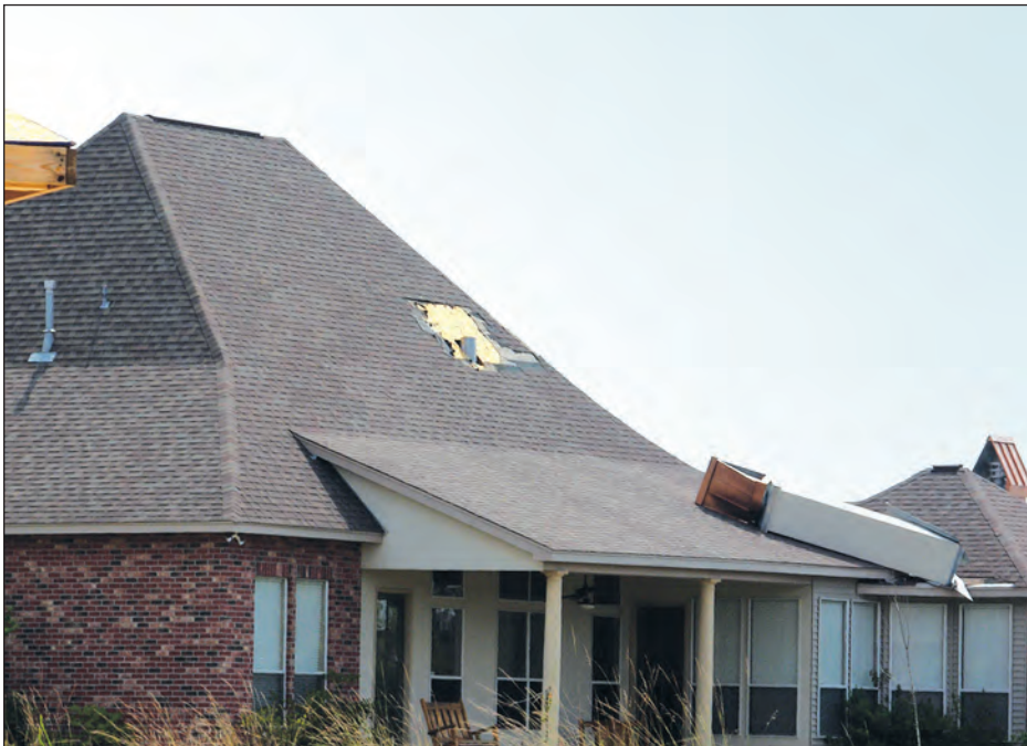
Figure 3-33. Loss of shingles and chimney failure caused by inadequate attachment (Slidell, Louisiana)
