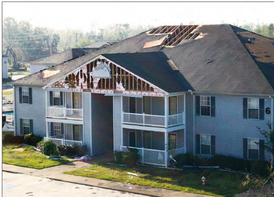
Figure 4-98. Apartment building's gable walls sheathed with insulation failed during Katrina (estimated wind speed: 130 mph. inland Long Beach, Mississippi)
