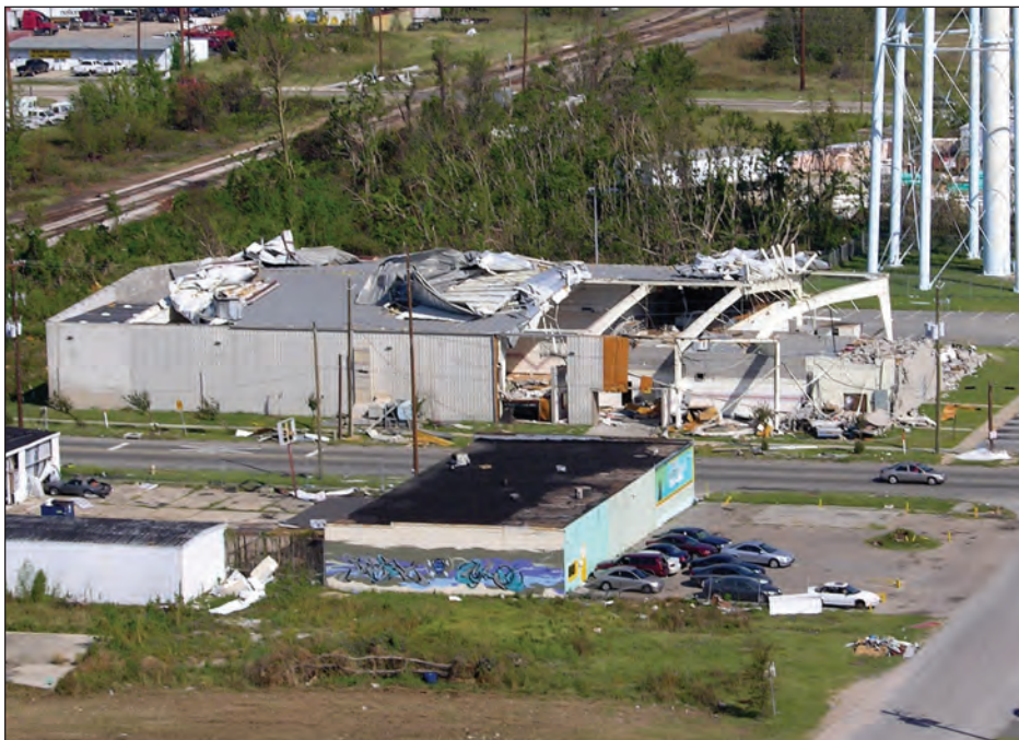
Figure 4-122. Failure of older (1974) pre-engineered metal building (estimated wind speed: 130 mph. Gulfport, Mississippi)
