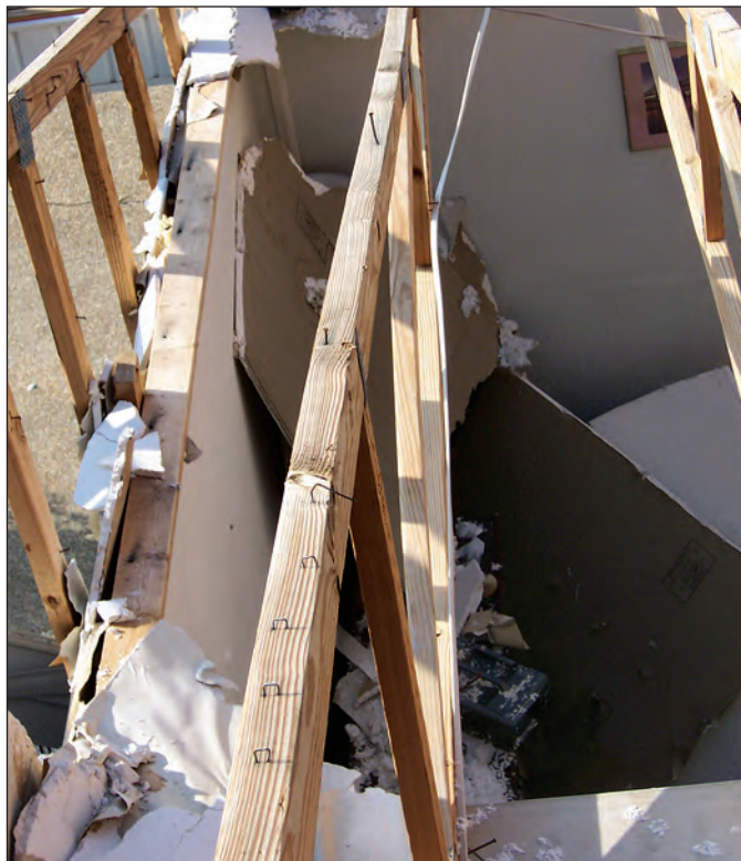
Figure 4-94. Roof sheathing attachment was inadequate. Several staples were missing, some staples missed framing, and inland the sheathing pulled over the staples (estimated wind speed: 130 mph. Long Beach, Mississippi).
