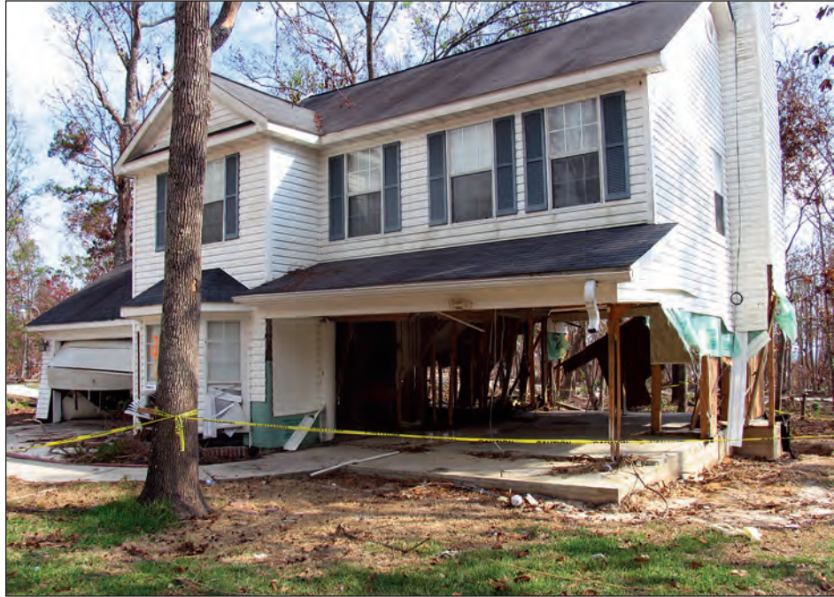
Figure 4-36. Wave and surge damage to a house supported by load-bearing wood-frame walls atop a slab foundation. The house was approximately 1/4 mile from the Gulf, in mapped flood Zone C (1992 FIRM), and was probably exposed to Coastal A Zone conditions (3-4 feet stillwater depth and small waves) during Katrina (Pointe Aux Chenes area, Jackson County, Mississippi).
