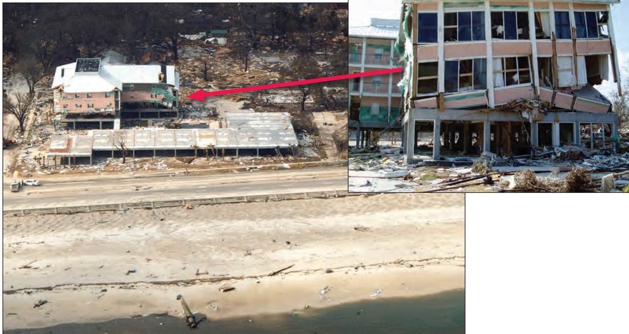
Figure 3-17. Wave and surge damage to Gulf-front apartments. Note the poured concrete foundation columns and slab performed well, but the waves rose above the slab and attacked the wood-framed buildings, destroying the building closest to the Gulf, and severely damaging the landward building. The severity of damage to the remaining building resulted in demolition (Biloxi, Mississippi).
