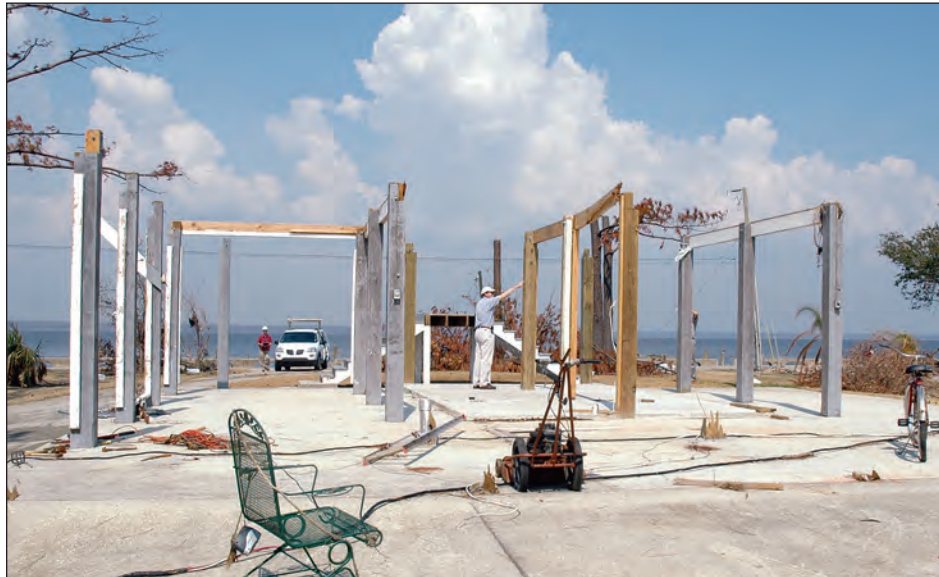
Figure 4-11. Pile and connection failure (Bay St. Louis, Mississippi)
