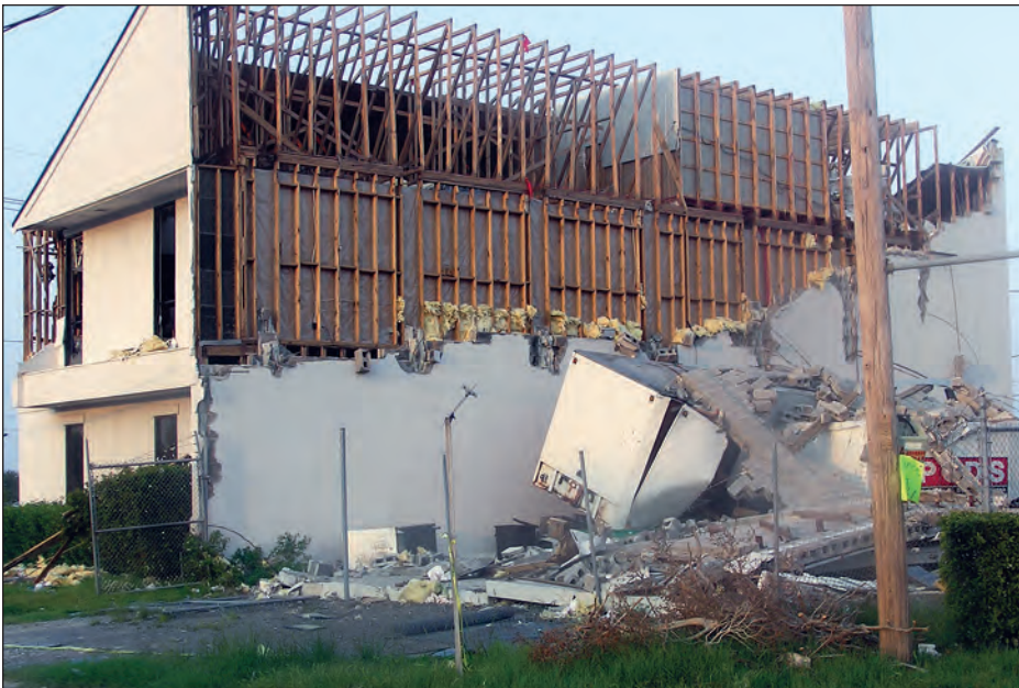
Figure 4-109. Three-story wood-framed commercial building lost roof sheathing and the exterior wall collapsed (estimated wind speed: 105 mph. New Orleans, Louisiana)
