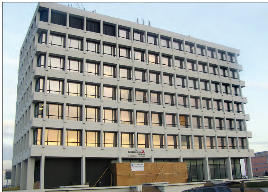
Figure 4-60. Concrete-framed building sustained non-structural damage to lower portions from storm surge (Gulfport, Mississippi)
