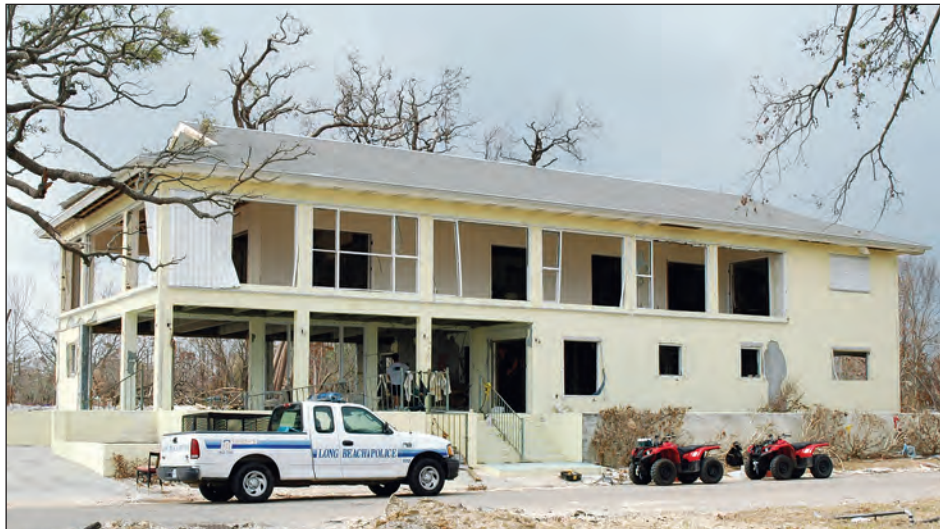
Figure 4-18. Surviving house constructed with a reinforced concrete frame and walls. Note storm shutters on upper level damaged by waves (Long Beach, Mississippi).
