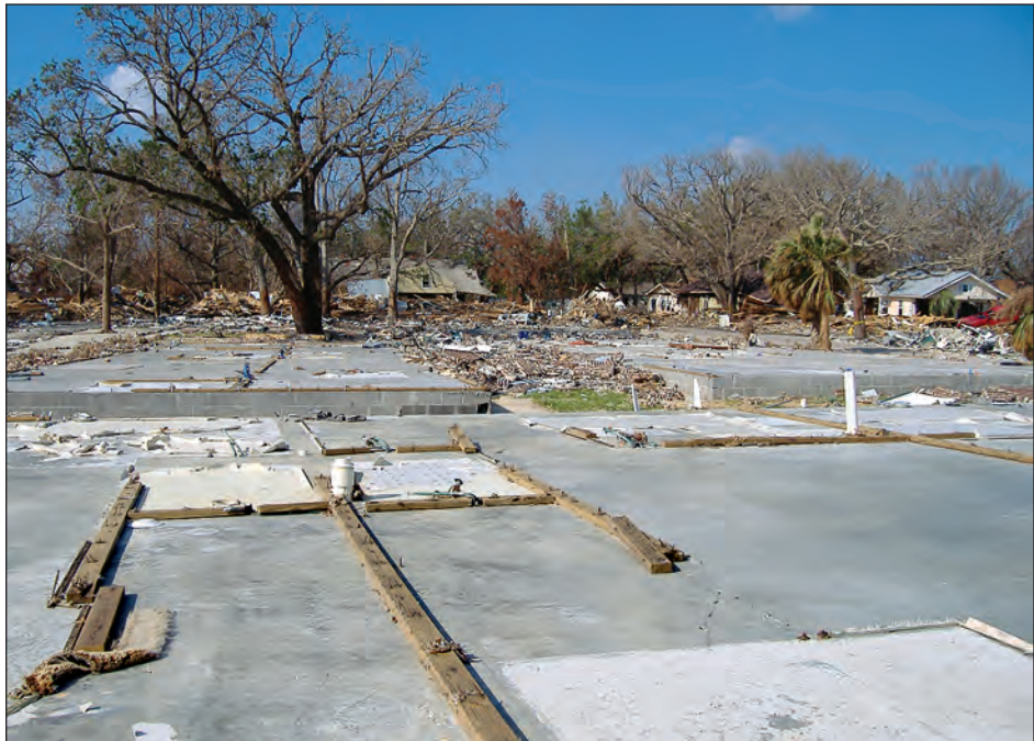
Figure 4-37. Waves, surge, and floating debris destroyed many single-family homes on slab foundations. Note debris from houses washed landward into other buildings (Biloxi, Mississippi).
