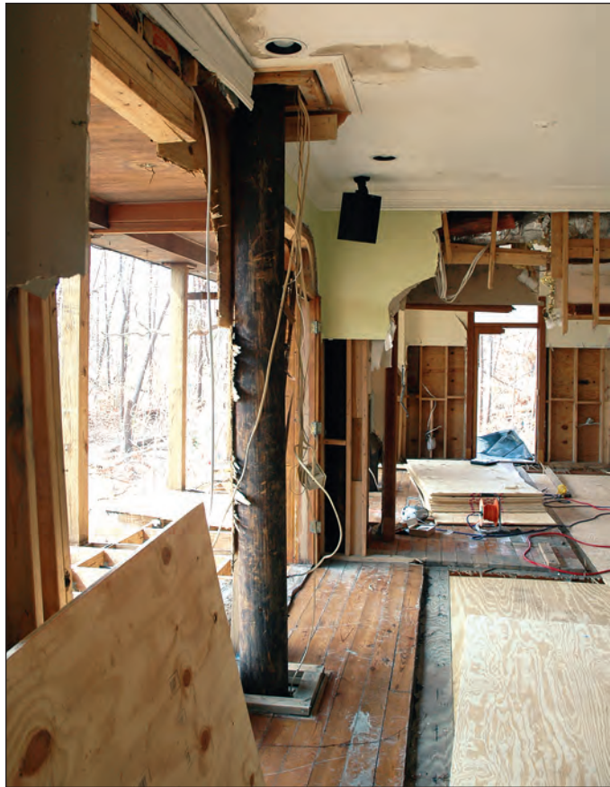
Figure 4-14. Wave damage to floors and walls, but pole construction left a repairable, surviving building (Waveland, Mississippi)
