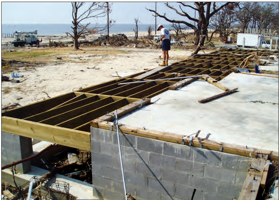
Figure 4-40. Stem wall foundation survived intact, but waves and surge above the floor destroyed the house, sweeping it off the foundation (Waveland, Mississippi).
