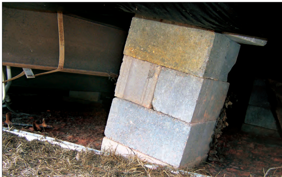
Figure 4-42. Dry-stacked pier under home rotated 20 degrees from vertical (Pass Christian, Mississippi).
