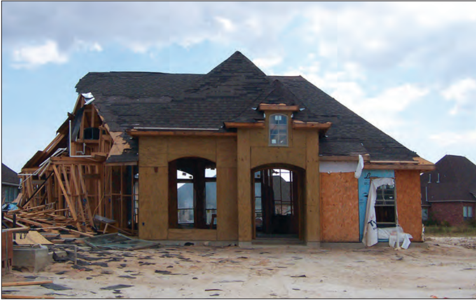
Figure 4-88. Home under construction whose garage collapsed and that racked laterally approximately 1 foot. Sheathing in the shear walls in the front of the home were found to be inadequately fastened to the wall framing (estimated wind speed: 120 mph. St. Tammany Parish, Louisiana).
