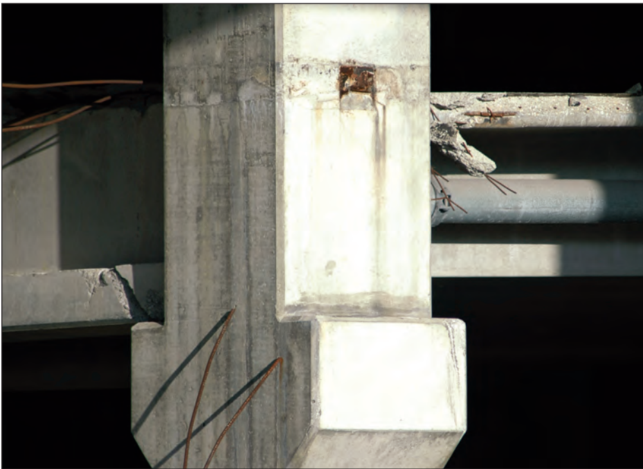
Figure 4-65. Another view of the collapse of first elevated level of pre-stressed parking decks shown in Figure 4-64 (Biloxi, Mississippi)
