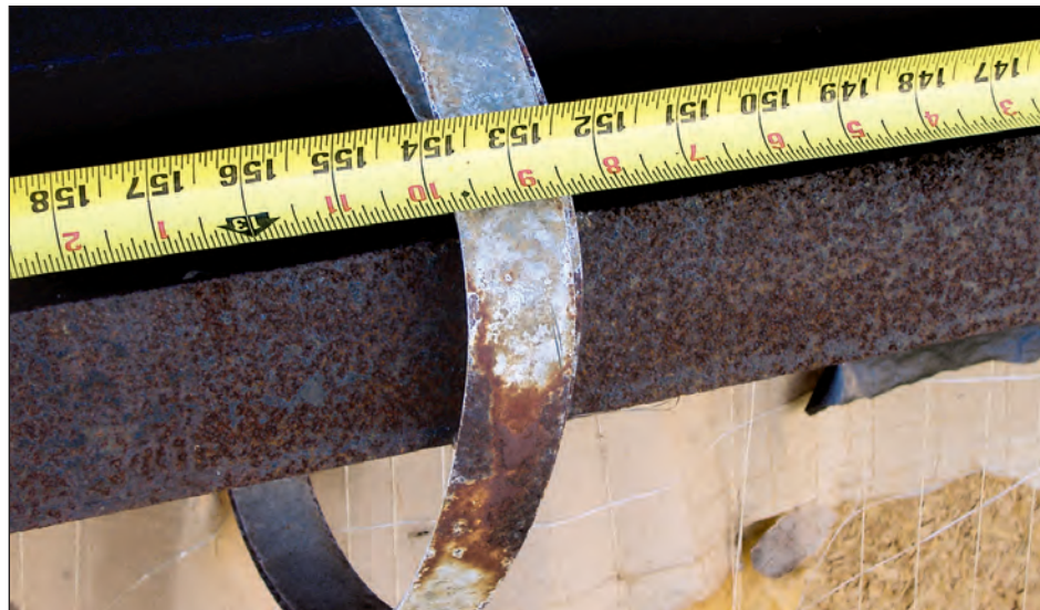
Figure 4-101. The metal straps were spaced approximately 13 feet on center on a manufactured home located in Exposure C (estimated wind speed: 110 mph. Chalmette, Louisiana).
