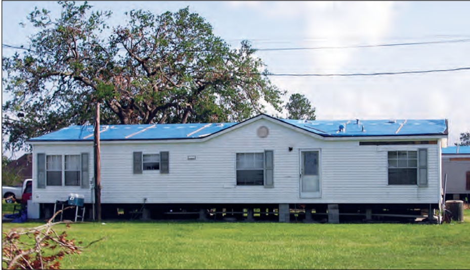
Figure 4-103. Newer manufactured home located in Exposure C with roof covering damage (estimated wind speed: 110 mph. Plaquemines Parish, Louisiana)
