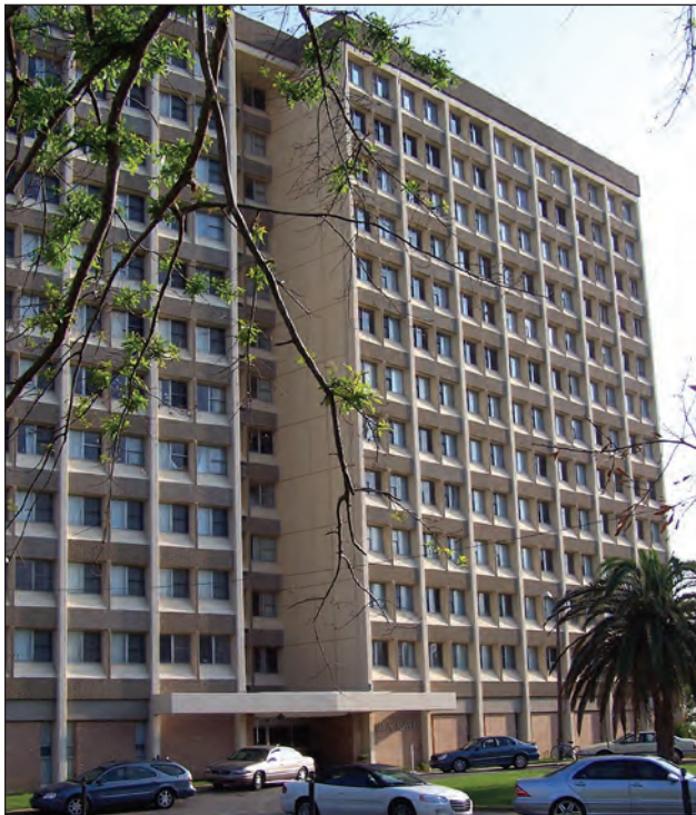
Figure 3-43. Multi-family residential building constructed with reinforced concrete frame showed no visible structural damage (Ocean Springs, Mississippi)
