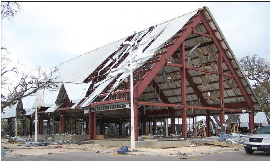
Figure 3-51. Wind, wave, and surge damage to St. Thomas Catholic Church. Destruction of the PEMB envelope likely reduced wind damage to the structure itself (Long Beach, Mississippi).
