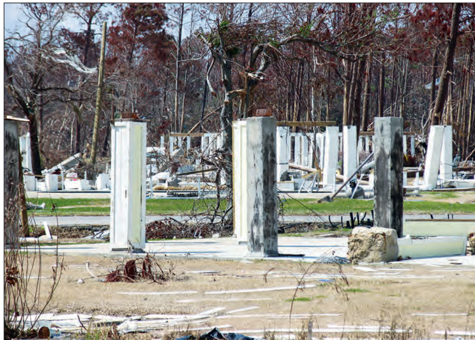
Figure 4-24. Typical building failures when surge and waves exceeded pier foundation height (Long Beach, Mississippi)
