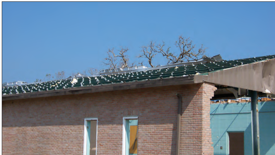
Figure 4-121 Severely damaged PEMB estimated to be 30 years old (estimated wind speed: 130 mph. Pass Christian, Mississippi)
