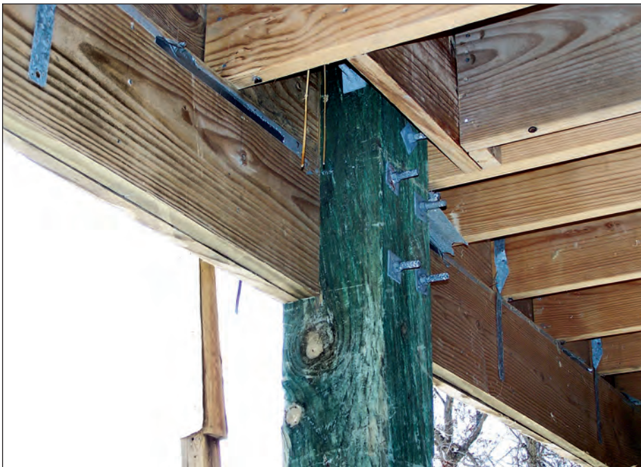
Figure 4-81. Coastal home located in Exposure C that is well connected with beam-to-column lap joints and galvanized bolts and straps (estimated wind speed: 120 mph. Ocean Springs, Mississippi)
