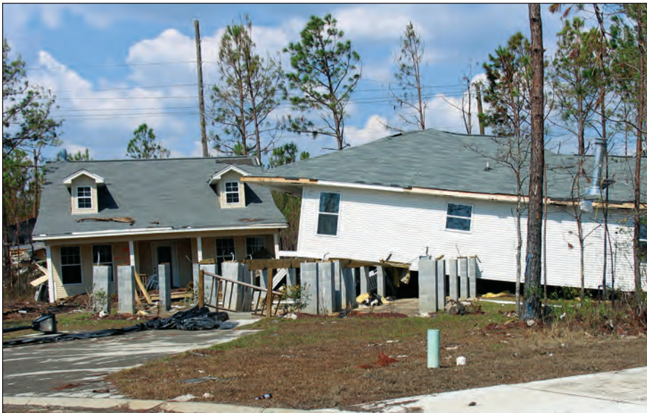
Figure 4-31. Failure of pier-to-beam connections due to wave and flood forces acting on the elevated building (Long Beach, Mississippi)
