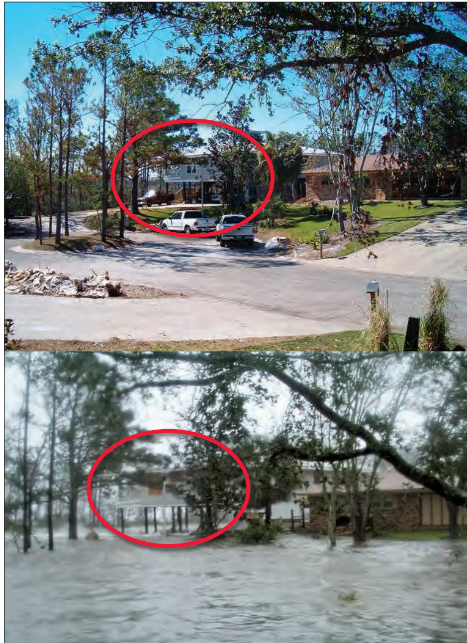
Figure 4-21. Successful pole construction home (background) near Old Fort Bayou. The top photo was taken approximately 3 weeks after Hurricane Katrina. The lower photo was taken during Katrina (the water level had dropped approximately 6 feet from its peak when the photo was taken) (Ocean Springs, Mississippi).
