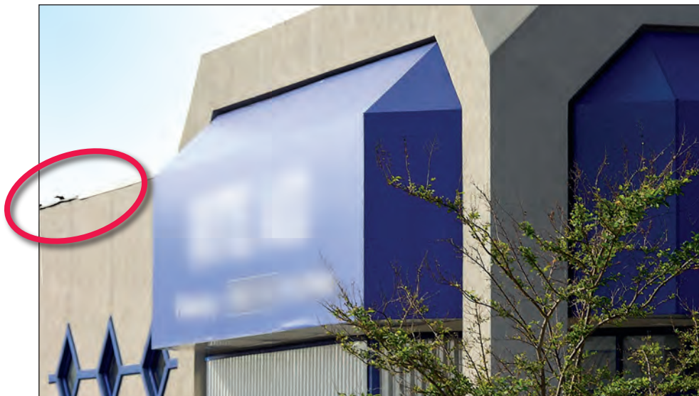
Figure 3-52. Newer low-rise PEMB that performed well structurally, but experienced some envelope damage. Metal coping along the top of the left wall (circle) was lifted by high winds (Bay St. Louis, Mississippi).
