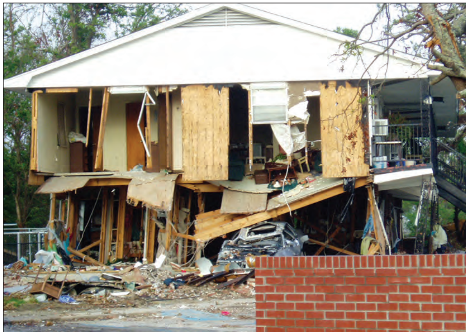
Figure 3-13. Apartments damaged by storm surge, floating automobiles, and wave action (Biloxi, Mississippi)
