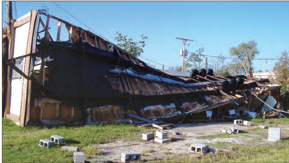
Figure 4-100. Manufactured home rolled over by Hurricane Katrina's winds (estimated wind speed: 110 mph. Chalmette, Louisiana)
