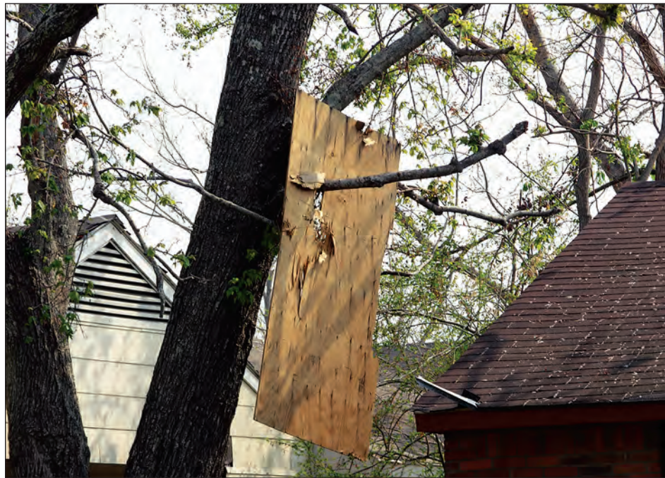
Figure 3-31. Roof sheathing was a source of windborne debris (Waveland, Mississippi).
