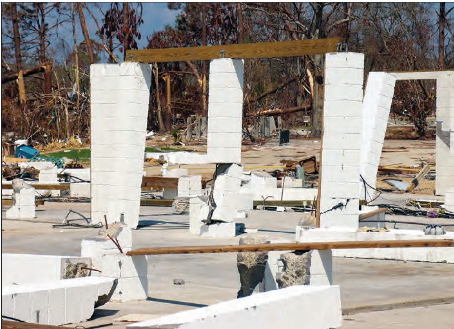
Figure 4-29. Pier breakage (Long Beach, Mississippi)
