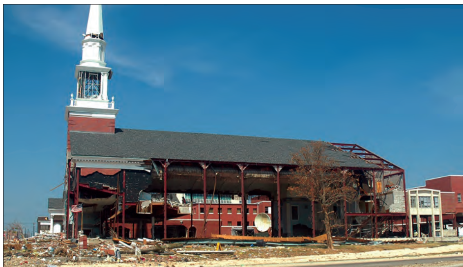
Figure 4-57. Steel-framed church that was gutted by waves, but the roof remained in place (Biloxi, Mississippi)
