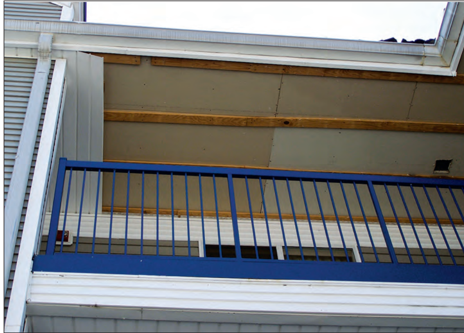
Figure 4-79. Properly attached gypsum board substrate avoided attic pressurization and entrance of wind-driven rain when the finish soffit material was lost (estimated wind speed: 120 mph. Ocean Springs, Mississippi).
