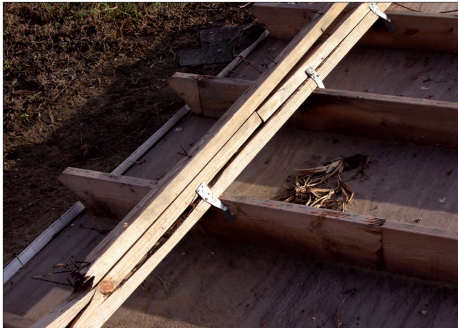
Figure 4-90. Framing anchors were used to connect rafters to top plate, but no framing anchors connected top plate to wall framing at this house located in Exposure C (estimated wind speed: 110 mph. Plaquemines Parish, Louisiana).
