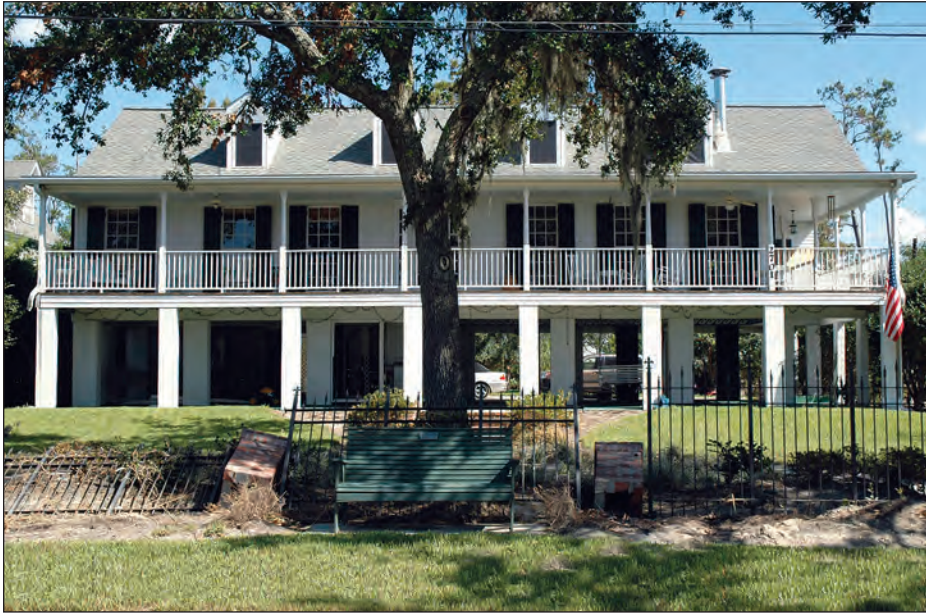
Figure 4-22. Pier-supported house with minimal flood damage (Mandeville, Louisiana)
