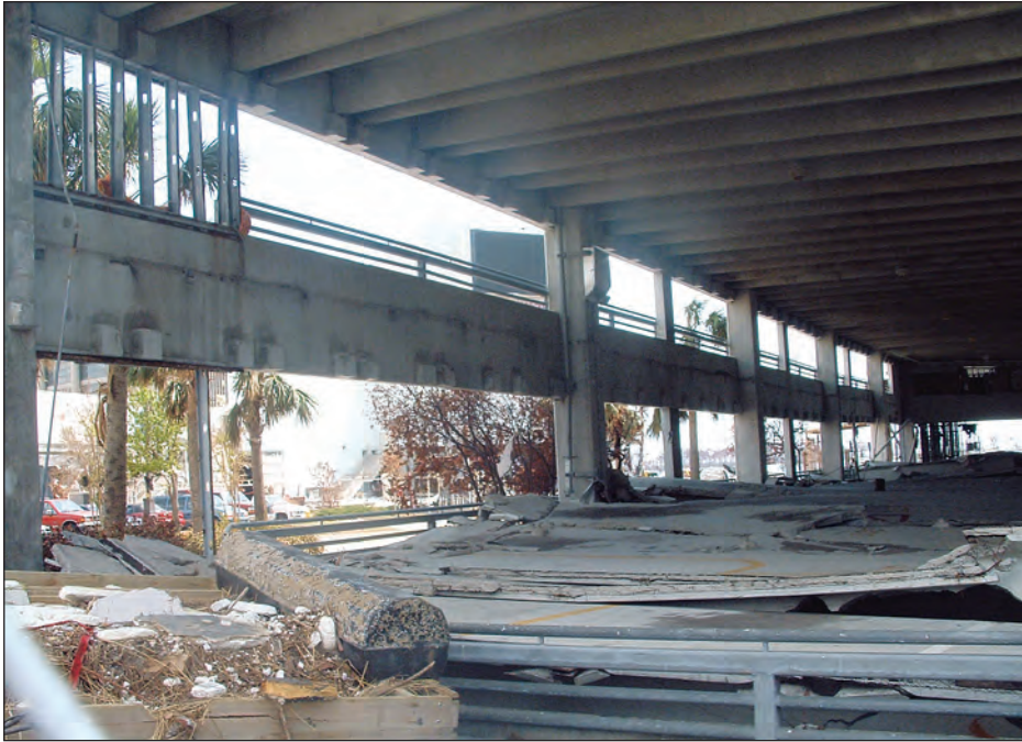
Figure 4-64. Collapse of first elevated level of pre-stressed parking decks due to poor column-to-beam gravity connections that failed when exposed to lateral and uplift wave forces (see Figure 4-65) (Biloxi, Mississippi)
