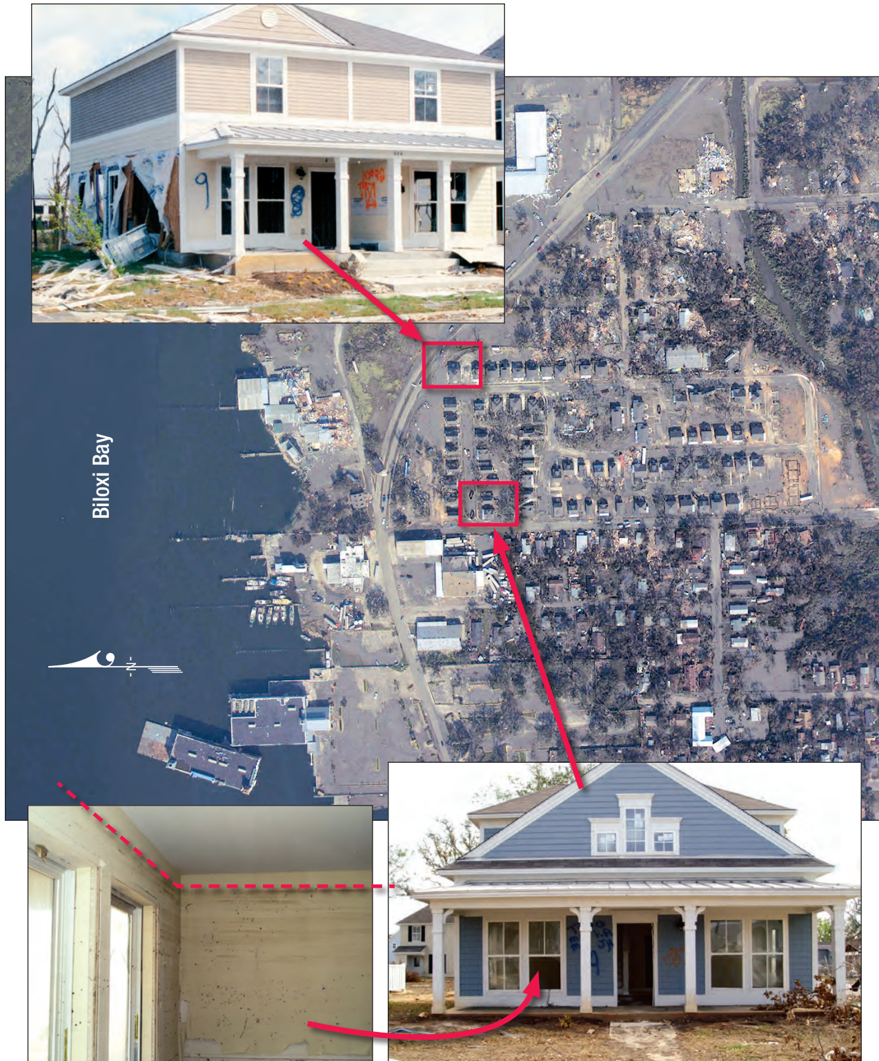
Figure 3-10. This new public housing neighborhood (not yet occupied) was flooded by storm surge to the first floor ceilings. Houses closest to the bay also sustained damage to walls by waves and floodborne debris. The arrows indicate the locations of the inset photos (Biloxi, Mississippi).
