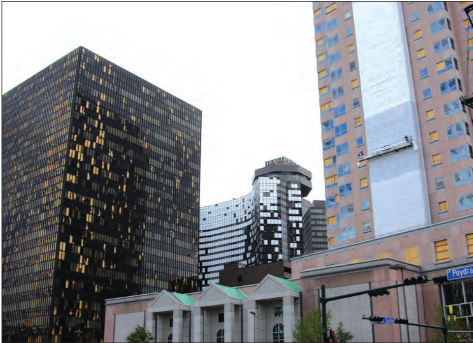
Figure 3-29. Roof aggregate was the primary windborne debris source for the window damage (New Orleans, Louisiana).
