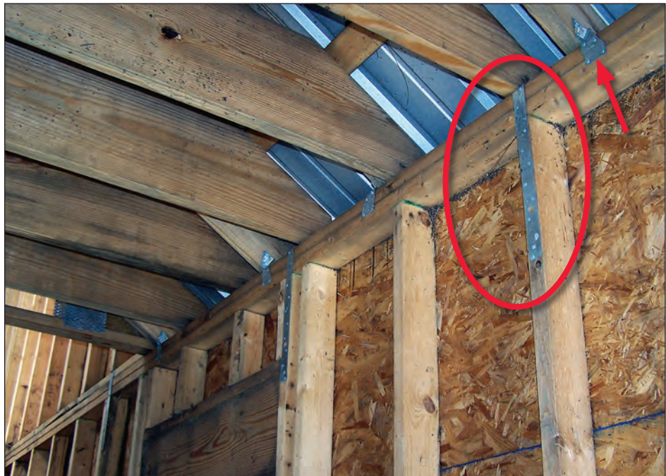
Figure 4-83. Home located in Exposure C with rafter-wall connectors and top plate- stud connectors. Note the rafter-top plate connector (arrow) is more effective to install on opposite side of wall, and the top plate stud connector (circle) (estimated wind speed: 130 mph. Pass Christian, Mississippi).
