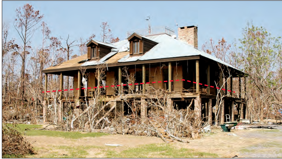
Figure 4-14. Wave damage to floors and walls, but pole construction left a repairable, surviving building (Waveland, Mississippi)
