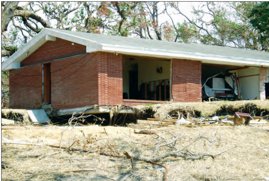
Figure 4-35. Slab-on-grade undermining (Ocean Springs, Mississippi)
