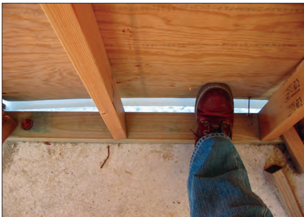
Figure 4-91 (a) and 4-91 (b). Wall framing was inadequately secured to the bottom plate with fasteners spaced over 32 inches on center. The presence of building wrap shows that no additional nailing was planned (estimated wind speed: 130 mph. St. Bernard Parish, Louisiana).
