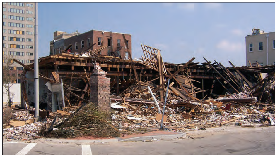
Figure 4-113. Wind-induced damage to older unreinforced masonry building located in Exposure C (estimated wind speed: 130 mph. Gulfport, Mississippi)
