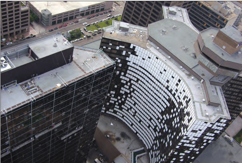
Figure 3-47. Roof aggregate was the primary windborne debris source for the glazing damage to the hotel and office building (New Orleans, Louisiana).
