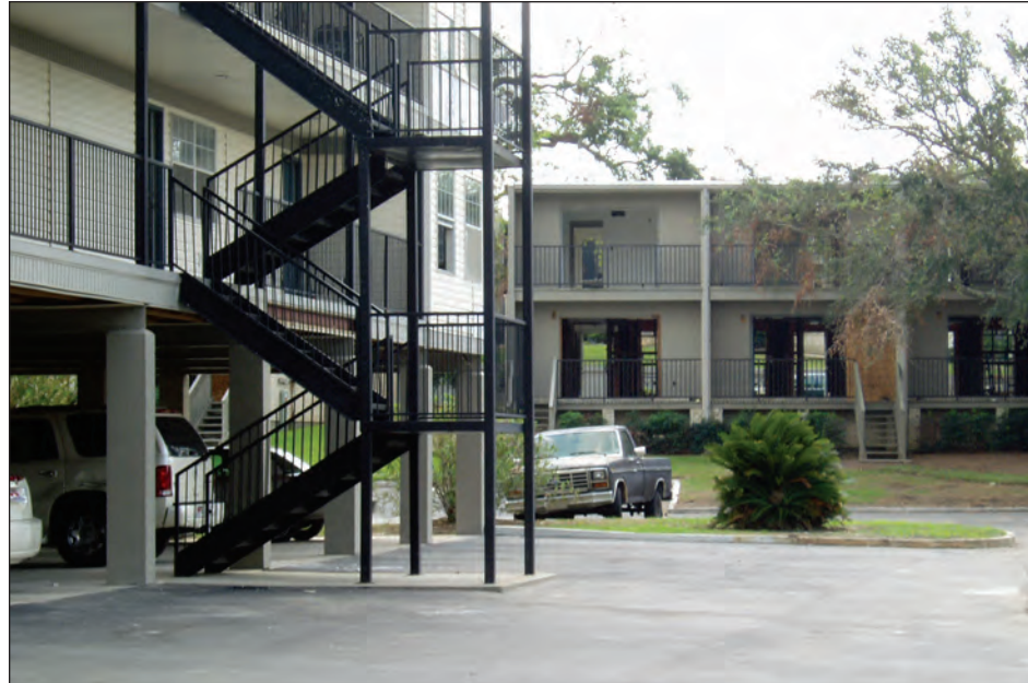
Figure 3-16. Wood-framed and masonry multi-family residential buildings damaged by storm surge (limited wave action). The building in foreground sustained flooding to a level approximately 30 inches above the elevated floor. The building in the background was flooded to the ceiling of the lower floor units (Ocean Springs, Mississippi).
