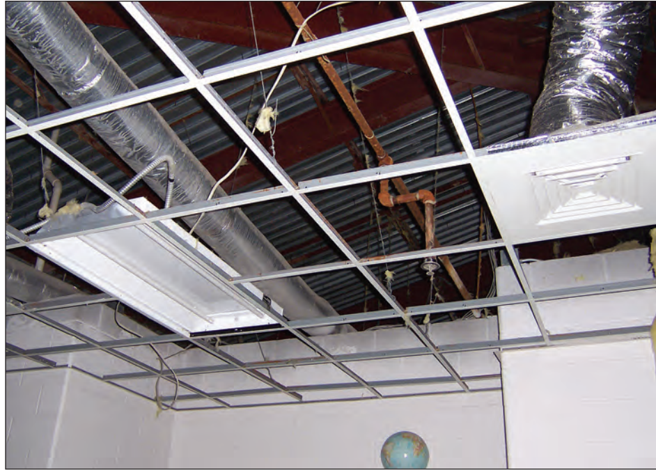
Figure 3-57. Ceiling damaged by wind and rain entry due to soffit failure (Gulfport, Mississippi)
