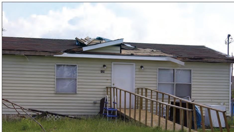
Figure 4-102. Newer manufactured home located in Exposure C that lost the gable roof over its entrance (estimated wind speed: 110 mph. Plaquemines Parish, Louisiana)
