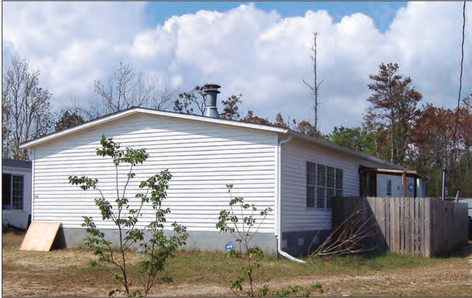
Figure 4-43. Manufactured home placed on and secured to poured concrete strip footing had floodwaters 6 feet above its floor, but was not moved from its foundation. Although this indicates good foundation performance, the cost of repairing may exceed the value of the residence because of the significant inundation damage (Ocean Springs, Mississippi).
