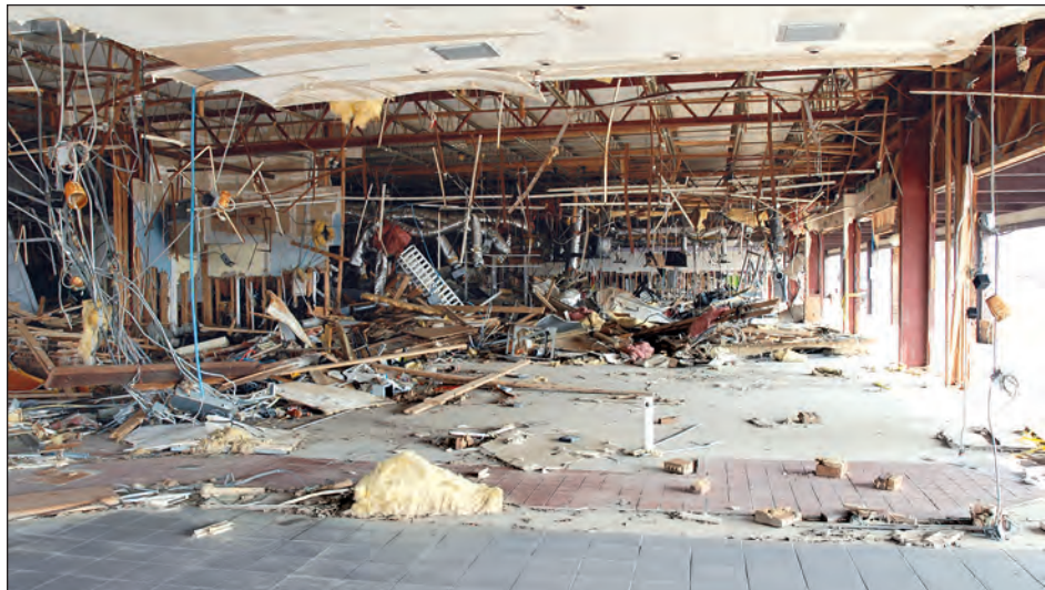
Figure 4-56. Interior of steel-framed strip mall construction shown in Figure 4-55 (Gulfport, Mississippi)
