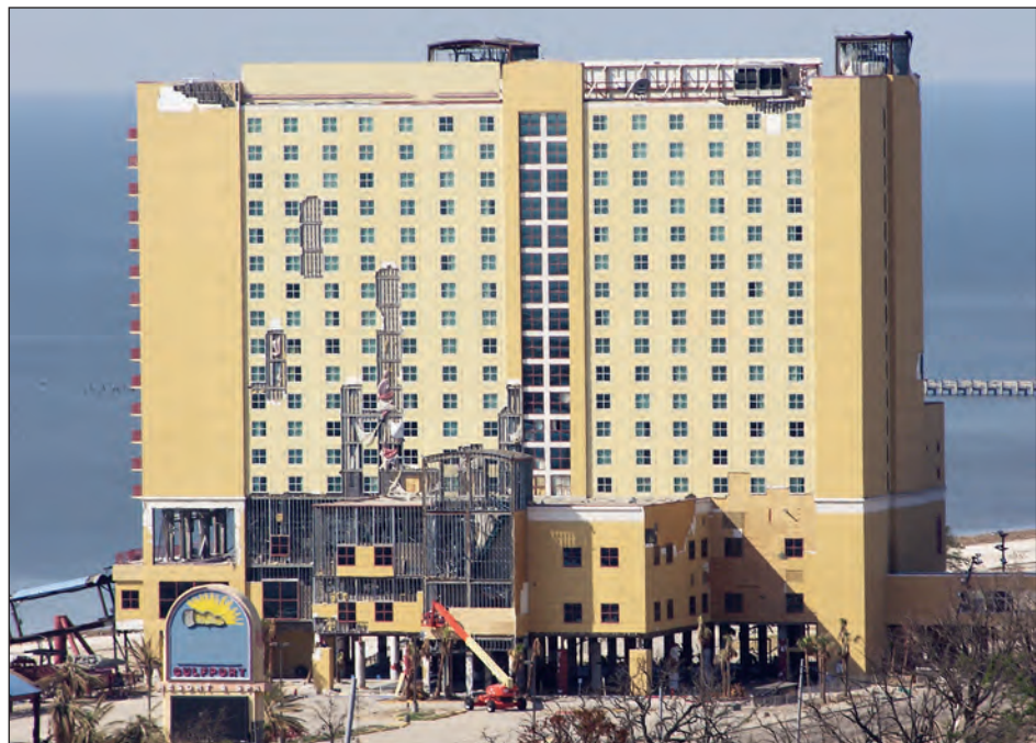
Figure 3-45. Damage to EIFS on hotel and casino (Biloxi, Mississippi)
