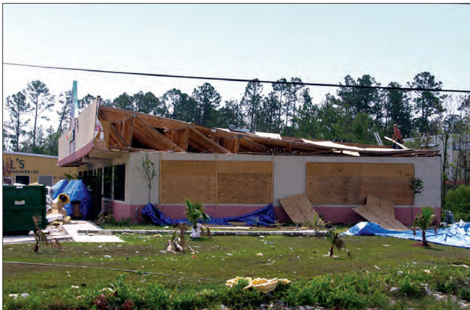
Figure 4-107. Failure in a wood-framed commercial building. Trusses lost roof sheathing, allowing trusses to tip over (estimated wind speed: 120 mph. Ocean Springs, Mississippi).
