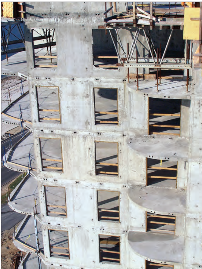
Figure 4-111. East tower located in Exposure C under construction with reinforced concrete and post-tensioned floor slabs. The east tower was water-inundated on the first floor and suffered only minor wind damage to the roof covering of the finished tower (estimated wind speed: 120 mph. Biloxi, Mississippi).
