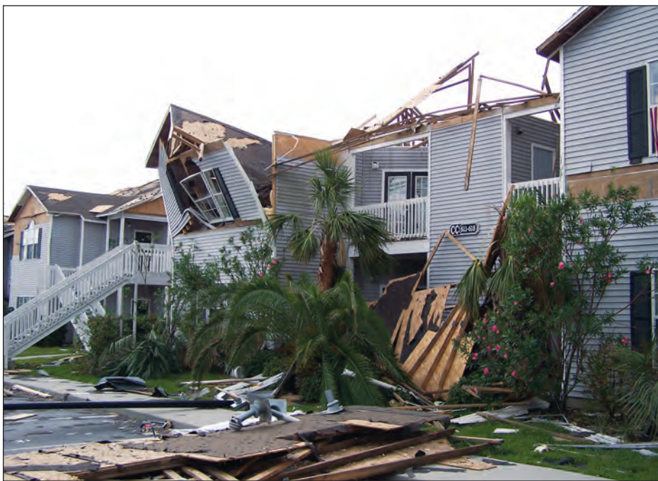
Figure 4-74. Two-story apartment building that lost its roof diaphragm and load path connections (estimated wind speed: 120 mph. Ocean Springs, Mississippi)
