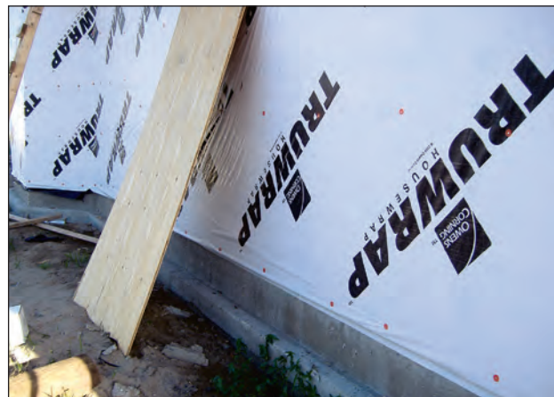
Figure 4-91 (a) and 4-91 (b). Wall framing was inadequately secured to the bottom plate with fasteners spaced over 32 inches on center. The presence of building wrap shows that no additional nailing was planned (estimated wind speed: 130 mph. St. Bernard Parish, Louisiana).
