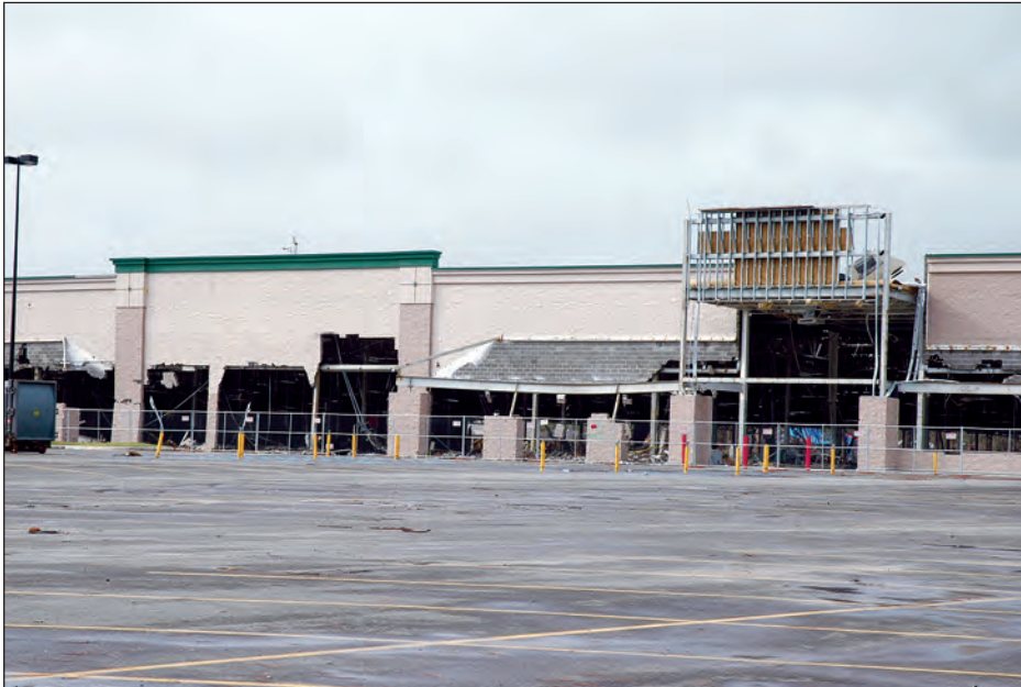
Figure 4-58. Large retail store that was gutted by waves, but most of the roof remained in place (Pass Christian, Mississippi)
