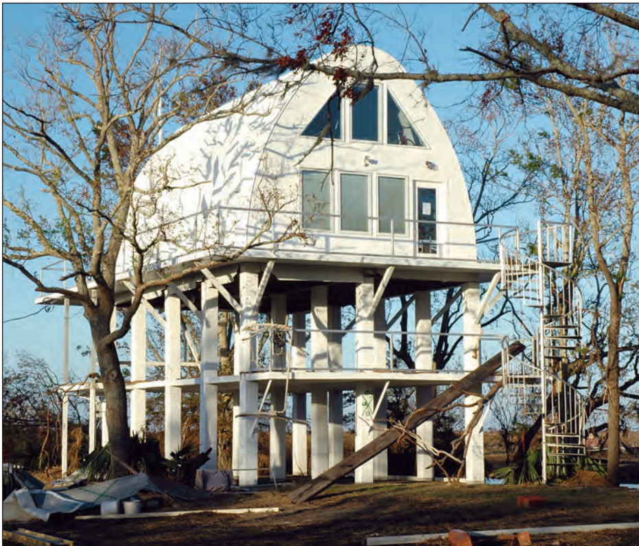
Figure 4-9. Successful house on high pile foundations, well above the local BFE (Shell Beach, Louisiana)
