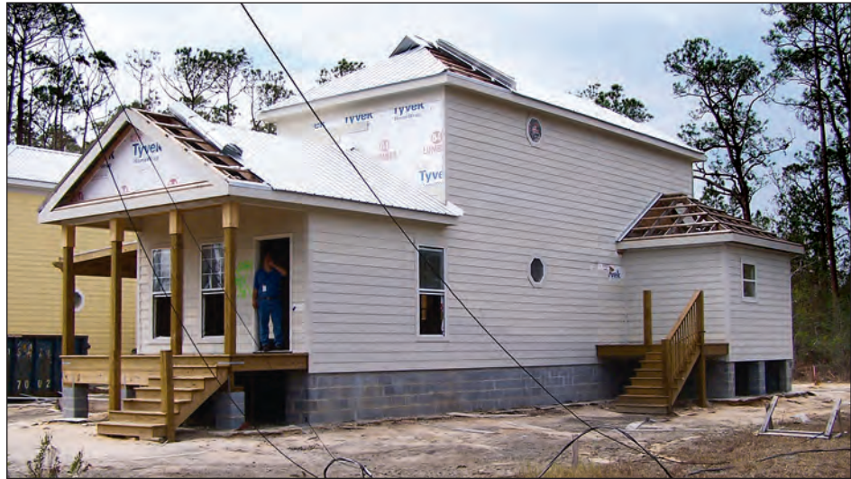
Figure 4-82. Home under construction subjected to flood and wind damage (estimated wind speed: 130 mph. Pass Christian, Mississippi)
