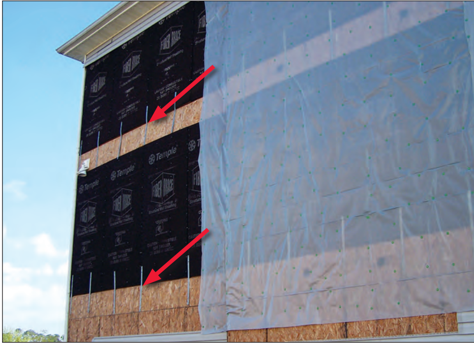
Figure 4-84. Two-story structure with floor-to-floor connectors (arrows) that are adequately spaced, but improperly attached (see Figure 4-83) (estimated wind speed: 120 mph. D'Iberville, Mississippi).
