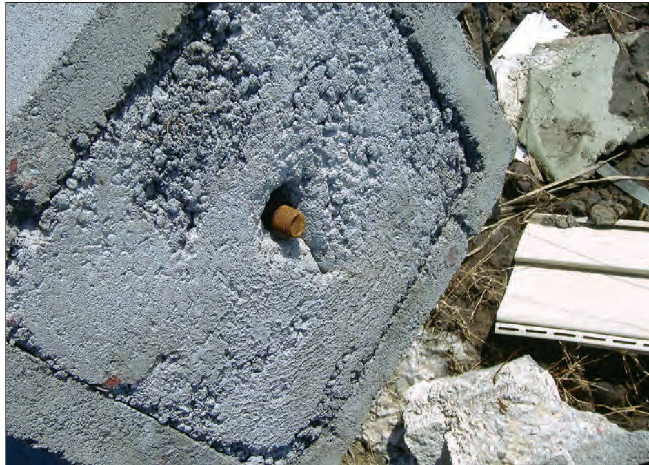
Figure 4-30. Failure from a poorly detailed pier to beam connection (Long Beach, Mississippi)
