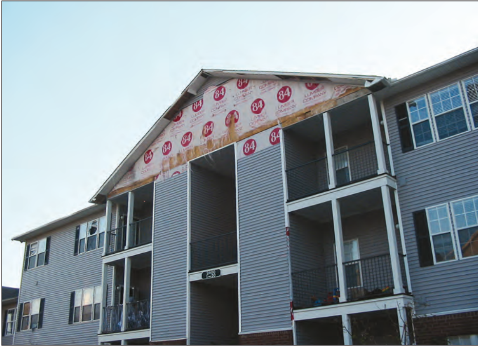
Figure 4-99. Apartment building with gable end walls that were constructed with OSB sheathing under housewrap (estimated wind speed: 120 mph. D'Iberville, Mississippi)
