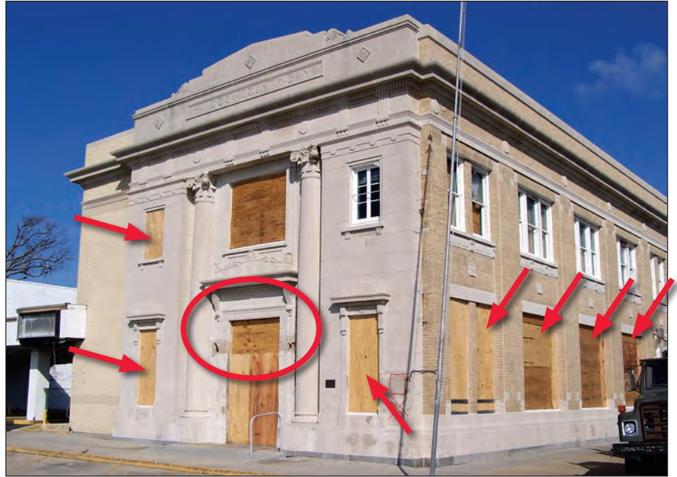
Figure 4-116. Heavy masonry Hancock Bank Building located in Exposure C on Highway 49. Note the location of a missing awning (circle) and damaged windows (arrows) (estimated wind speed: 130 mph. Pass Christian, Mississippi).
