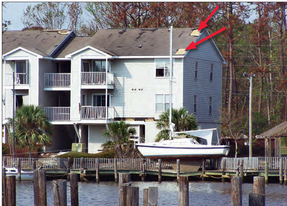
Figure 4-76. Roof corners, edges, and ridges are zones of increased wind pressures (arrows), as seen in this apartment complex (estimated wind speed: 120 mph. Ocean Springs, Mississippi).
