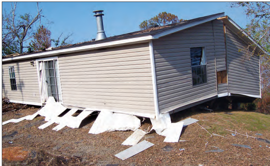
Figure 4-41. Collapse of manufactured home due to loss of anchorage and pier settlement (indicative of soil saturation under flooded conditions) (Pass Christian, Mississippi).
