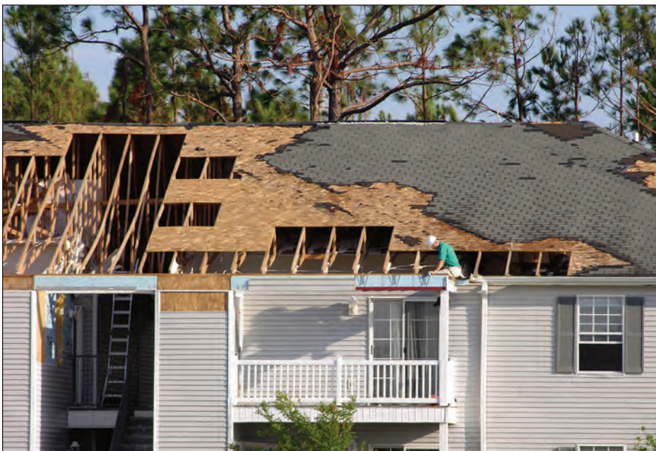
Figure 4-96. Metal connectors were lacking on the gabled roofs over the porches and entrances. Several roof structures were blown off (estimated wind speed: 130 mph. Long Beach, Mississippi).
