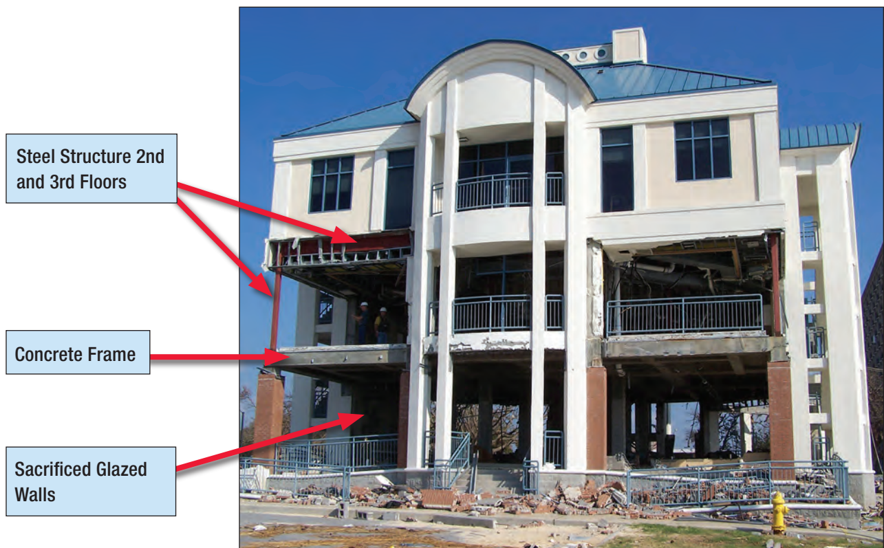
Figure 4-59. Biloxi Harbor Master Administration Building with a hybrid structural system, concrete and steel (Biloxi, Mississippi)
