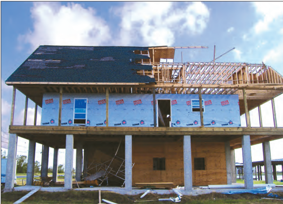
Figure 4-89. Home located in Exposure C that lost portions of its roof structure (estimated wind speed: 110 mph. Plaquemines Parish, Louisiana)
