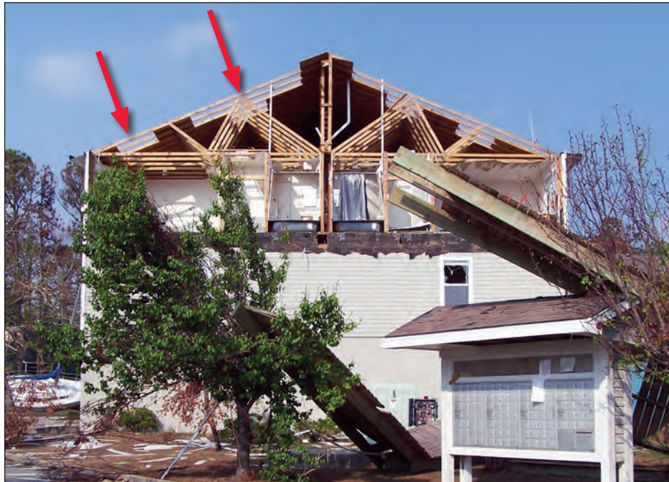
Figure 4-75. Failure of the gable end wall of this apartment building led to pressurization of the attic and the release of sheets of plywood sheathing. Note the plywood roof sheathing “unzipped” by wind pressures (arrows) (estimated wind speed: 120 mph. Ocean Springs, Mississippi).
