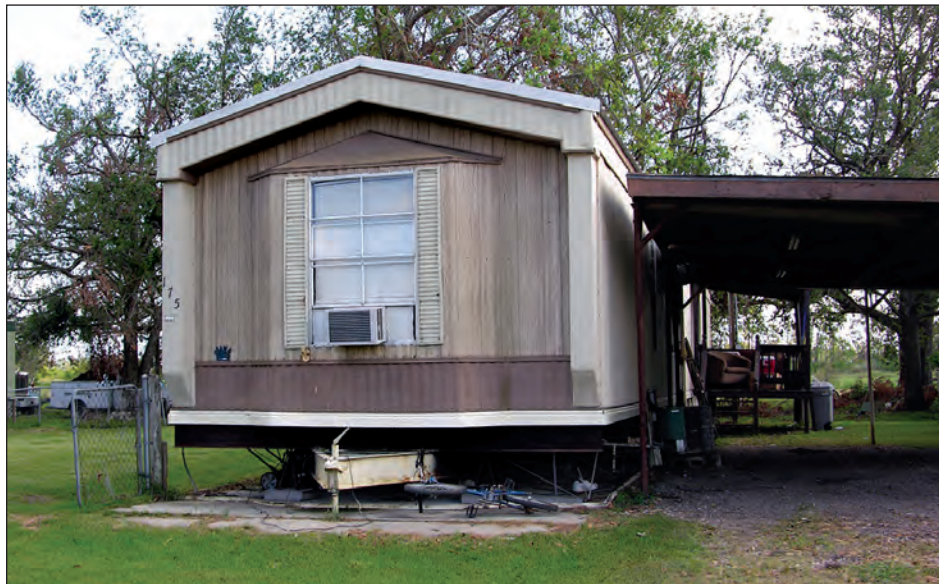
Figure 4-106. Manufactured home located in Exposure C secured to taut anchors in the concrete slab (estimated wind speed: 110 mph. Plaquemines Parish, Louisiana)
