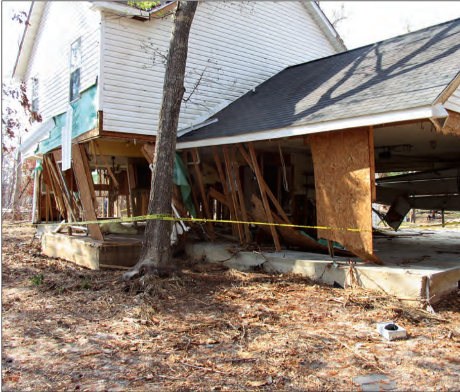
Figure 3-8. Wave and surge damage to load- bearing walls atop stem wall foundation. The house was located in flood hazard zone C, approximately 1/4 mile from the shoreline (Pointe Aux Chens area, Jackson County, Mississippi).
