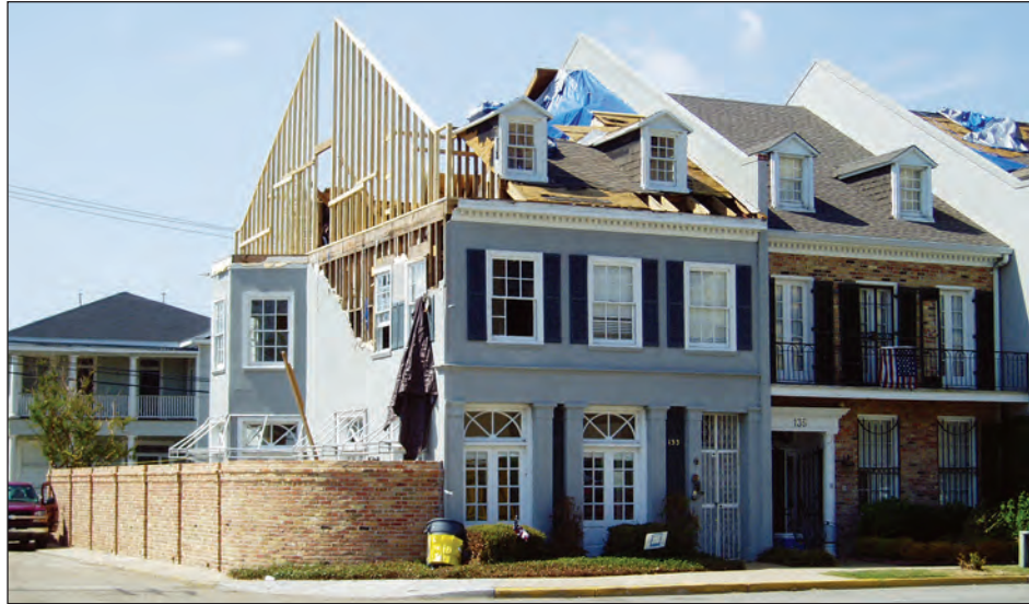
Figure 3-34. Row house with failed gable end wall and roof (gable end wall was being replaced when this photo was taken) (Biloxi, Mississippi).
