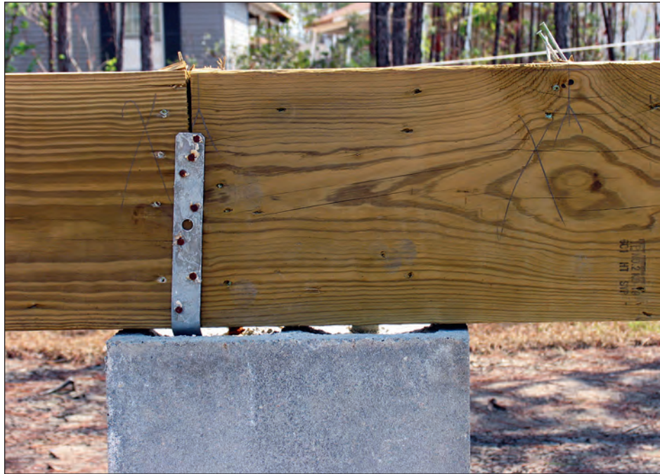
Figure 4-33. Poor pier-to-beam connection. Although this particular connection did not fail (because the wall and floor-to-beam connections failed first), this connection is poor. Note use of light gauge metal straps and nailing of strap at a joint in the beam (Pass Christian, Mississippi).
