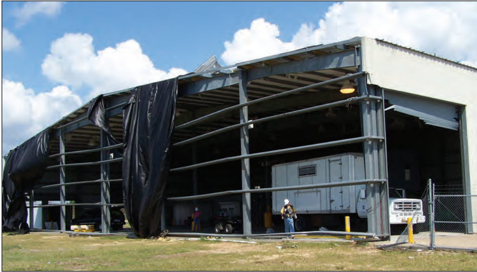
Figure 3-50. Low-rise PEMB at the Gulfport-Biloxi Airport severely damaged by winds. The building was constructed with steel moment frames and purlins, and metal roof and wall panels (Gulfport, Mississippi).
