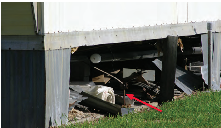
Figure 4-105. Ground anchors at manufactured home located in Exposure C (estimated wind speed: 110 mph. Plaquemines Parish, Louisiana)
