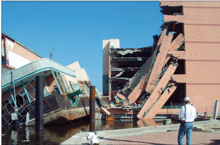
Figure 4-66. Parking deck collapse due to impact by casino barge, on left (Biloxi, Mississippi)
