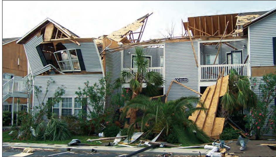
Figure 3-39. Apartment complex severely damaged by wind. Although wind speeds were less than current code-specified values, widespread and severe damage occurred at this development, a result of poor construction quality (Ocean Springs, Mississippi).
