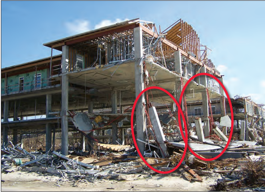
Figure 4-61. Multi-family property on Beach Boulevard with failed post-tensioned slabs and columns. Note the post-tensioning tendons (circles) (Pass Christian, Mississippi).
