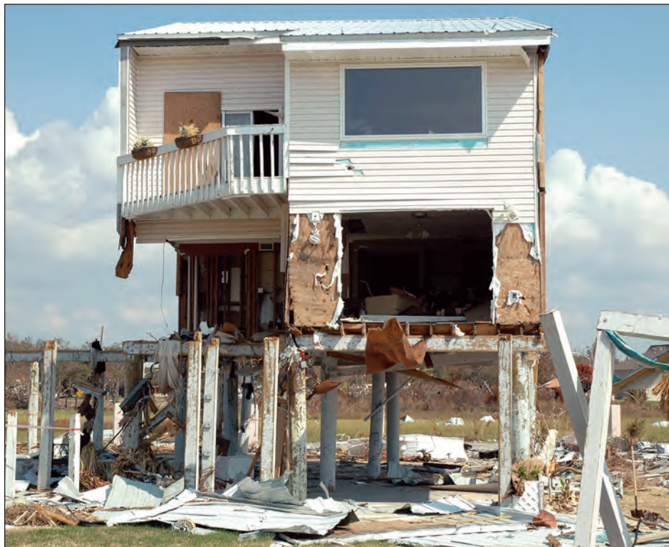
Figure 4-49. Severely damaged condominium unit was the only one remaining of 20 units (Pascagoula, Mississippi)
