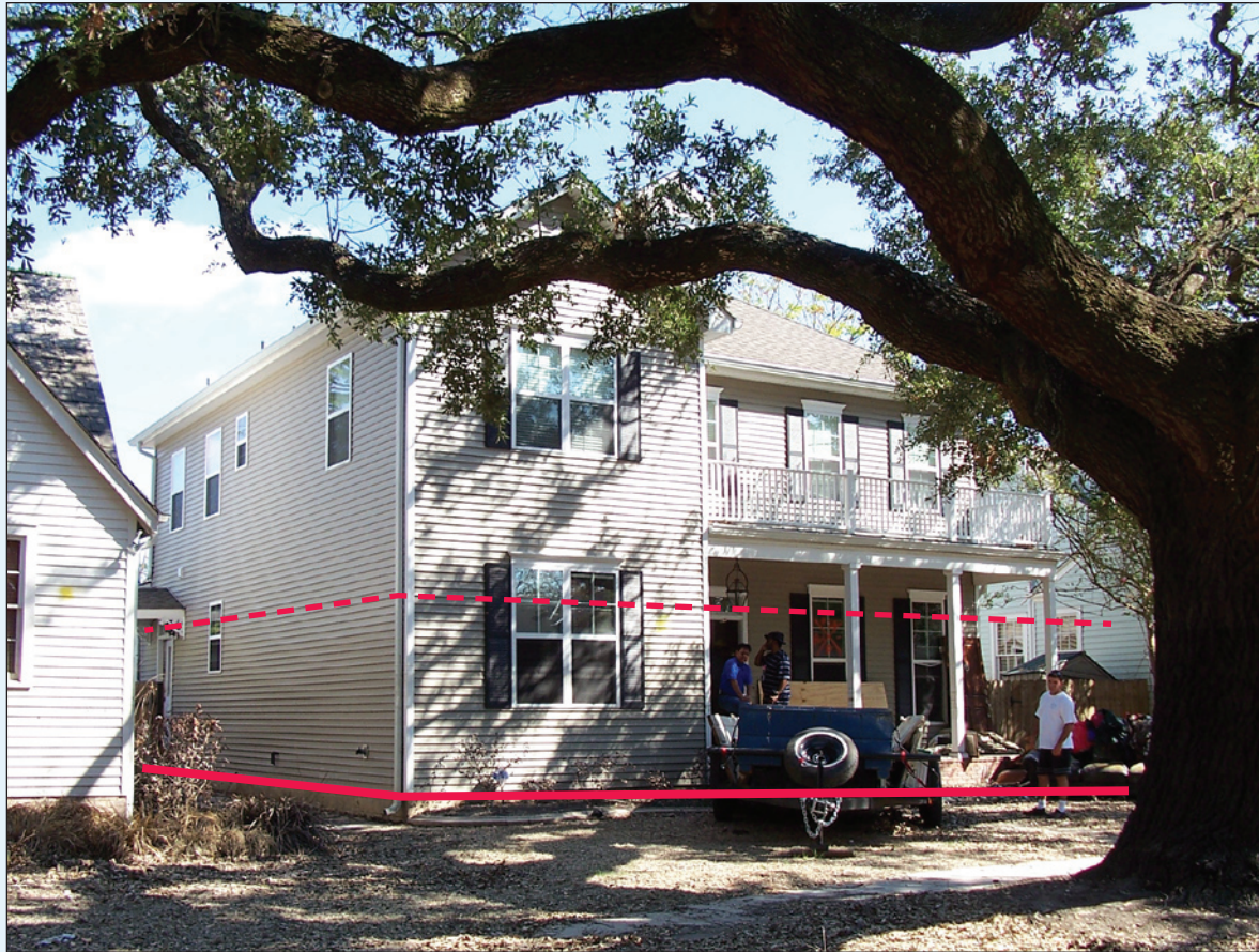
Figure 2-6. Note the actual flood depth from Hurricane Katrina (dashed line) vs. the BFE (solid line).
