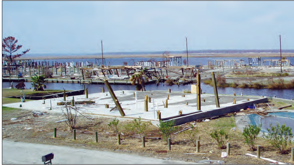
Figure 4-17. Destruction of pile-and pier-supported homes (platform type construction) adjacent to the house shown in Figure 4-16. Only two homes out of approximately 100 survived in the neighborhood (Bay St. Louis, Mississippi).
