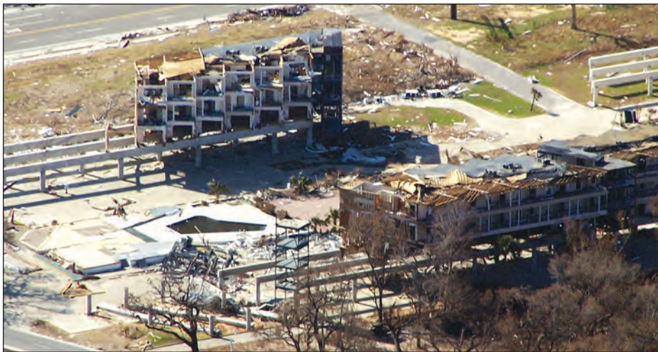
Figure 4-51. Condominium on heavy concrete foundation severely damaged when wave elevations exceeded lower floor elevations (Gulfport, Mississippi)
