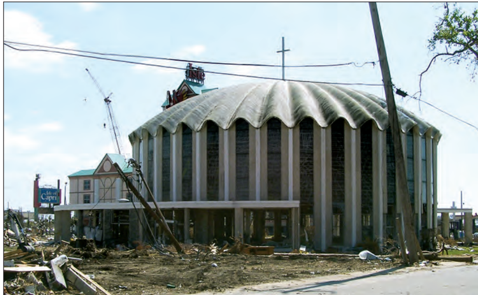
Figure 4-112. St. Michael's Catholic Church on Beach Boulevard (Highway 90), with its concrete shell roof and supporting concrete columns, was undamaged by Katrina's winds, but was severely damaged by the storm surge (estimated wind speed: 120 mph. Biloxi, Mississippi).
