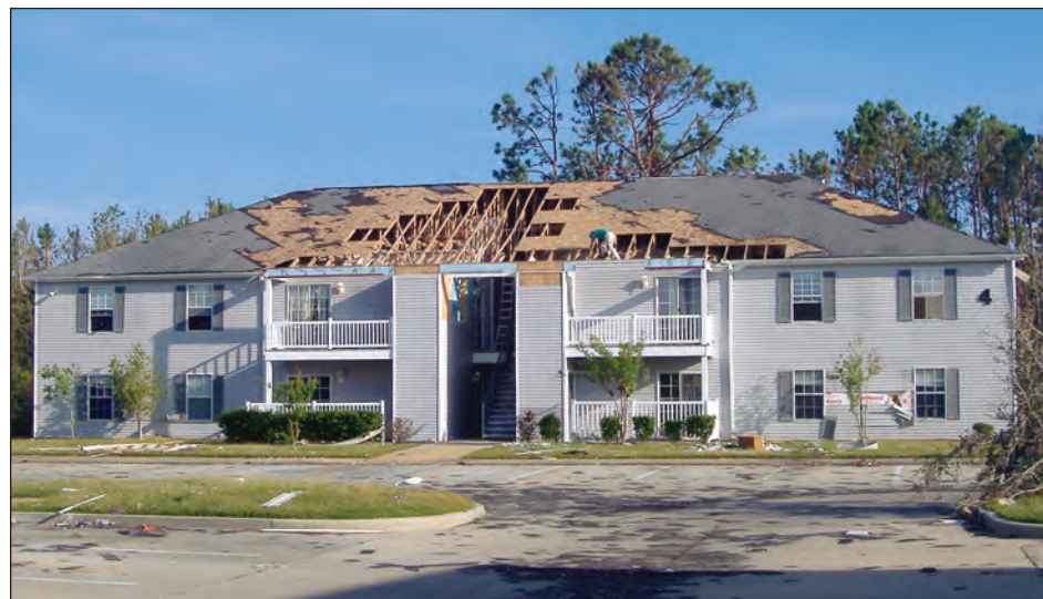
Figure 3-41. Wind damage to wood-framed, multi-family residential building (Long Beach, Mississippi)
