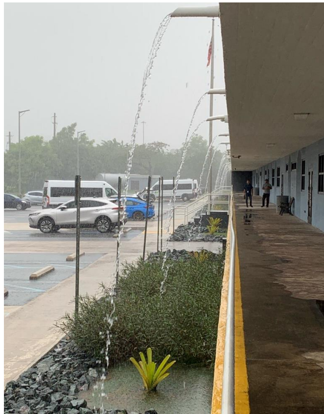
Figure 2-2. Bioretention planter boxes at the GSA federal facility in the municipality of Guaynabo during an afternoon rain
