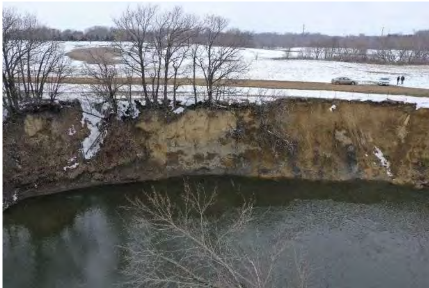
Figure 1 – Blue Earth River outer bank erosion and tree debris at damage site
