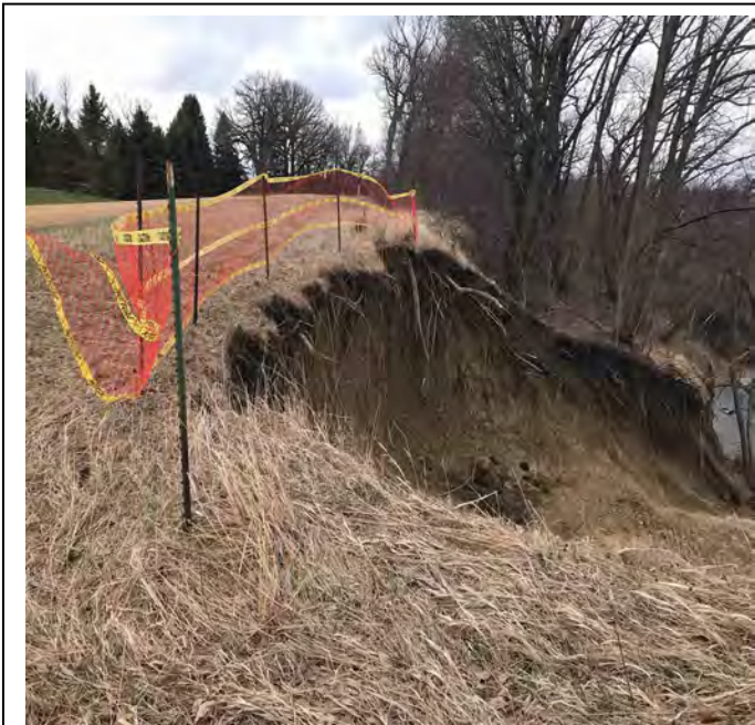
Site 3. Slope failure on 330 th AVE. 43.75472, -94.20634. Photo taken looking southwest.
