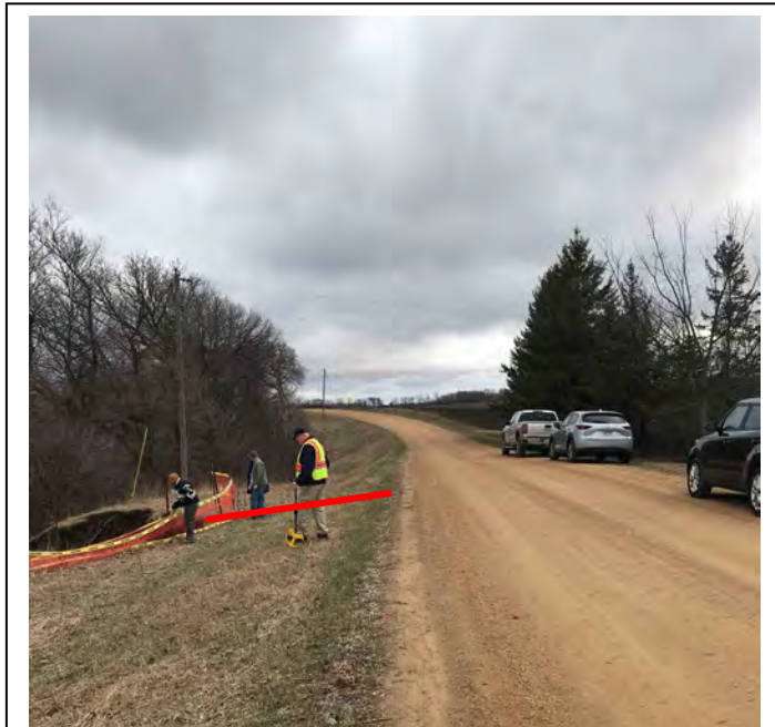
Site 3. Slope failure on 330 th AVE. 43.75472, -94.20634. Photo taken looking northeast. Red line indicates the point at which slope failure is closest to road, 15 ft.
