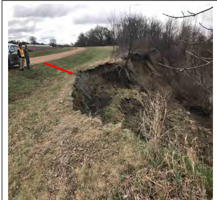
Site 2. Slope failure on 156 th Street. 43.75472, -94.14647 Photo taken looking southeast. Red line indicates the point at which slope failure is closest to road, 13 ft.
