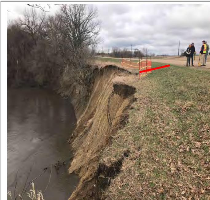
Site 1 slope failure. Red line indicates the point at which slope failure is closest to road, 13 ft. The gravel road in the photo is 150 th Street. Photo taken looking southwest.
