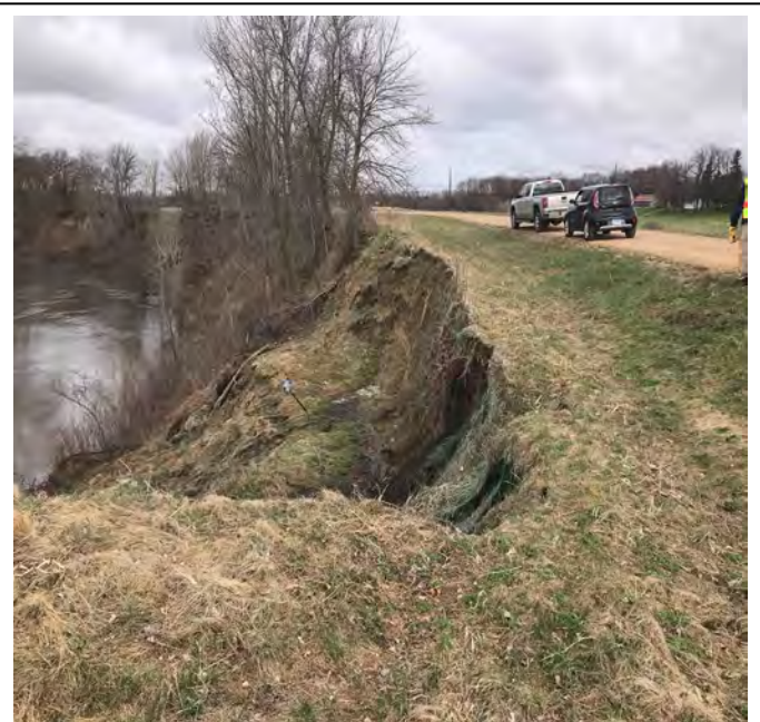
Site 2. Slope failure on 156 th Street. 43.75472, -94.14647 Photo taken looking northwest.
