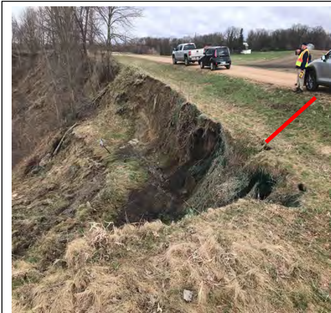
Site 2. Slope failure on 156 th Street. 43.75472, -94.14647 Photo taken looking northwest. Red line indicates the point at which slope failure is closest to road, 13 ft.
