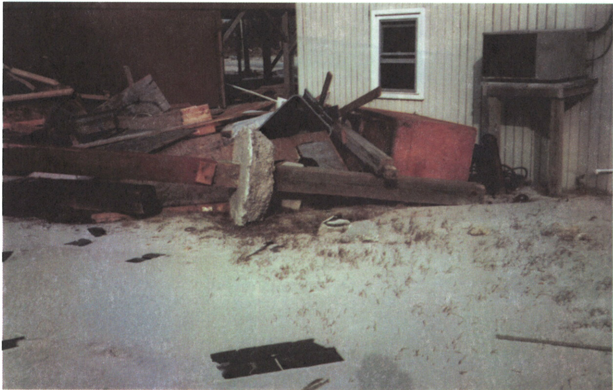
Figure 2-14 Storm-generated debris impacted nearby structure.
