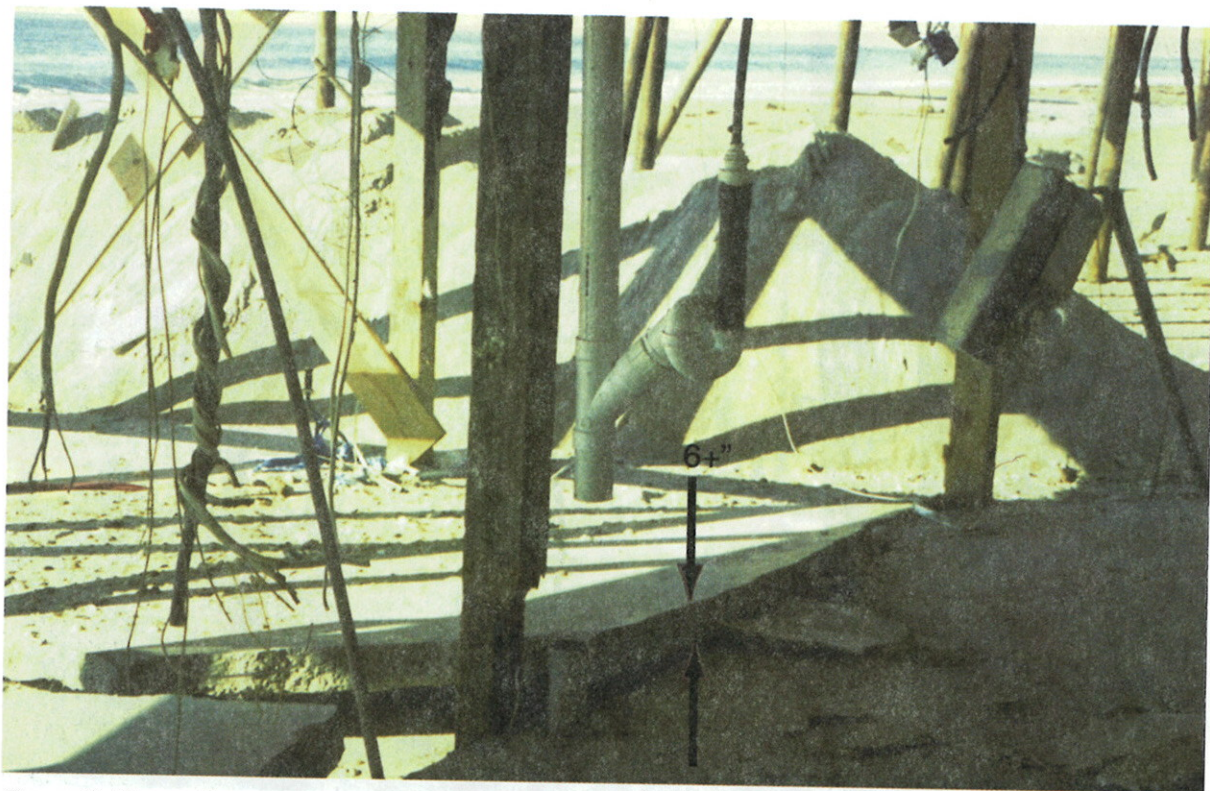
Figure 2-30 Example of unnecessarily thick slab.
