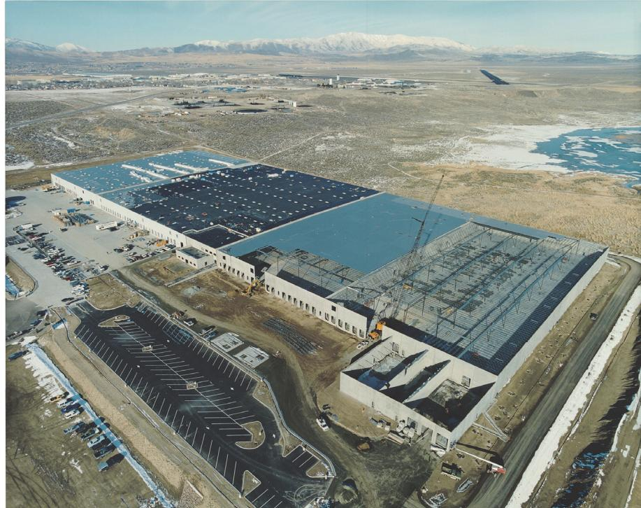
Figure 2-2      RWFD building with a bare steel deck diaphragm (photo credit:
