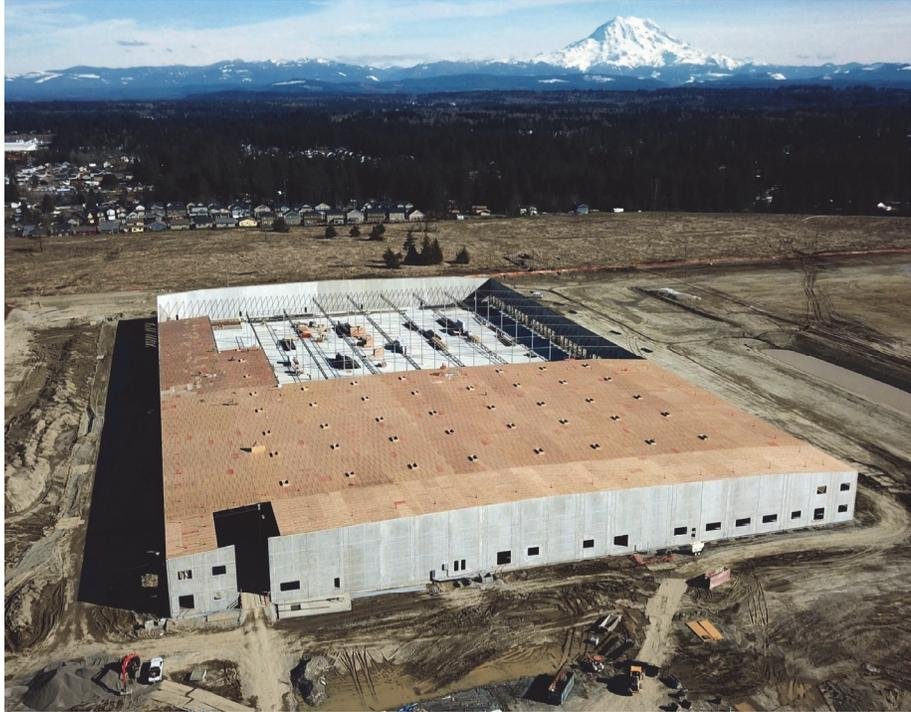
Figure 2-1 RWFD building with a wood structural panel diaphragm (photo credit: Panelized Structures).
