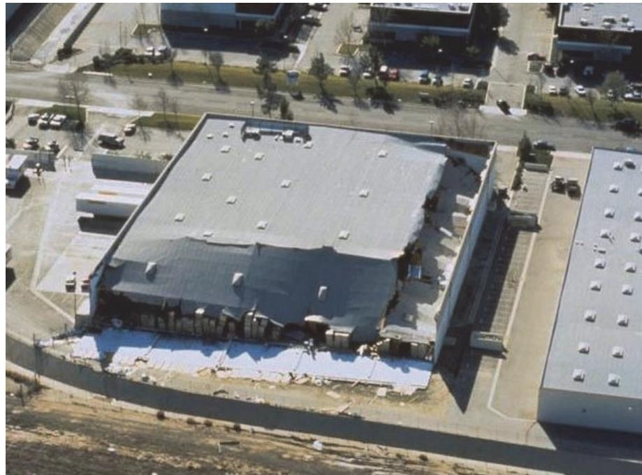
Figure 2-5 Partial collapse of a RWFD Building in the 1994 Northridge earthquake (photo credit: EERI).
