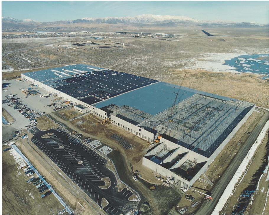
Figure 2-2 RWFD building with a bare steel deck diaphragm (photo credit: Vulcraft/Verco Group – A Division of Nucor).
