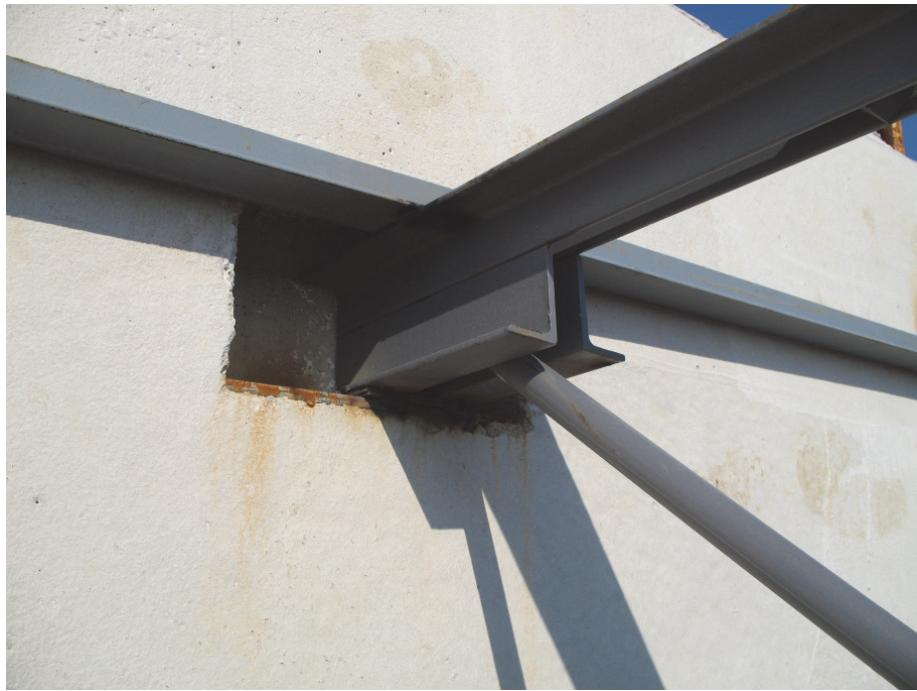
Figure 8-7 Joist seat in bearing pocket of wall (photo credit: Joseph Steinbicker).
