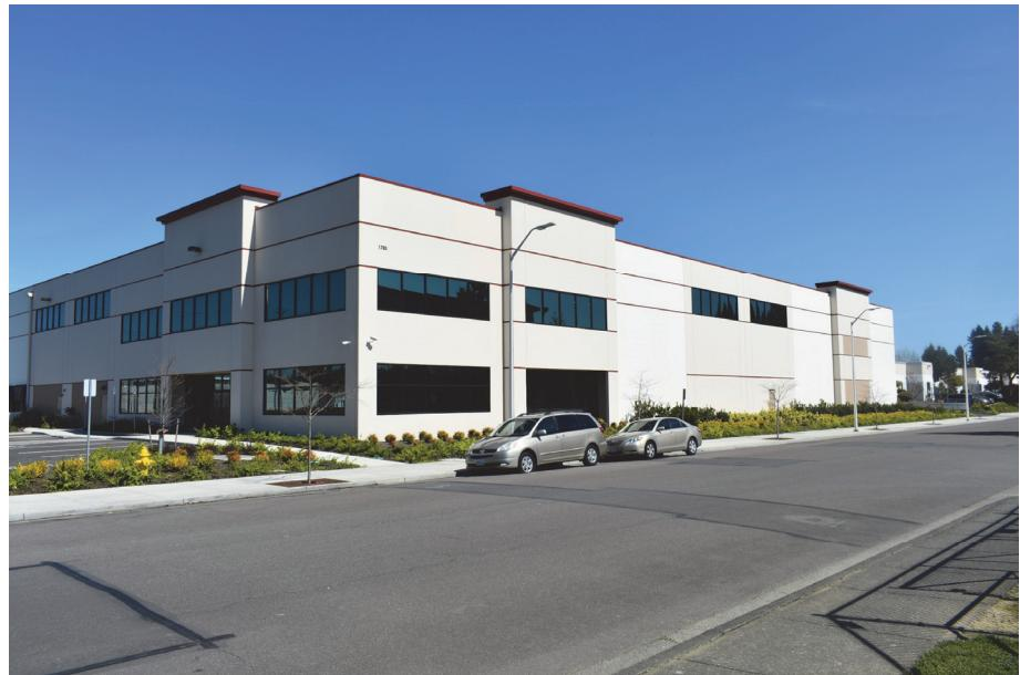
Figure 8-2      Example of a RWFD building with a small wall pop-out (photo credit: VLMK Engineering + Design).
