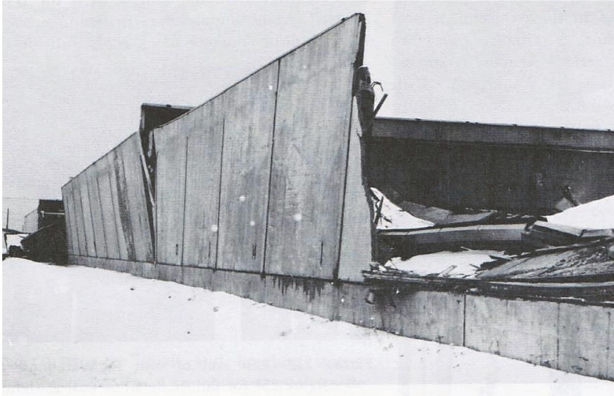
Figure 2-3 Collapse of a RWFD building at Elmendorf Air Force Base (photo credit: U.S. Air Force).
