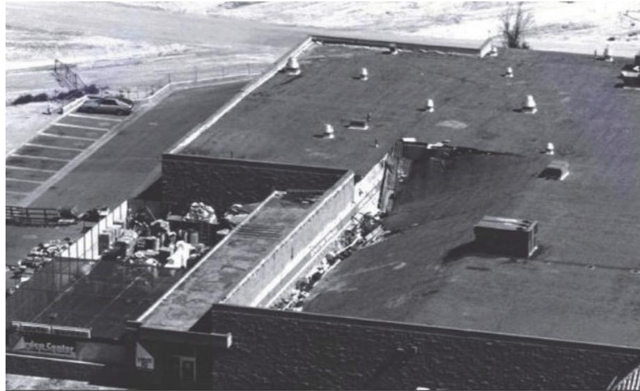
Figure 2-4 Partial collapse of a RWFD building with a steel deck diaphragm in Yucca Valley during the 1992 Landers Earthquake (photo credit: Gregg Brandow).
