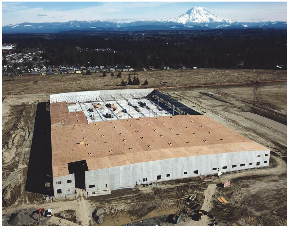
Figure 2-1      RWFD building with a wood structural panel diaphragm
