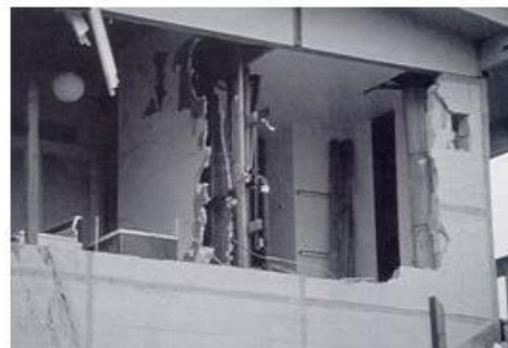
D) Collapse of masonry wall (HUD, 1993)
