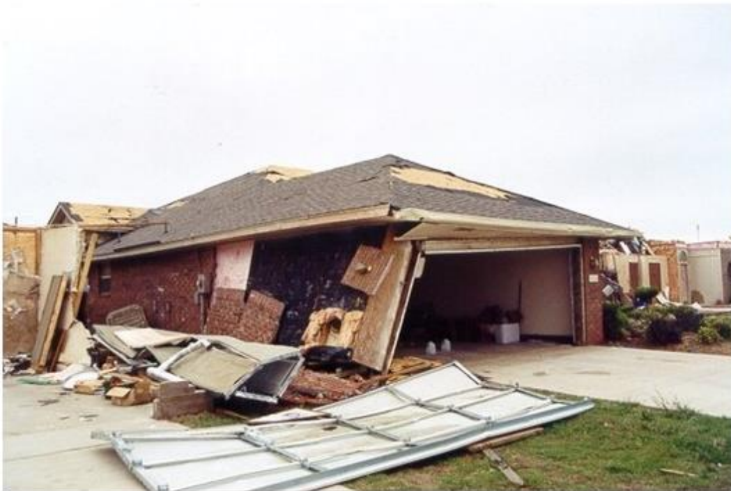
B) A wall section collapses
