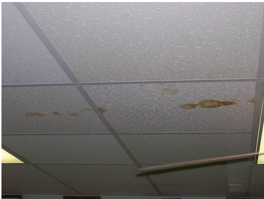
Figure 5-145 Water Damage to Interior Ceiling of a Fire Station in the Houston Area as a Result of Roof Damage (2008, Hurricane Ike)
