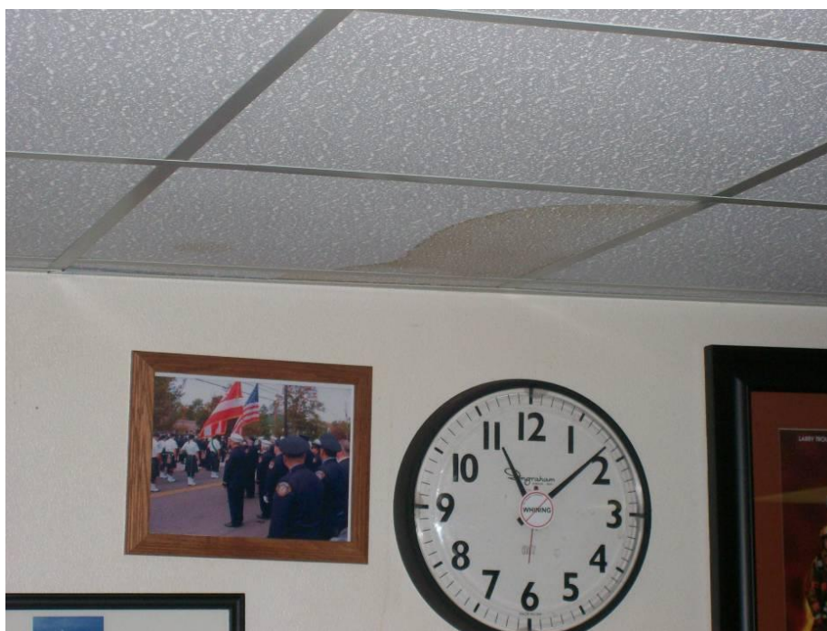
Figure 5-145 Water Damage to Interior Ceiling of a Fire Station in the Houston Area as a Result of Roof Damage (2008, Hurricane Ike)
