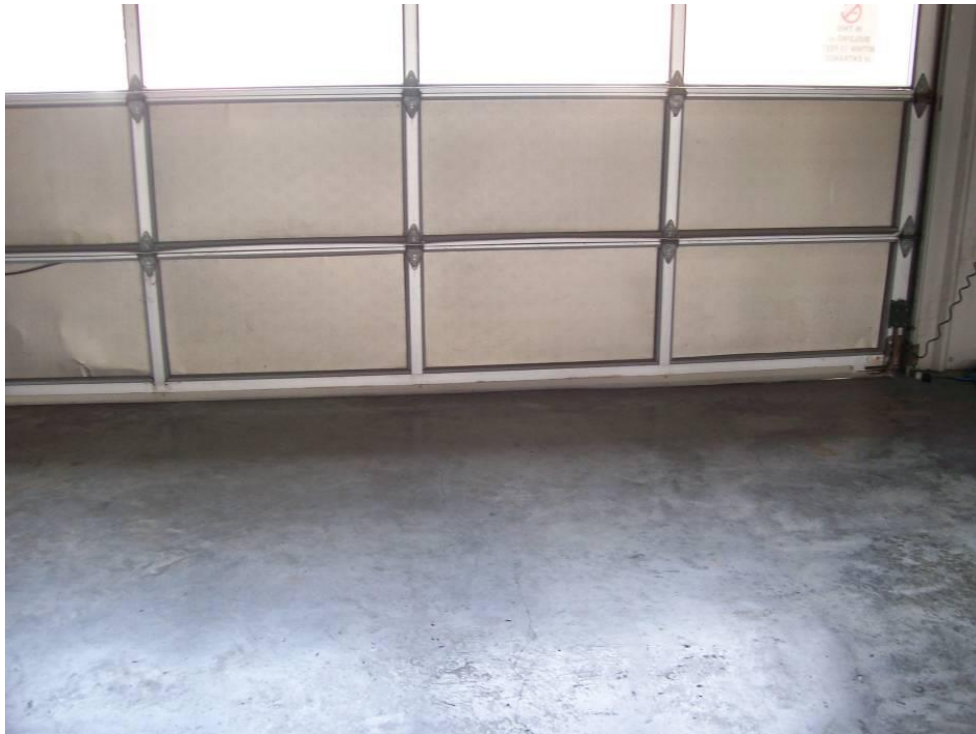
Figure 5-148 Panel Damage to Bay Doors for a Fire Station in the Houston Area (2008, Hurricane Ike)
