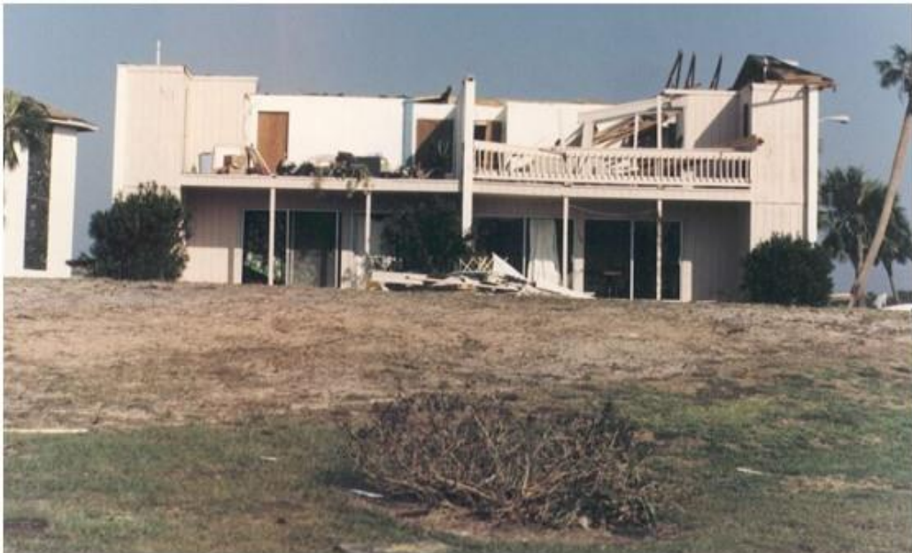
D) Whole Roof Failure, Wall Failure
