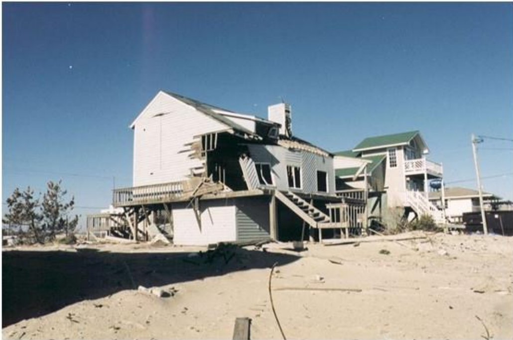
C) Wall Failure
