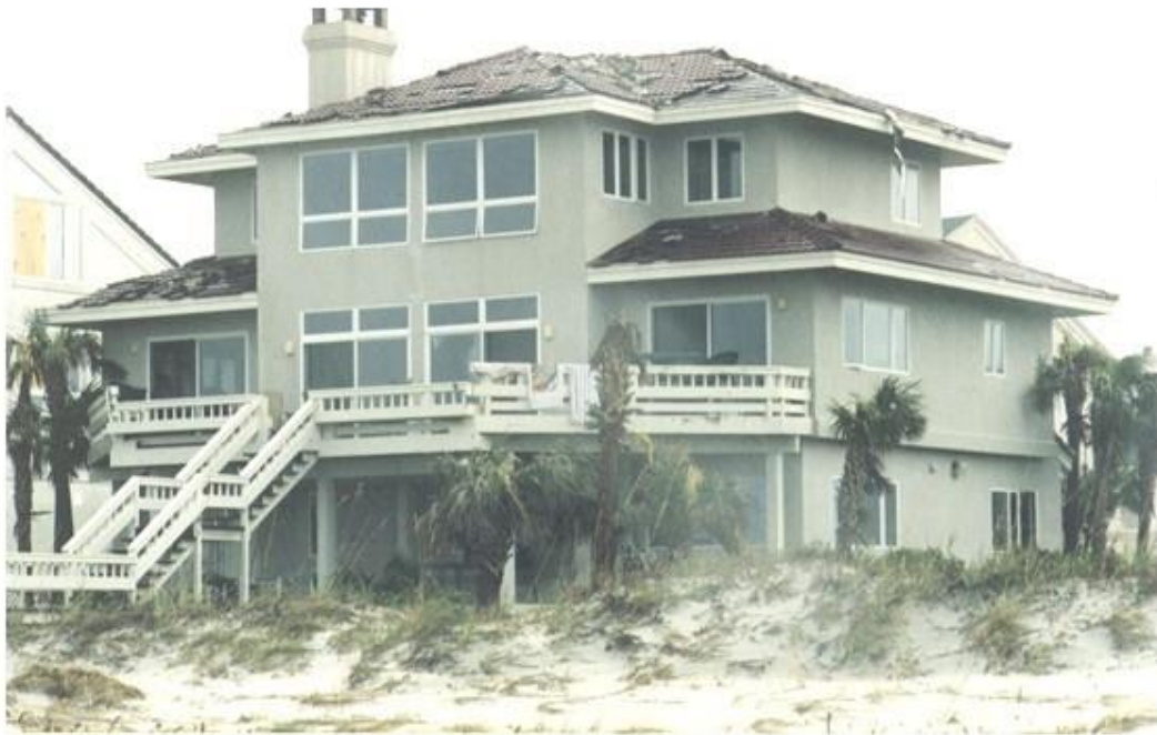
C) 2% to 15% Roof Cover Loss
