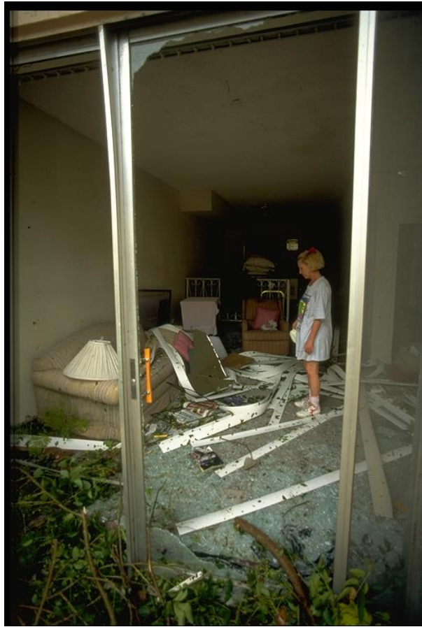
Figure 8-4 Content Losses Due to Fenestration Breach
