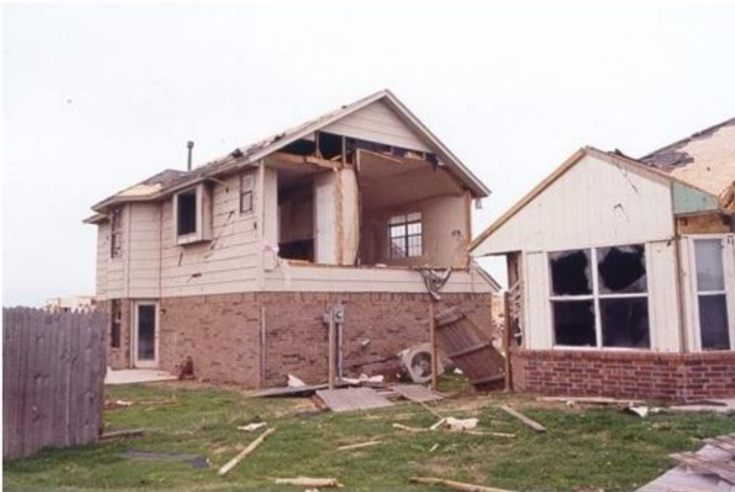
B) Wall failure at the other side of the same building shown in (a)
