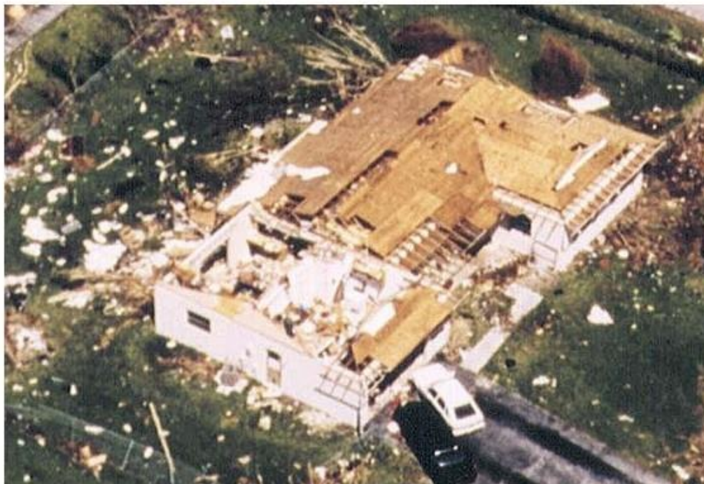
B) Complete Roof Failure, Greater than 25% Sheathing
