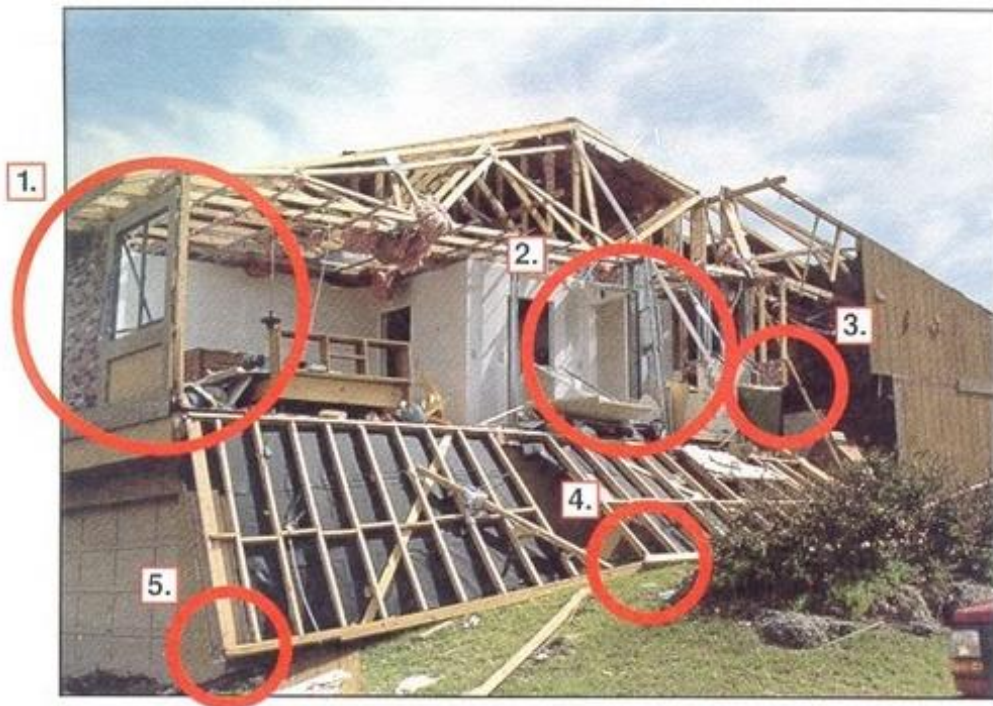
B) Several sections of a let-in braced wall collapse, failed at connections to gable end truss
