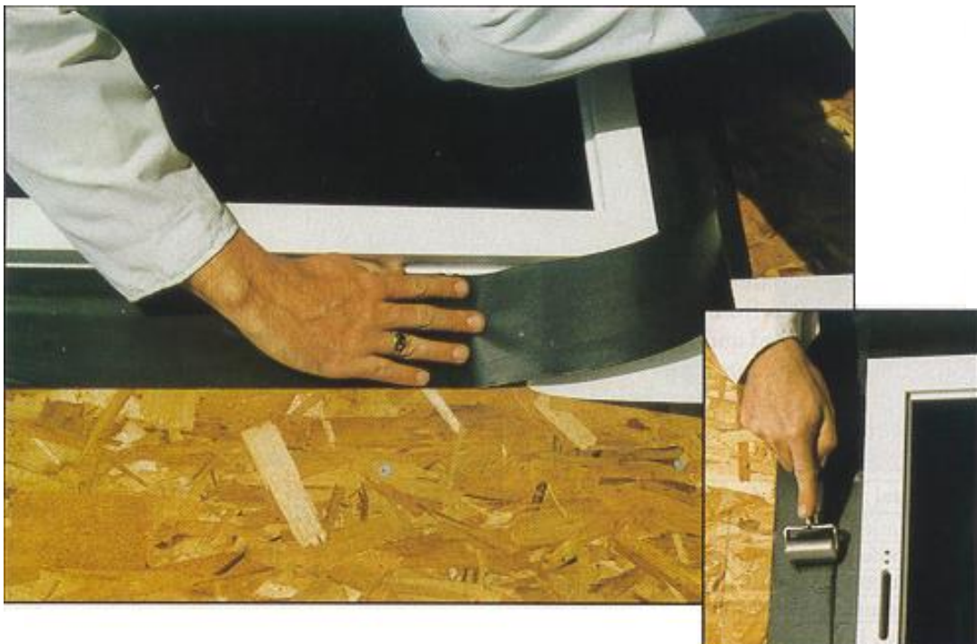
Figure 8-15 Example of Self-Adhering Waterproof Underlayment Used to Tape Plywood Joints, Ridges and Eaves; Photo Depicts Use Around Fenestrations
