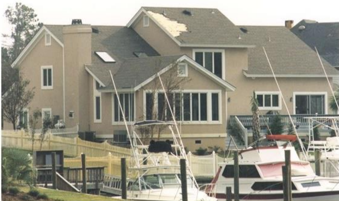
B) 2% to 15% Roof Cover Loss
