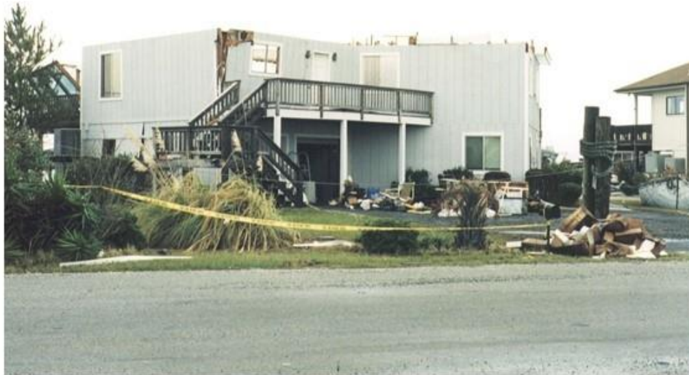
A) Complete Roof Failure
