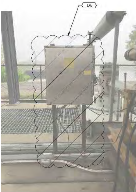
DEMOLITION PHOTO "D-02"
