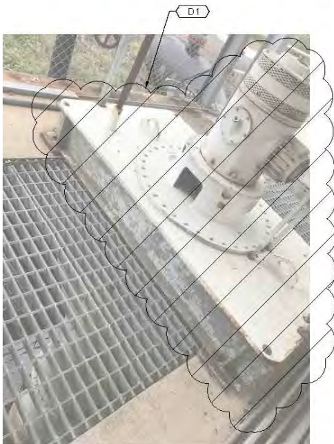
DEMOLITION PHOTO "D-01"
