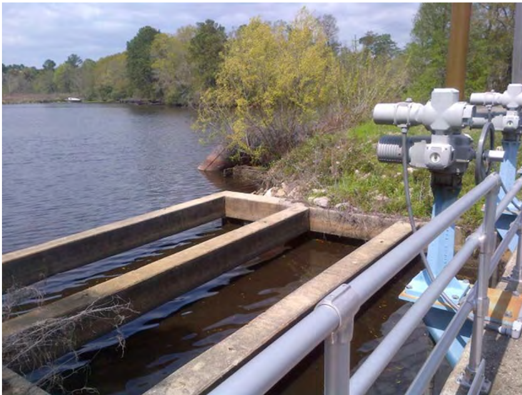
Looking west at Bayou Bonfouca while crossing the levee. Note the outfall pipe under the surface of the water.
