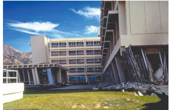
**Figure 2:** The recently opened Olive View Hospital was heavily damaged during the 1971 San Fernando earthquake. It was razed and rebuilt with a stronger, more seismic-resistant structure; see Figure 3. The San Fernando earthquake demonstrated deficiencies in the building code provisions of the time and was a motivating factor for the creation of NEHRP. Source: USGS (2003).
