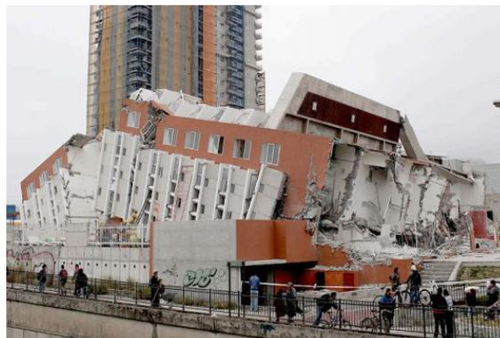
**Figure 5:** The Alto Rio 15-story apartment building in the city of Concepción, Chile, that collapsed during the 2010 Maule earthquake. Source: USGS (2011).
