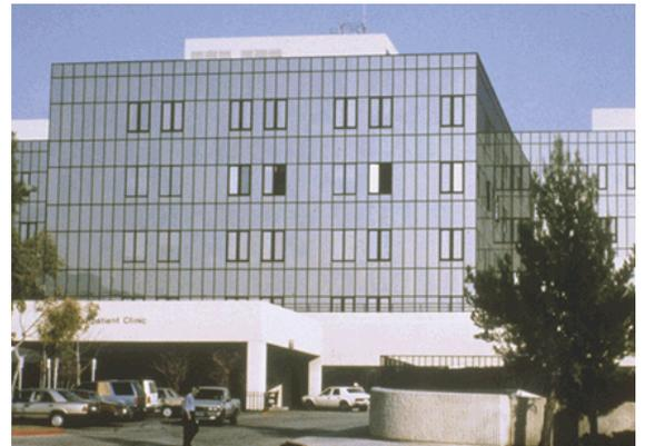
**Figure 3:** The new Olive View Hospital survived the 1994 Northridge earthquake with only minor structural damage. Source: USGS (2003).
