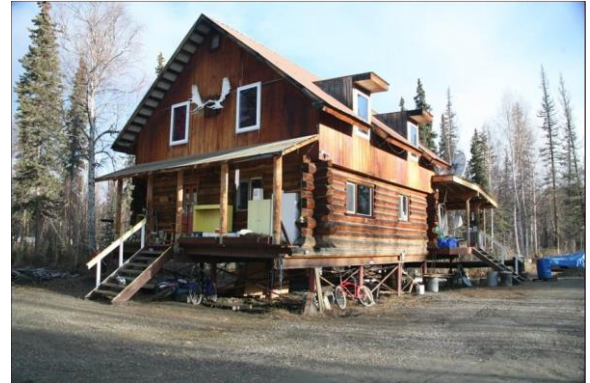
Figure 2. A home in Galena prior to elevation.
