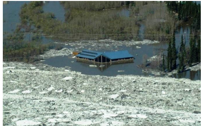
Figure 1. Flooding in Galena in 2013.
